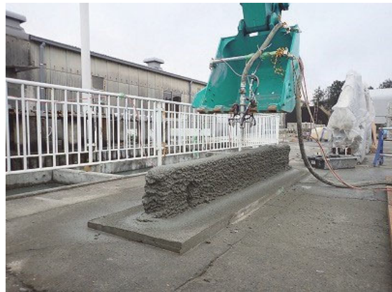
Rectangular wall constructed by downward spraying
