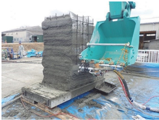
Wall constructed by sideways spraying
