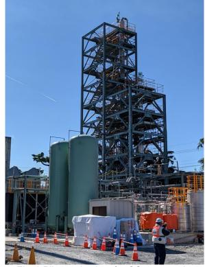
Fig. 3 Pilot-scale plant for CO<sub>2</sub> capture by chemical absorption
