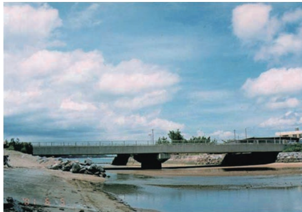
Fig. 7 Post-tensioned PC hollow-deck bridge
