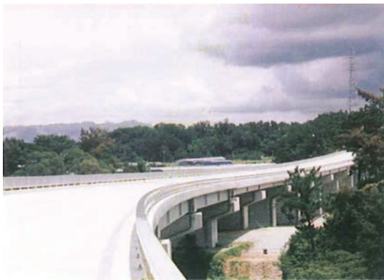
Fig. 5 Three span jointed pretensioned T-shaped girder bridge
