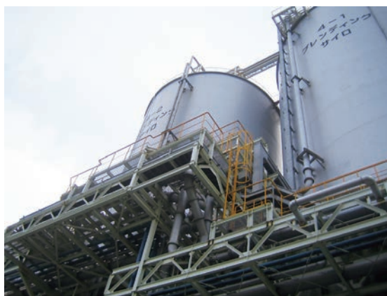
Fig. 3 Blending silo at power plant
