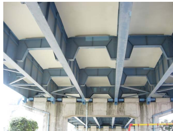
Fig. 2. Bottom-surface overlaying method
