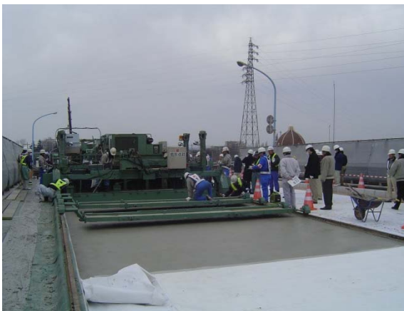
Fig. 1. Top-surface overlaying method
