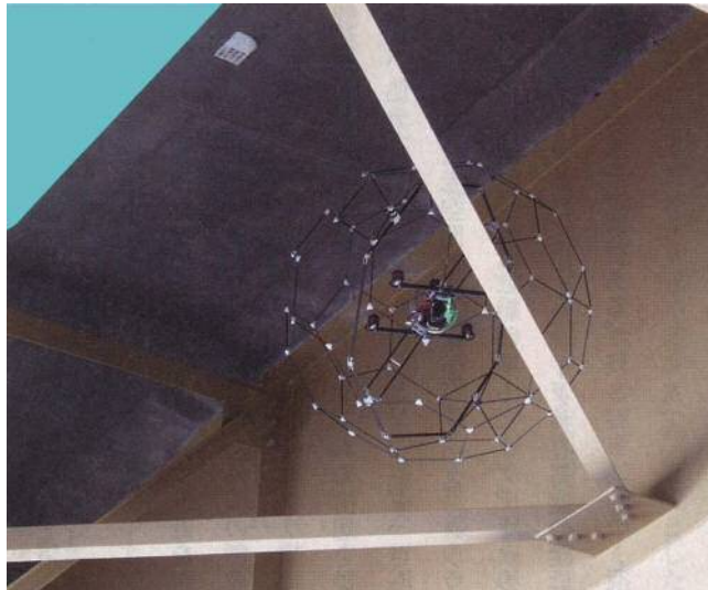
Photograph 1. A spherical multirotor craft inspecting a bridge.
