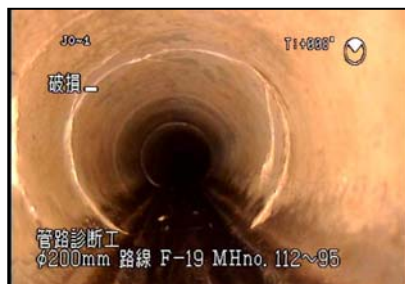
Crack (Concrete Pipe)
