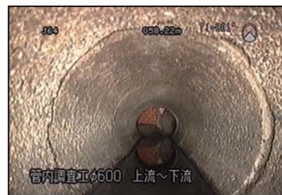
Corrosion (Concrete Pipe)
