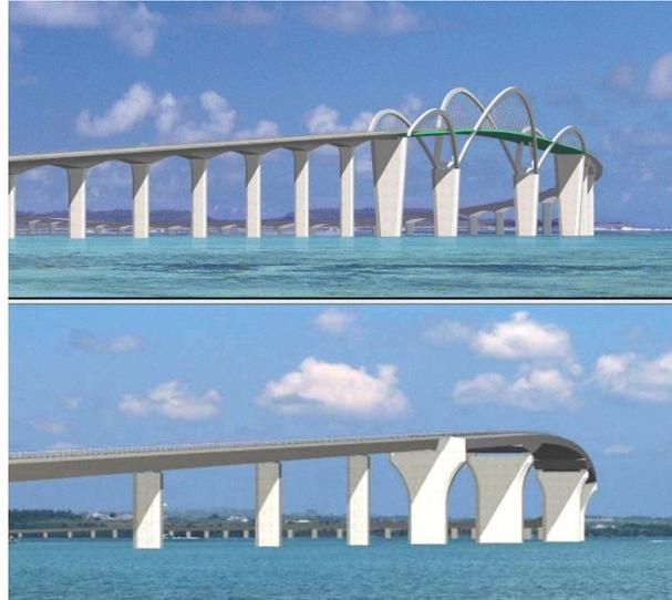
Figure 6. Top: The initial plan called for a three-span continuous half-through steel arch bridge. Bottom: The final plan called for a three-span continuous steel floor-slab box-girder bridge.
