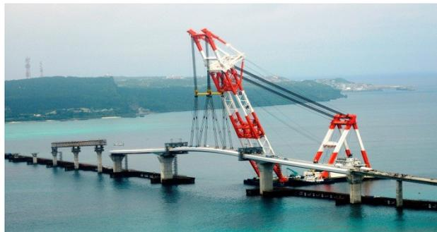
Photo 8. Simultaneous erection of large blocks
