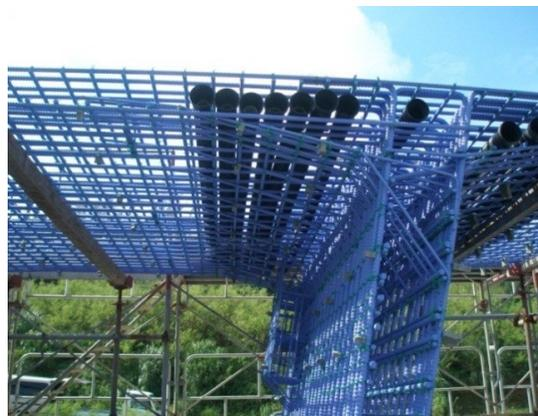
Photo 3. Salt damage protection measures for superstructure (coated reinforcing steel and polyethylene sheath)
