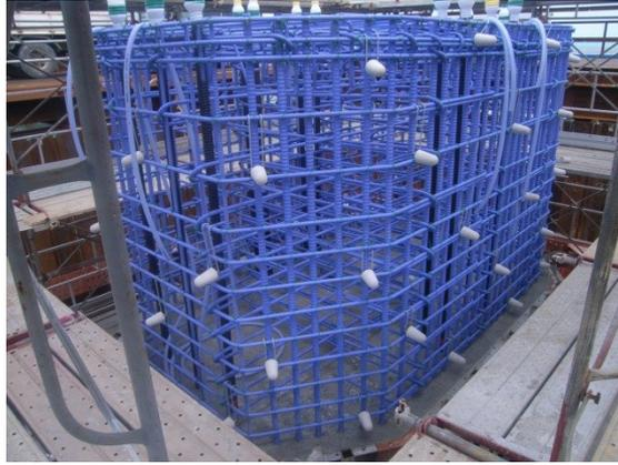
Photo 2. Erection of coated reinforcement steel for substructure
