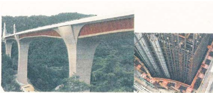
図-7 高橋脚と過密配筋 Fig. 7 High pier of bridge and confined zone of reinforcing bars
