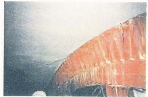
図-8 トンネルアーチクラウン部に確実に充填 Fig. 8 Self-compacting concrete for reliable placement into archcrown of tunnel
