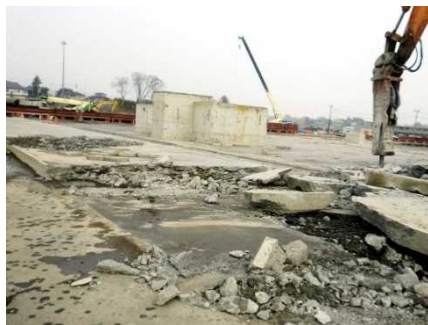
Demolition of cement-hardened material
