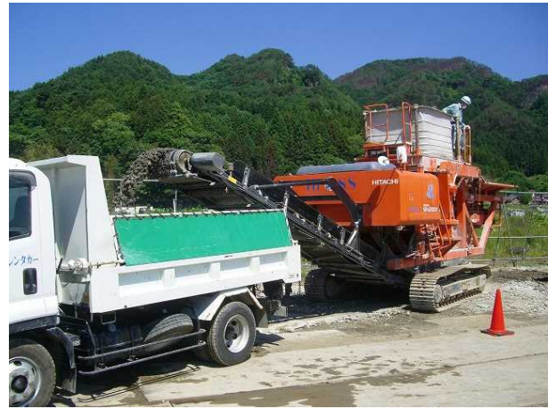
Photo 2. Mixing with cement and water
