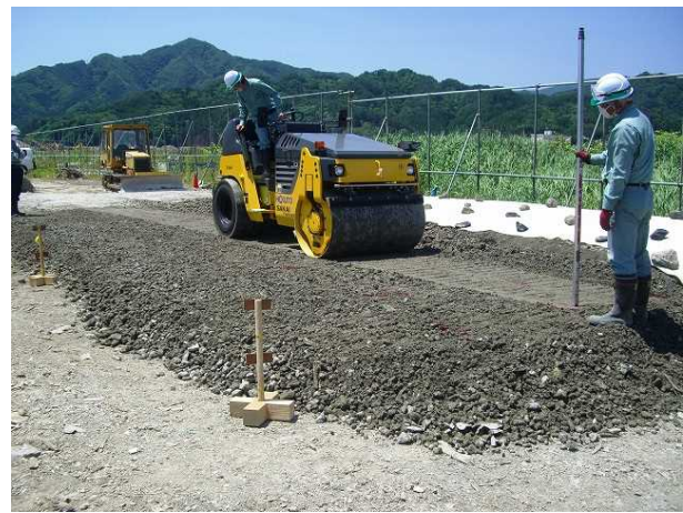
Photo 4. Compacting with a vibrating roller
