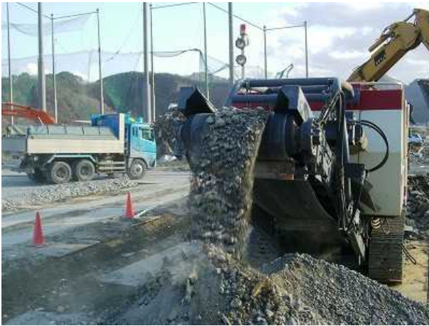
Photo 1. Crushing concrete rubble
