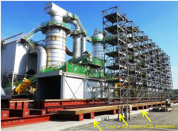
Photo 5. Location where cement-hardened material was placed
