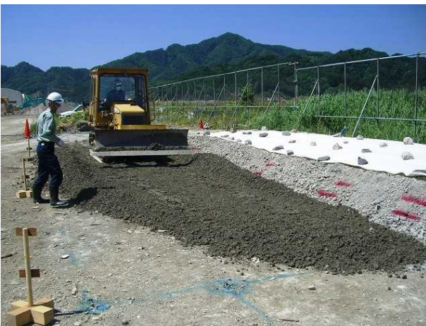
Photo 3. Leveling with a bulldozer
