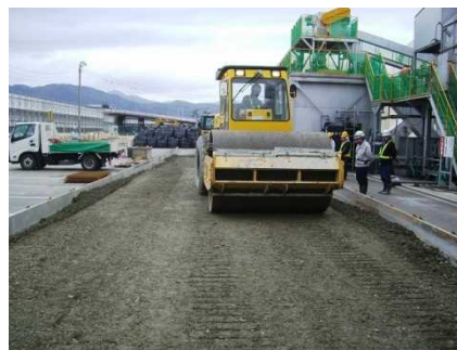
Placement with rolling compaction
