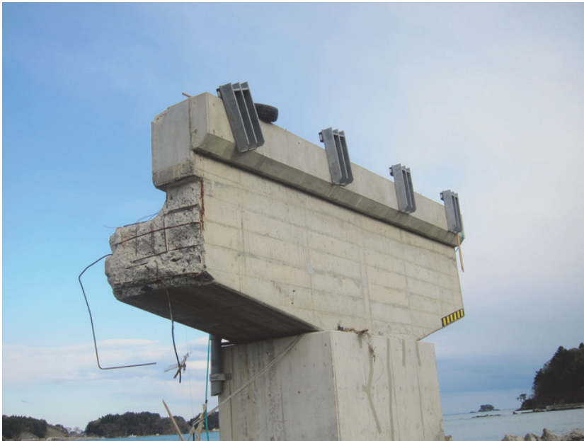
Figure 7 Stoppers on the Utsu-Ohashi bridge
