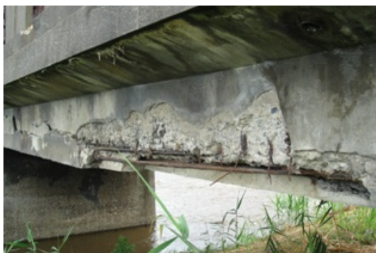
Fig.1 Reinforcement corrosion
