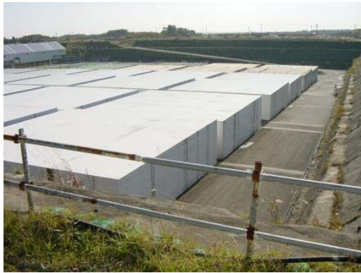
Huge concrete structures for storage of nuclear waste in Aomori, Japan
