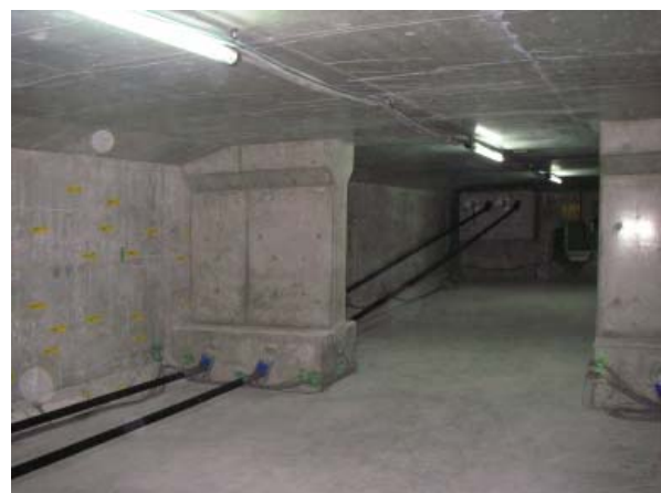
Crack repairs and strengthening by out-cables
