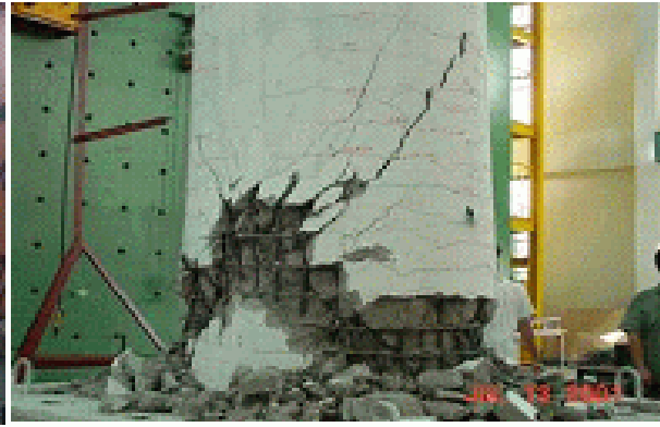
Figure 13. Failure of MD-HT6-N-L2
