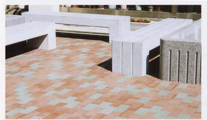
Interlocking blocks at Hitachi Seaside National Park
