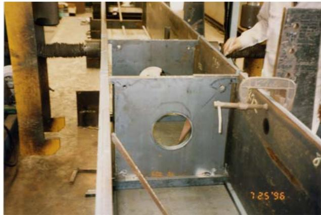
Fig. 23 Diaphragms in a steel tubular column
