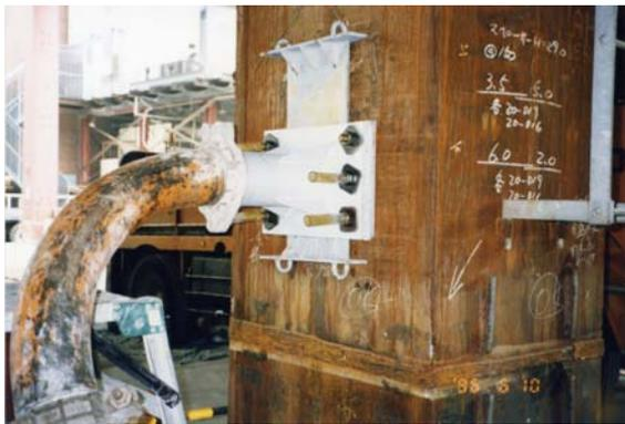
Fig. 24 Placing with a concrete pump
