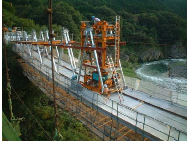
Fig.4-2 Erection of truss chords
