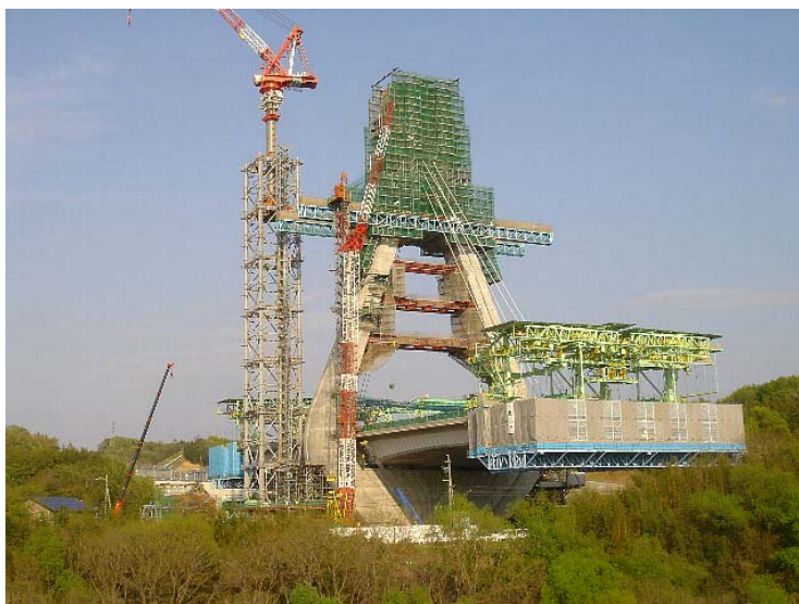
Photo 2-3 Free cantilever erection with the traveler
