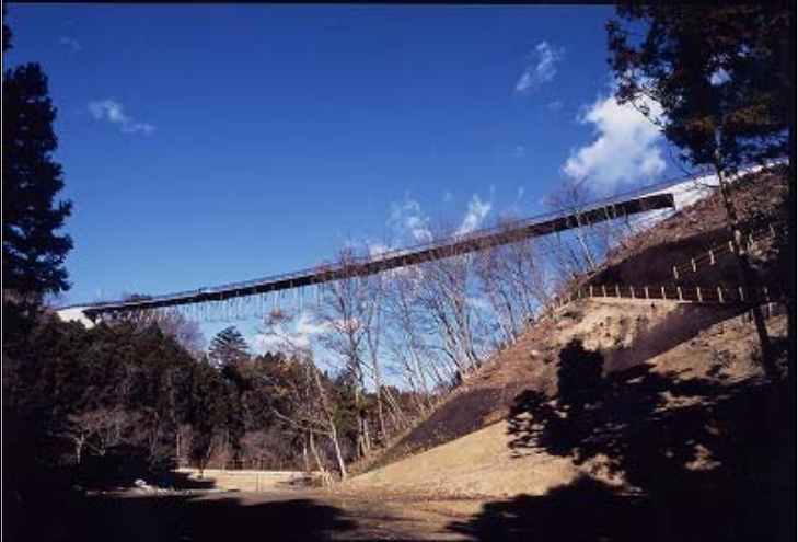
Photo 5-1 Completed MORINO-WAKUWAKU Bridge
