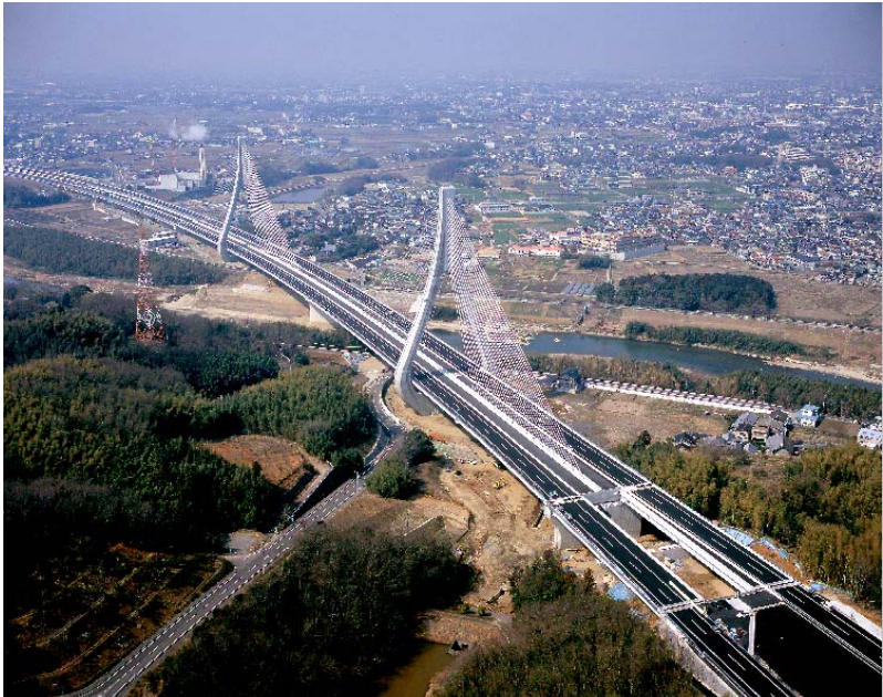
Photo 2-1 the completed YAHAGI-GAWA Bridge
