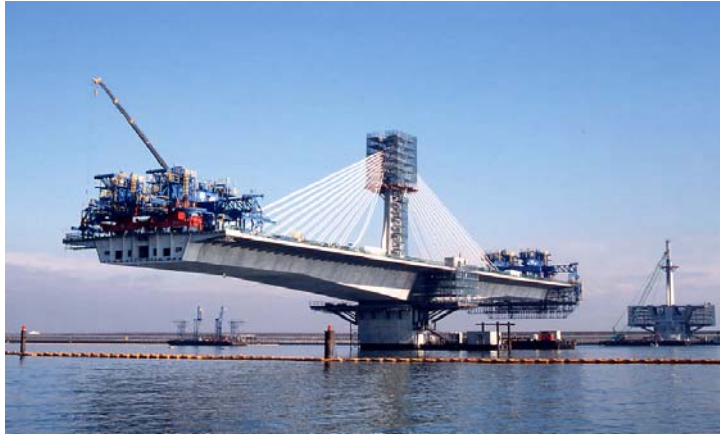
Photo 1-2 After the completion of concrete
