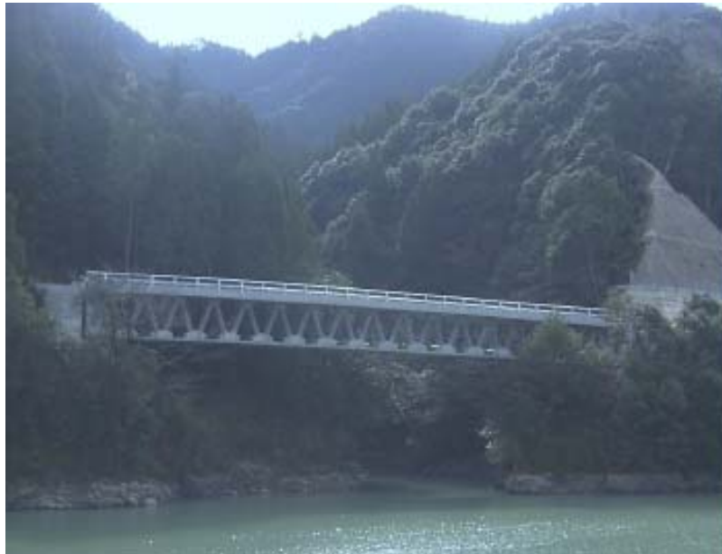
Photo 6-1 Completed KAMAN-TANI Bridge
