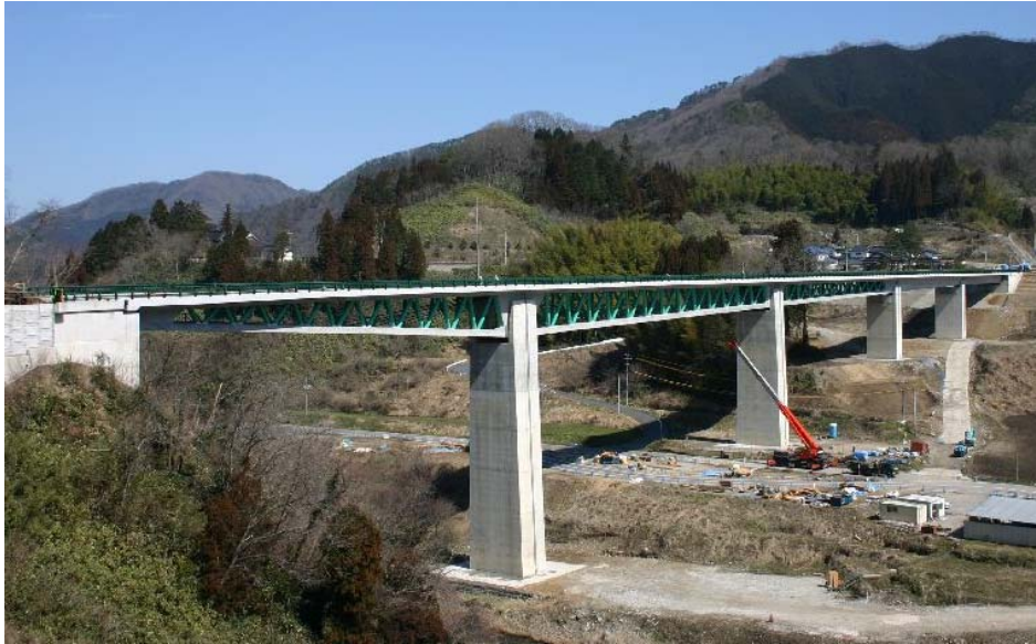
Photo 3-1 the completed bridge SHITSUMI-OHASHU Bridge
