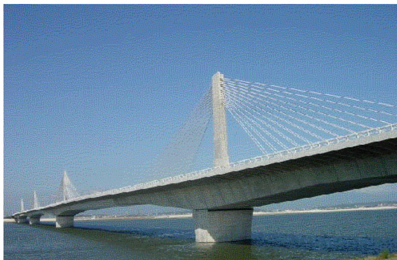
Photo 1-1 Completed KISO River Bridge
