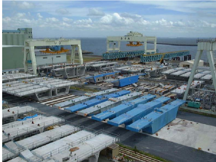
Photo 1-5 Prefabrication casting yard
