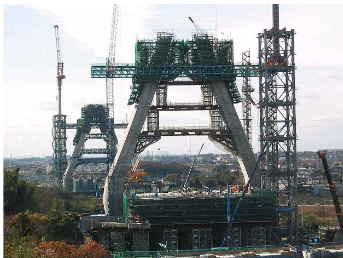
Photo 2-2 Climbing scaffolding for the pylon
