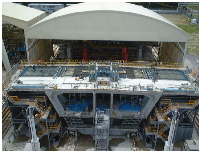
Photo 1-4 Short-line-match-casting
