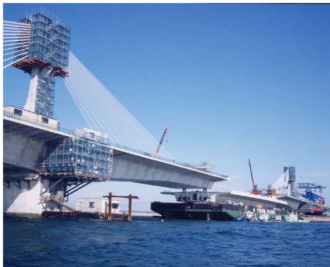
Photo 1-3 Erection of the central steel girder
