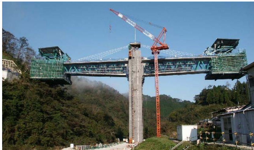
Photo 3-3 the bridge under erection
