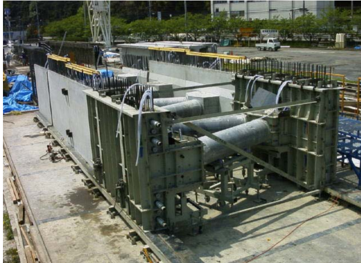
Photo 6-2 Segment fabrication
