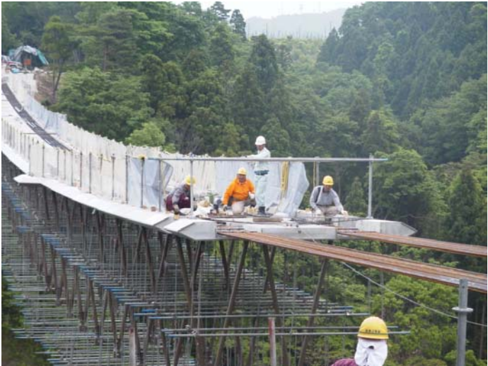
Photo 5-2 Sliding erection
