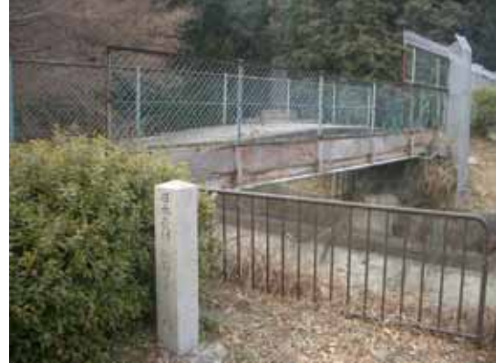
Fences have been installed to prevent passersby from falling.
