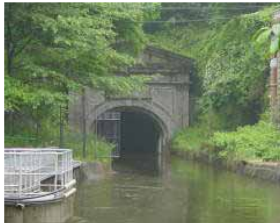
Hinooka, the third water tunnel outlet
