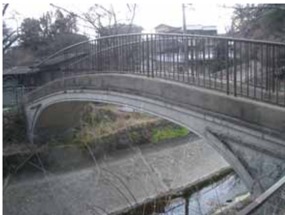
The fences were installed later
