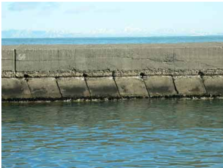
Close-up View of Breakwater
