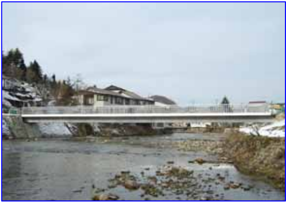
Akakura Onsen Yukemuri Bridge (Span: 35m)
