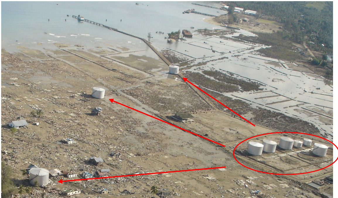
Photo 9.2 Displaced oil tanks by the tsunami
