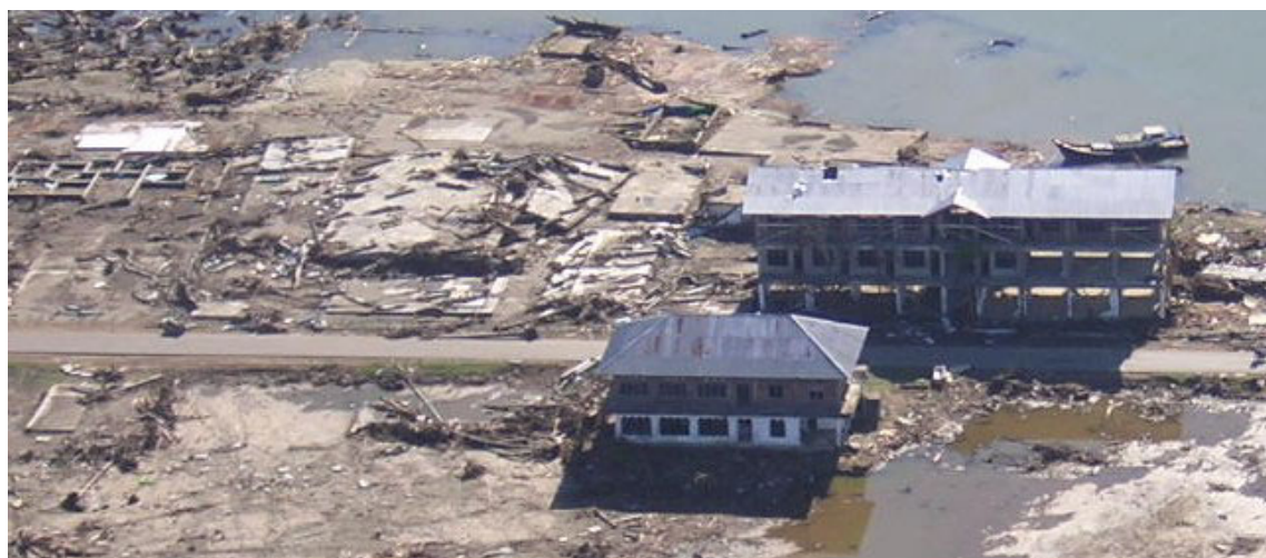
Photo 7.4 Damage to RC buildings in tsunami-affected area
