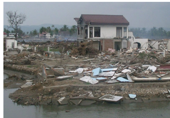
Photo 7.2 Damage to masonry (brick) buildings
