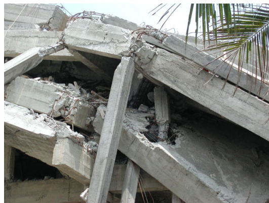
Photo 7.3(b) Collapsed or heavily damaged RC buildings
