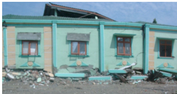
Photo 7.3(a) Collapsed or heavily damaged RC buildings
