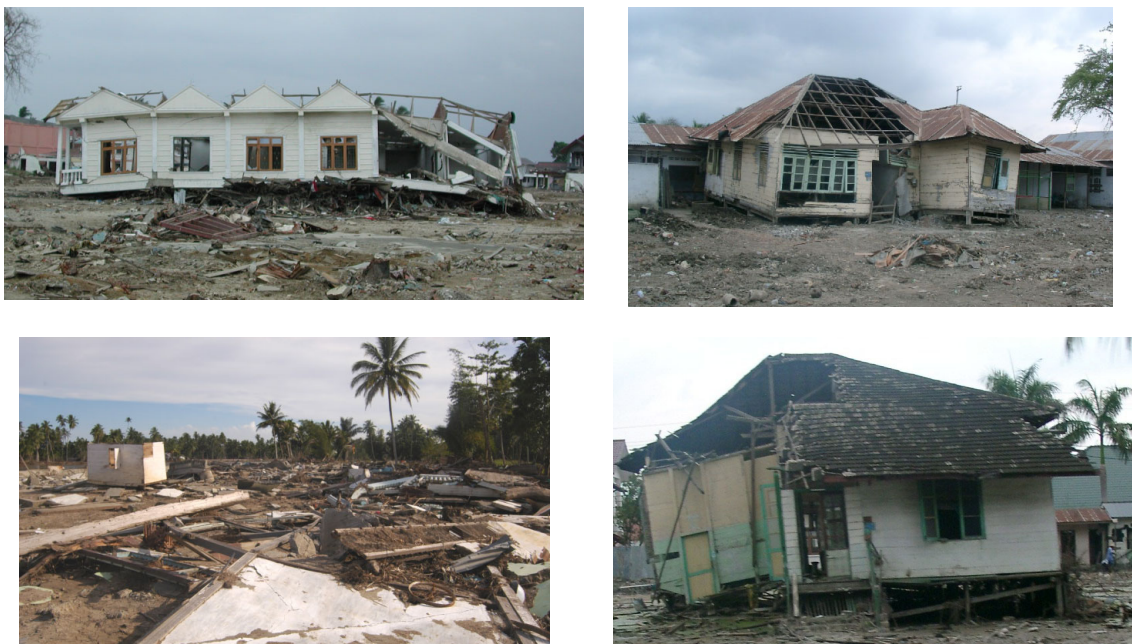
Photo 7.1 Damage to wooden houses
