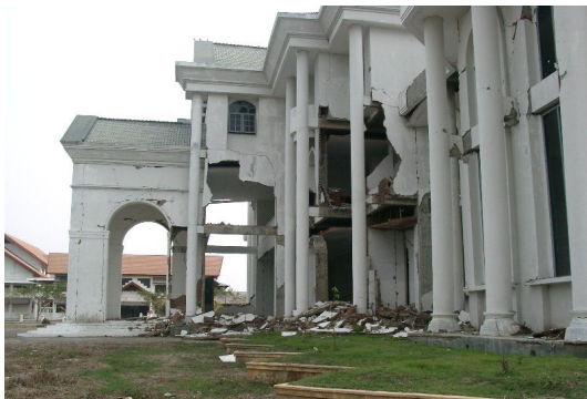
Photo 7.3(a) Collapsed or heavily damaged RC buildings
