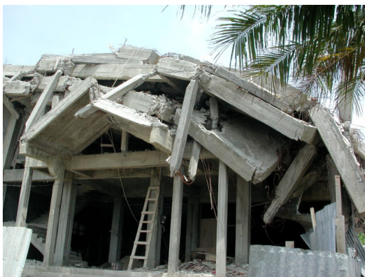
Photo 7.3(b) Collapsed or heavily damaged RC buildings
