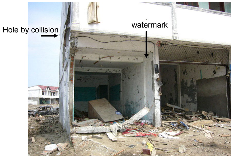
Photo 5.4 A hole by collision of an obstacle and watermark
