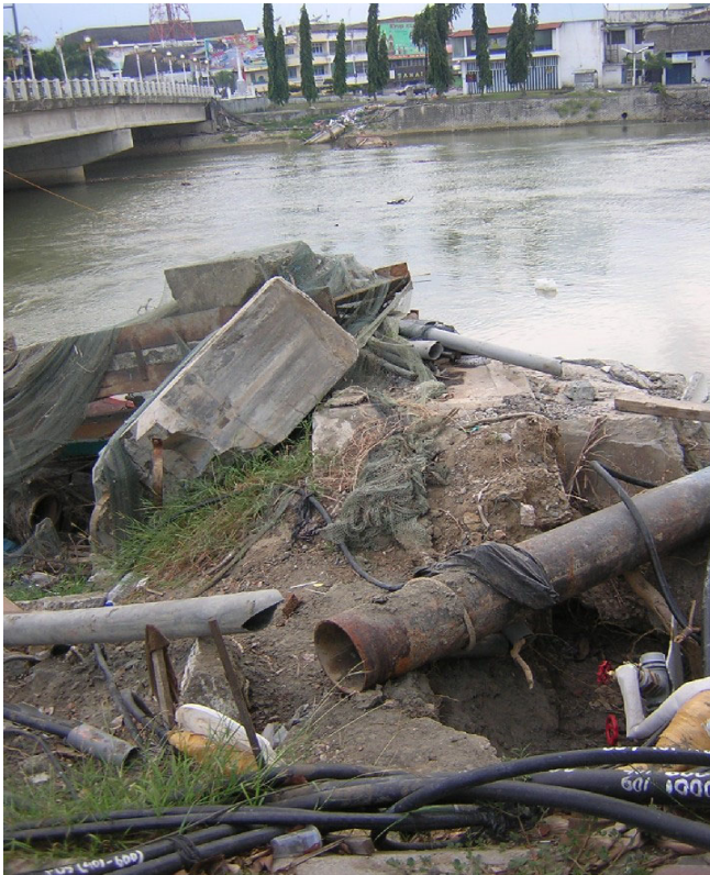
Photo 12.4 Broken water pipes nearby or attached to bridges
