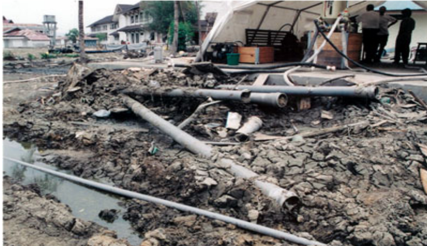
Photo 12.7 Scattered transmission pipe around pump station
