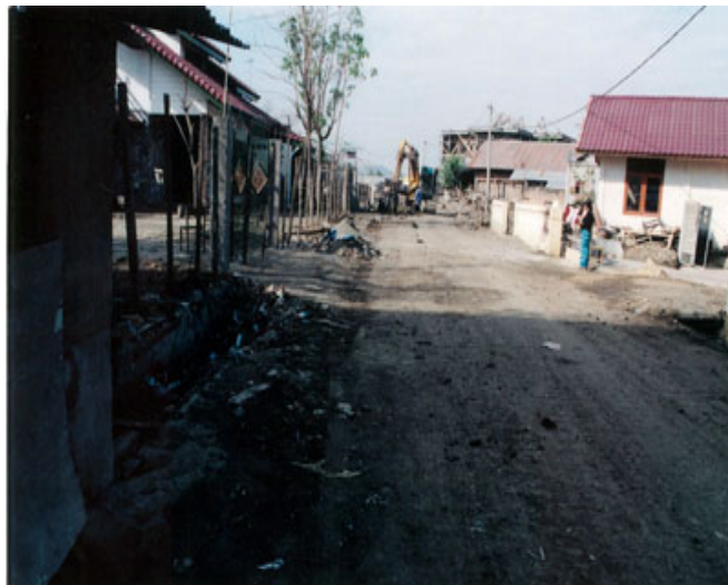
Photo 12.6 Drain ditches are clogged with mud and debris. Backhoe is operating for removal of deposit of the flood.
