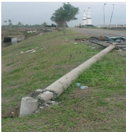
Photo 12.9 Broken electric distribution poles
