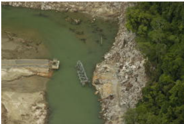
Photo 11.26 Washout of Truss Bridge (3) (courtesy of Aceh Provincial Government)
