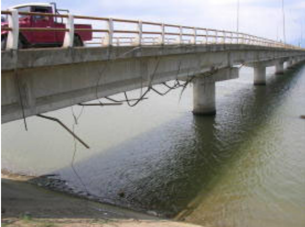
Photo 11.11 Undamaged Bridge by Tsunami
