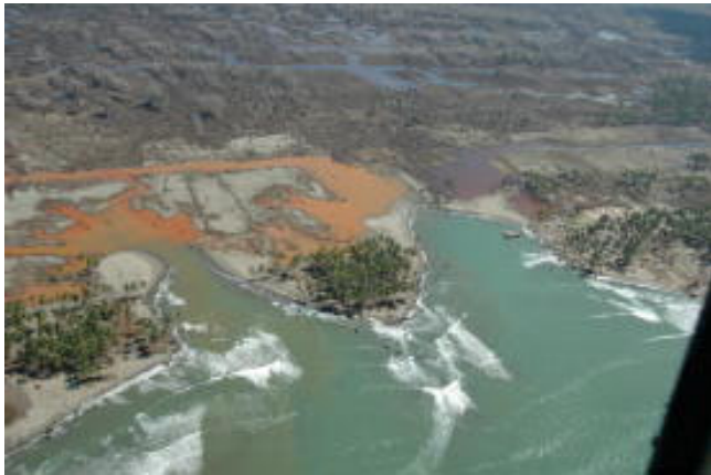
Photo 11.29 Erosion of Road and Coastline (courtesy of Aceh Provincial Government)
