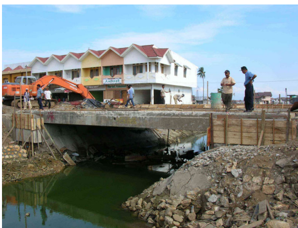
Photo 11.1 Repair of Washed-out Girder Bridge
