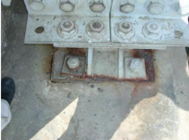
Photo 11.16 Steel Bearing Supports
