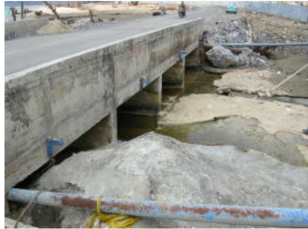
Photo 11.23 Concrete Box Culvert Bridge
