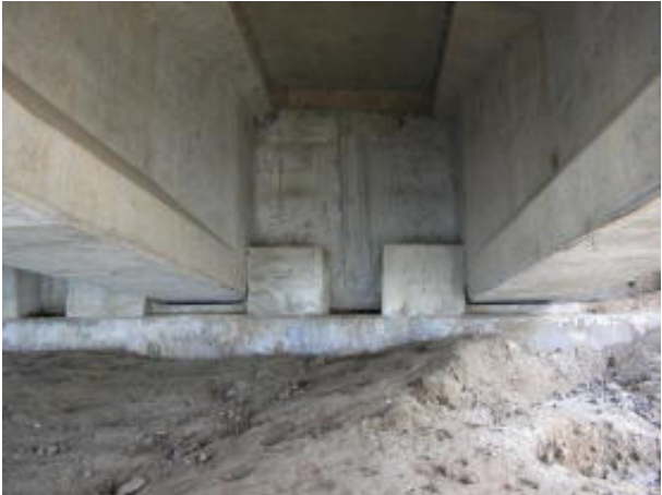
Photo 11.12 Concrete Block Shear Keys
