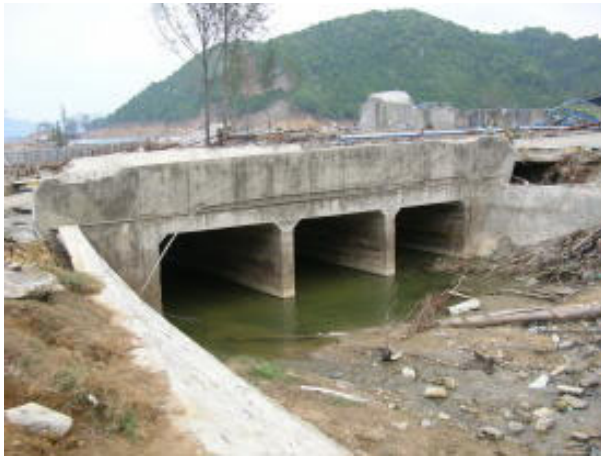
Photo 11.22 Concrete Box Culvert Bridge
