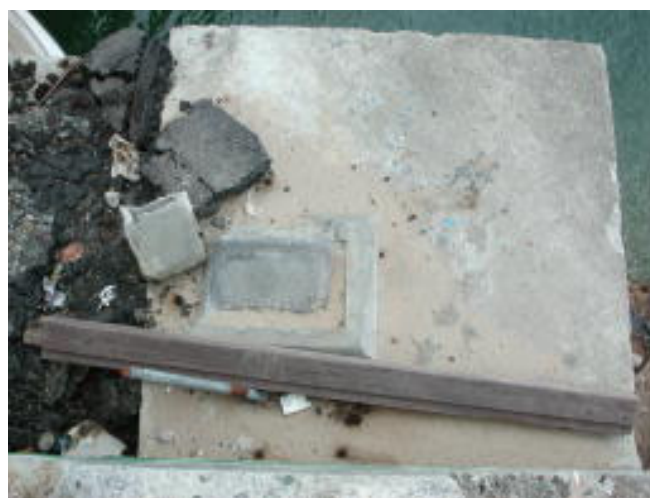
Photo 11.21 Bearing Support and Bolt to connecting Deck and Substructures
