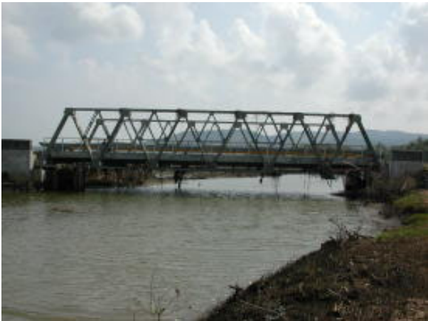
Photo 11.15 Steel Truss Bridge without Damage
