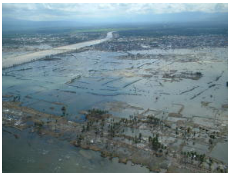
Photo 11.31 Erosion of Road and Coastline (courtesy of Aceh Provincial Government)
