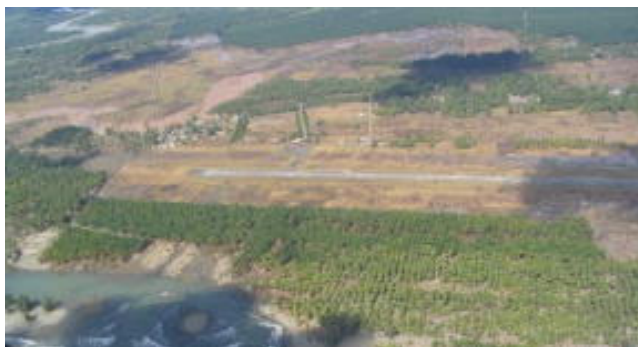
Photo 11.33 Damage of Airstrip at Meulaboh Airport
