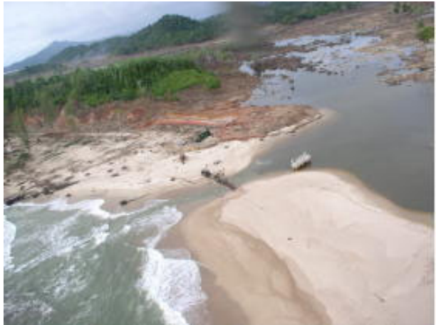
Photo 11.30 Erosion of Road and Coastline (courtesy of Aceh Provincial Government)
