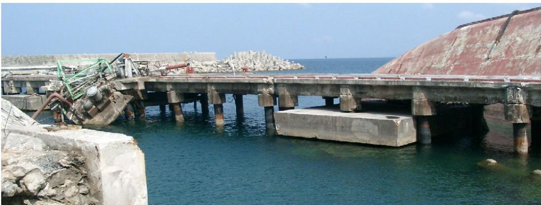
Photo.10.7 Damaged pile-supported wharf at cement factory
