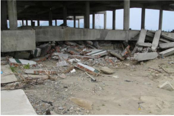
Photo 10.4 Ferry terminal (collapsed ground floor)
