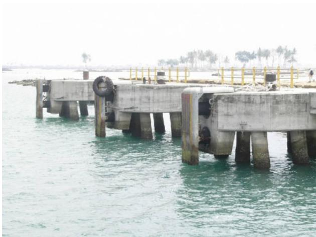
Photo 10.2 Dolphin for a power generator barge
