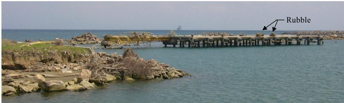
Photo 10.1 Pile supported wharf for ferry boat
