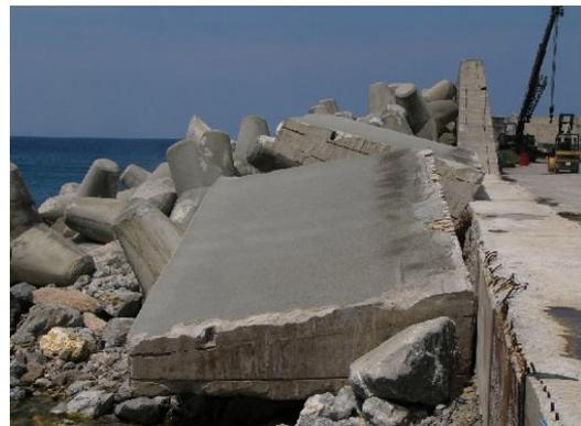
Photo 10.6 Damaged seawall at cement factory
