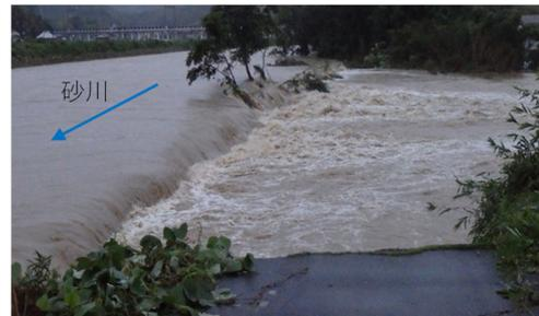
図-11 砂川左岸決壊状況(図-2赤枠②地点)<sup>2)</sup>
