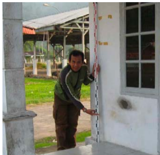
Fig.6.8 Measuring tsunami height of water marks on the wall above the ground
