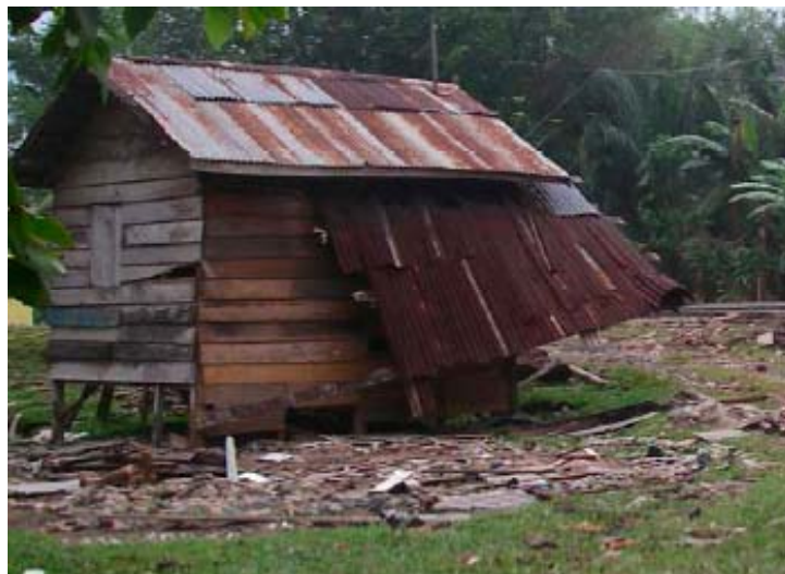
Fig.6.13 The house damaged and moved by the tsunami
