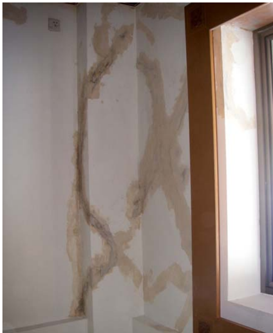
Fig.5.5 Re-Plastered columns of an RC building used as an hotel in Padang
