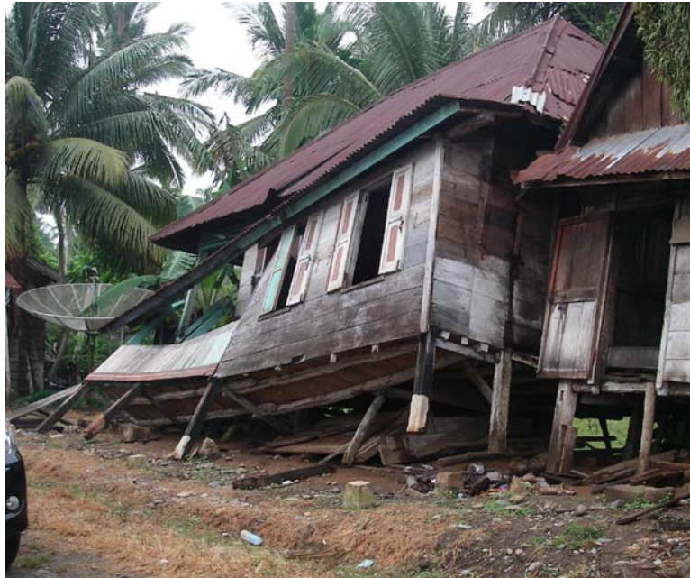
Fig.5.3 Total collapse of a wooden house in Pasir Banting due to embankment failure
