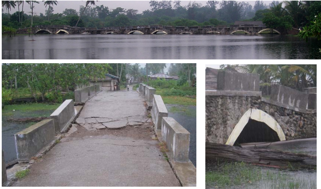
Fig.5.9 Damage to the arch bridge at Pasir Ganting due to ground liquefaction
