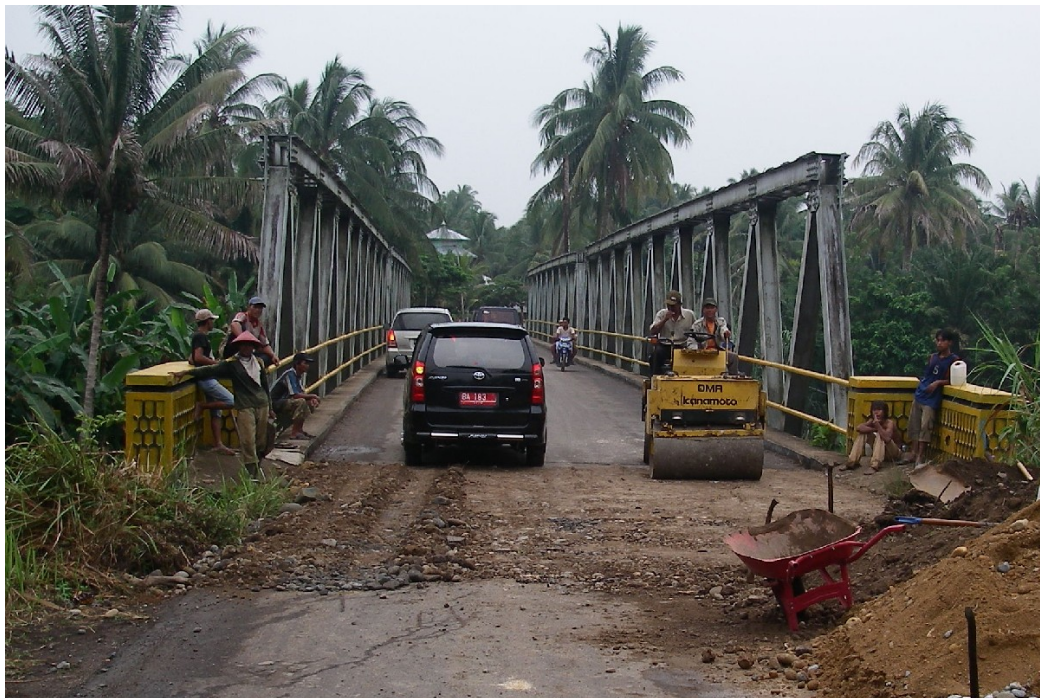
Fig.5.11 Damage to approach embankments of bridges
