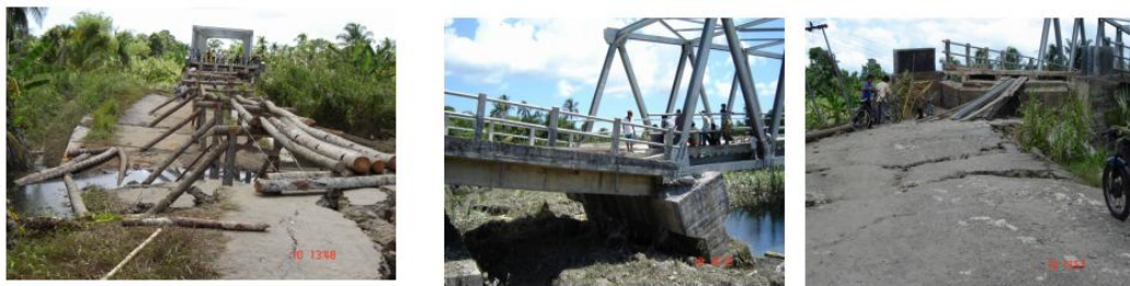
Fig.8.3 Liquefaction induced damage to Muzoi River bridge by 2005 Nias earthquake
