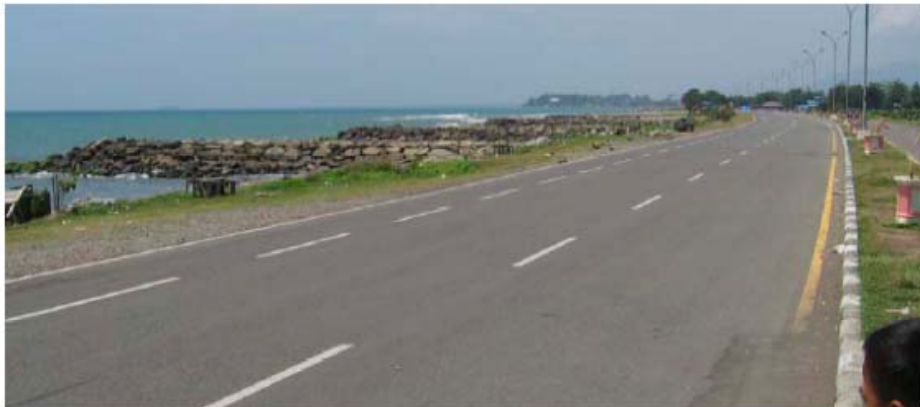
Fig.8.5 Sea dike with the height of 2-3 m at Padang, which prevent a small tsunami and stop the inundation.
