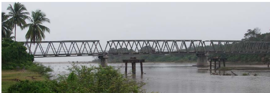
Fig.5.10 Slight damage to Seblat River Bridge due to uneven settlements
