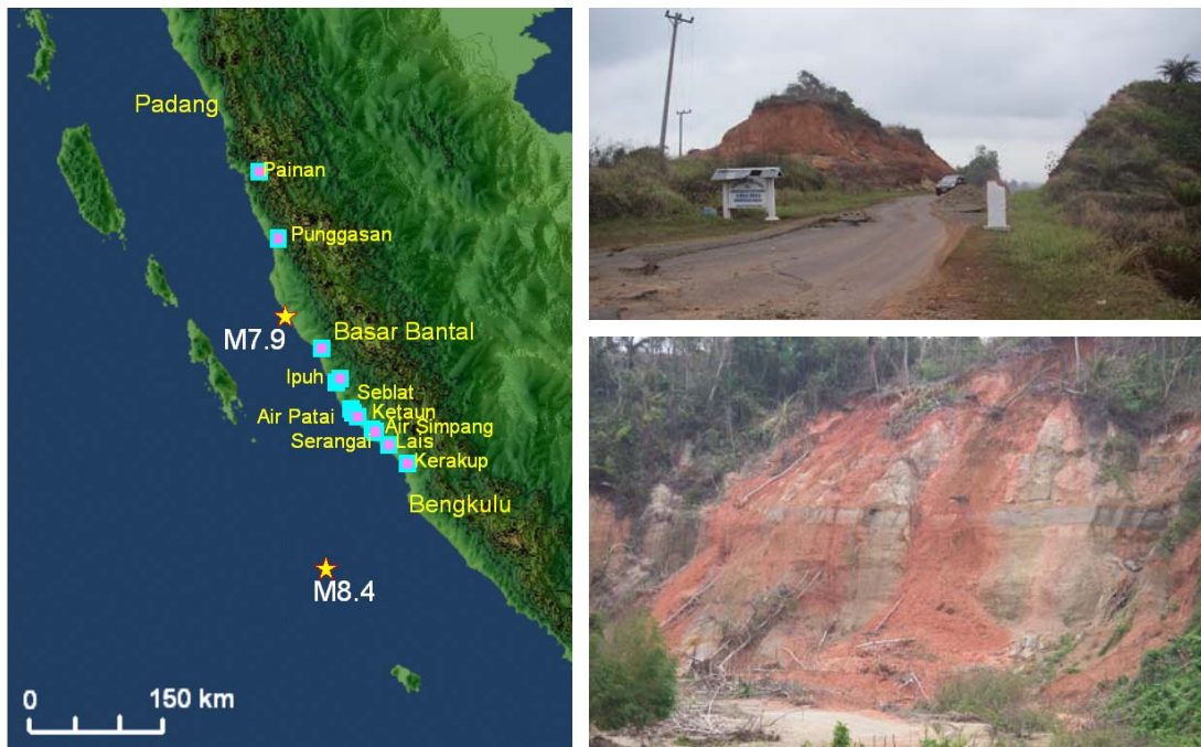
(a) Locations of observed slope failures (b) views of some slope failures
