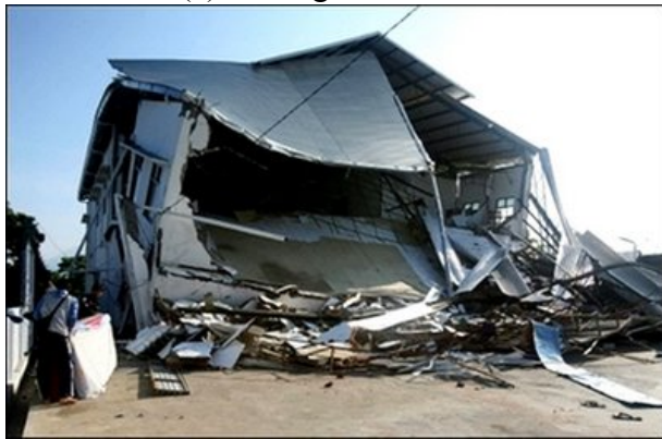
(c) Collapsed show room in Argamakmur
