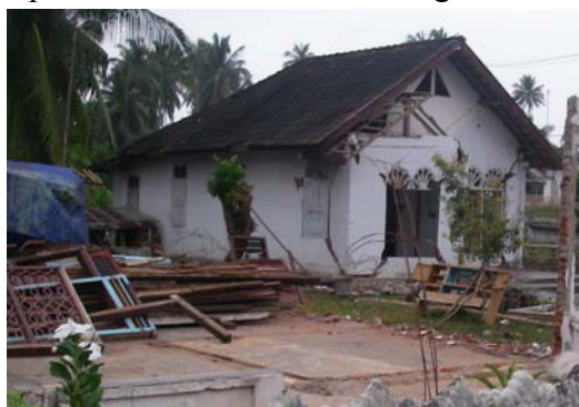
Fig.5.2 Collapsed or heavily damaged brick masonry houses
