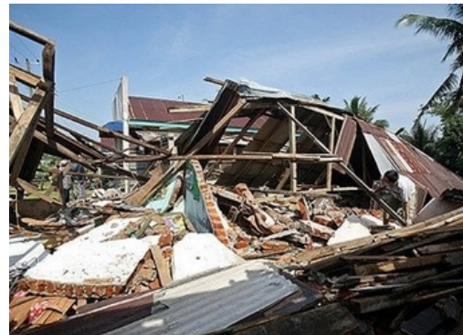
Fig.5.2 Collapsed or heavily damaged brick masonry houses
