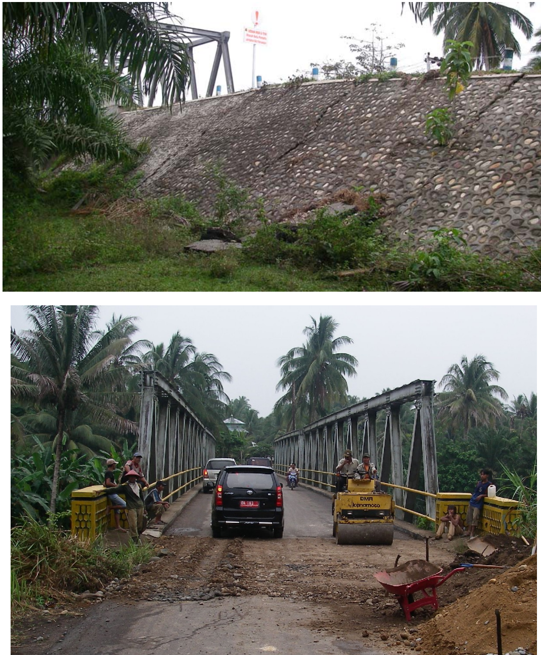
Fig.5.11 Damage to approach embankments of bridges
