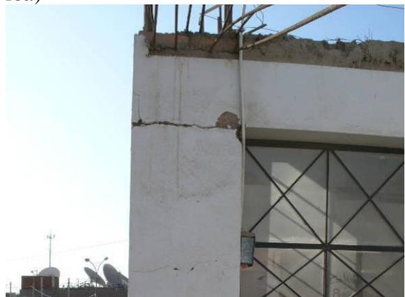
*Fig. 4.37 Weak cold joint between column and beam/slab (Parcona, Ica)*
