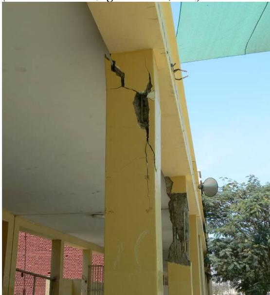
Fig. 4.50 Lack of shear reinforcement in columns (San Luis Gonzaga School, Ica)
