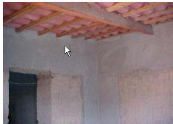
Step 4. Moisten the area and plaster it with cement sand mortar applied in two layers.
