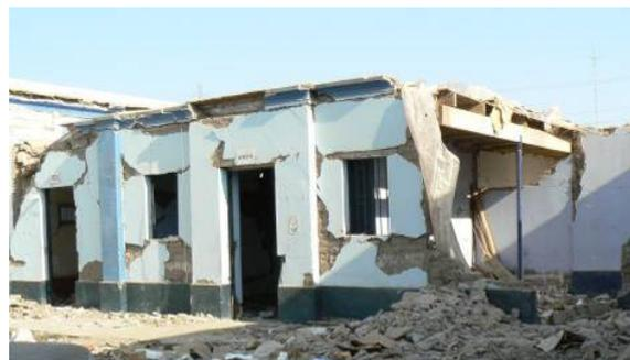
Fig. 4.41 A hospital building made of non-reinforced adobe was heavily damaged
