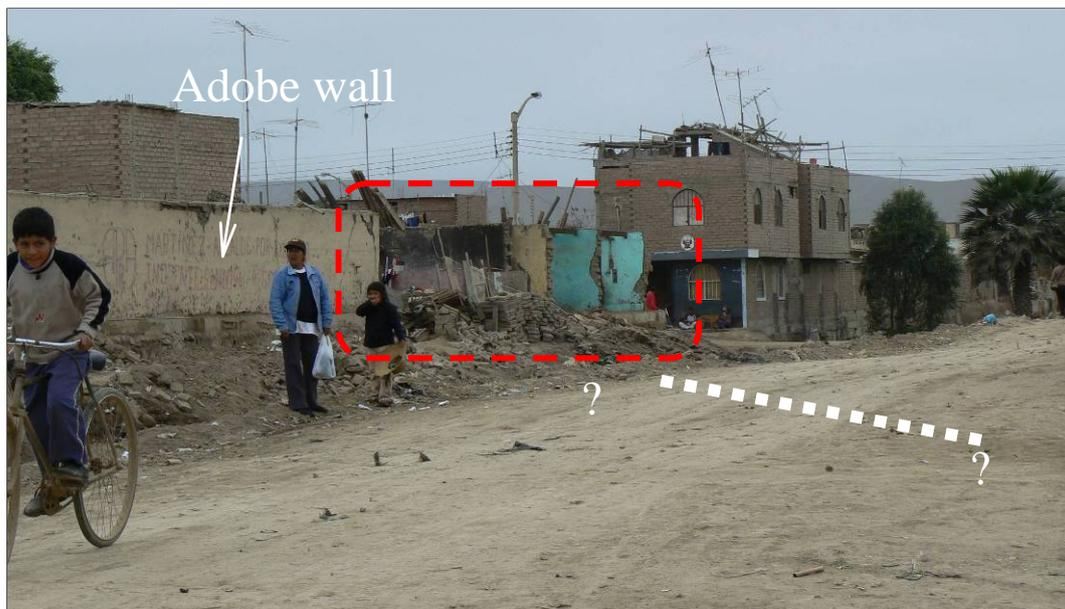
*Fig. 3.11. Collapsed adobe house due to large ground cracks in Nuevo Monterrico. The local people told us the crack crossed the street. The adobe wall to the left did not collapse.*
