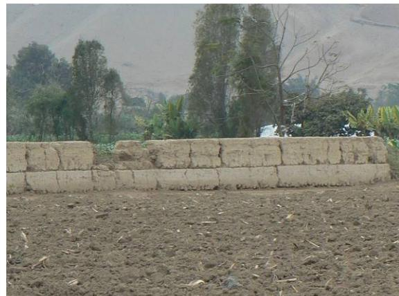
Fig. 4.2 Rammed earth or *tapial*. Note the vertical and horizontal cold joints showing different construction stages
