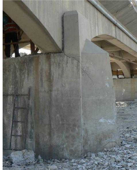
*Fig. 5.30 Cracks in the wing of the pillar with fixed bearing*
