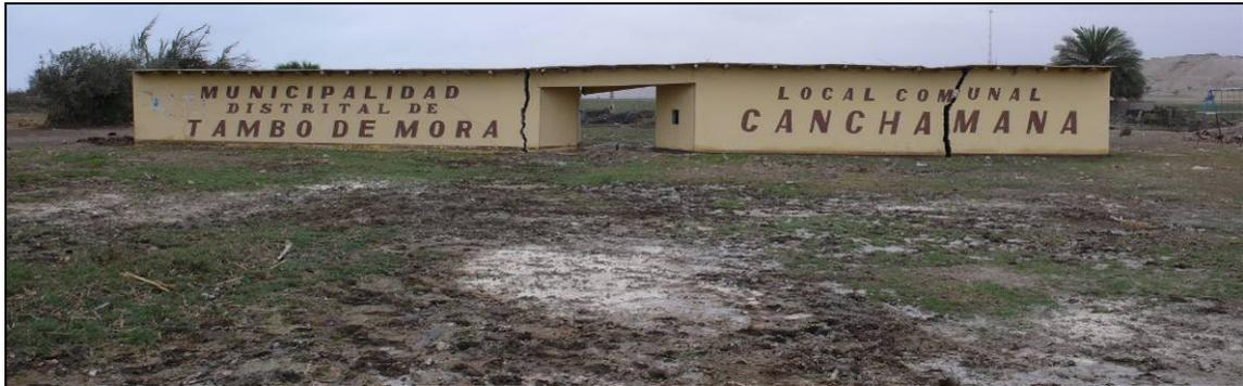
*Fig. 3.26. Severely damaged community building in Canchamana, with liquefaction traces in the foreground.*
