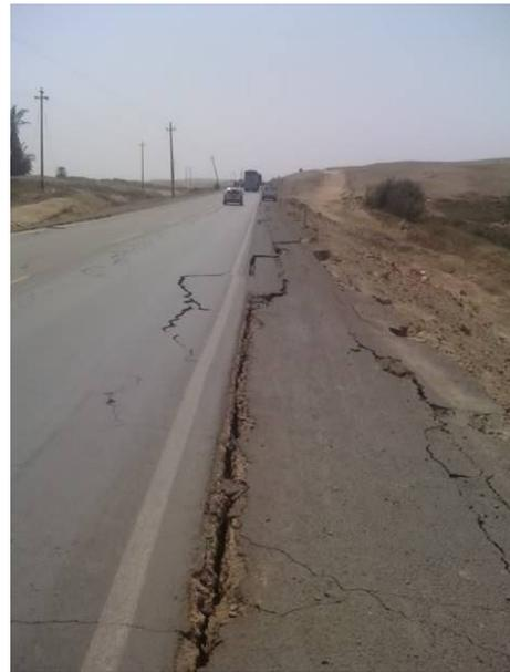
*Fig. 5.5. Shoulder settlement and displacement*
