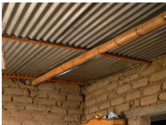
Fig. 4.10 Light gage steel plate roof
