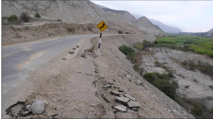
*Fig. 5.12. Slope failure at Canete-Yauyos road (Km. 23)*
