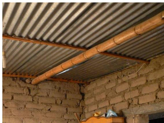
Fig. 4.10 Light gage steel plate roof
