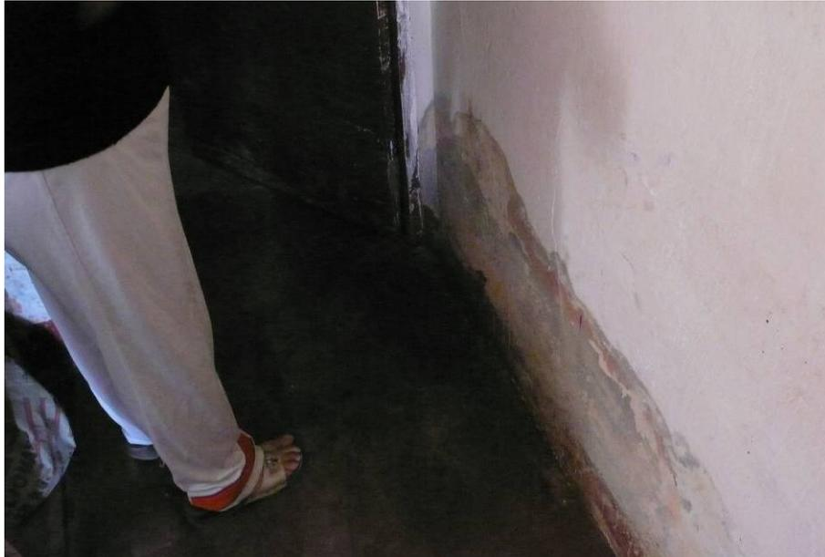
*Fig. 3.15. Foundation problems in Guadalupe: Miscoloring due to moisture absorption by adobe wall. The moisture weakens the structural properties of the wall, thereby the earthquake resistance of the house, and it also constitutes general health threat.*
