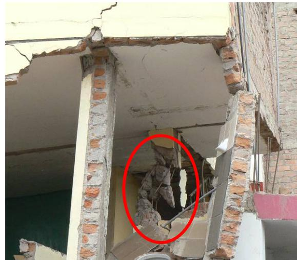
Fig. 4.63 Insufficient column shear reinforcement.
