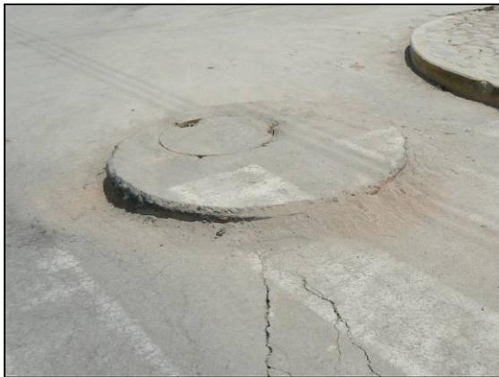
*Fig. 3.40. Manhole pushed up and surrounded by ejected fine sand. Northwest of Pisco (S13 42.343 W76 13.029)*
