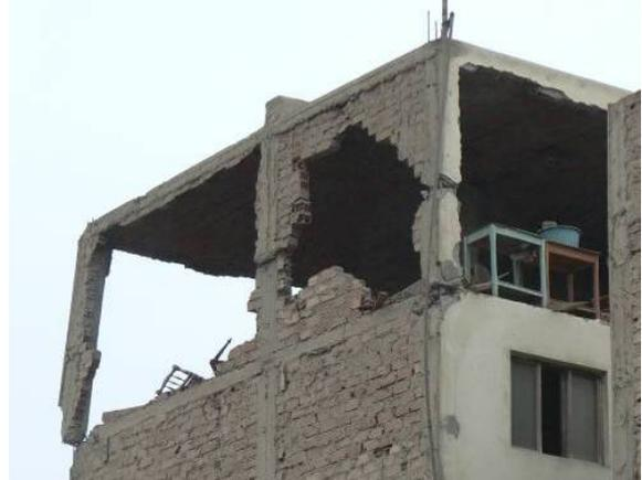
Fig. 4.30 Detail of the 5<sup>th</sup> story of the building to the left. Note the small amount of reinforcement in the columns. The failure pattern suggests that the columns were built first and then the brick wall.
