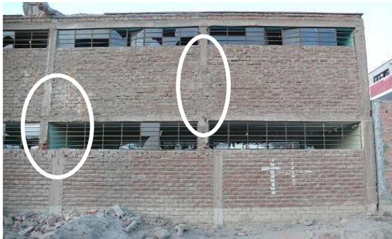
*Fig. 4.52 Bad construction example in Los Molinos, Ica*
