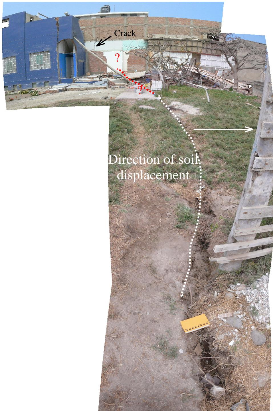
*Fig. 3.18. Soil displacement crack next to old building. (blue mark in Fig. 3.17). The crack probably continues in front of and/or beneath the building and then up through the confined masonry wall as marked by the black arrow. (The curvature of the building top is due image distortion, it should be a straight line.)*
