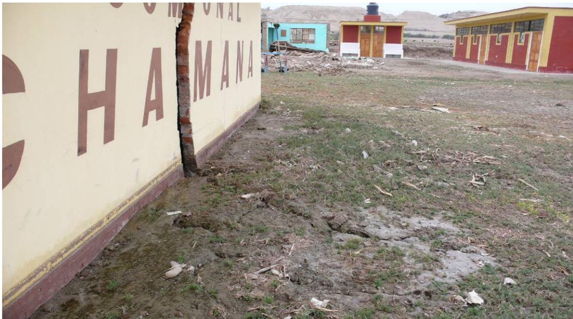
*Fig. 3.27. Severely damaged community building in Canchamana, with liquefaction traces in the foreground and well behaved red school building in the background.*
