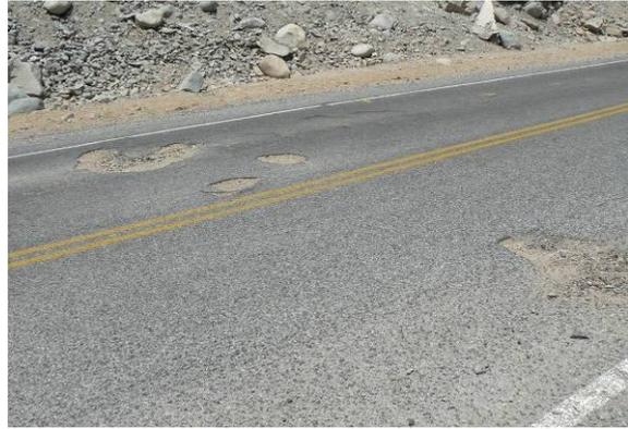
*Fig. 5.6. Road distortion due to liquefaction*   *Fig. 5.7 Pot holes caused by rock falls induced lateral spreading*
