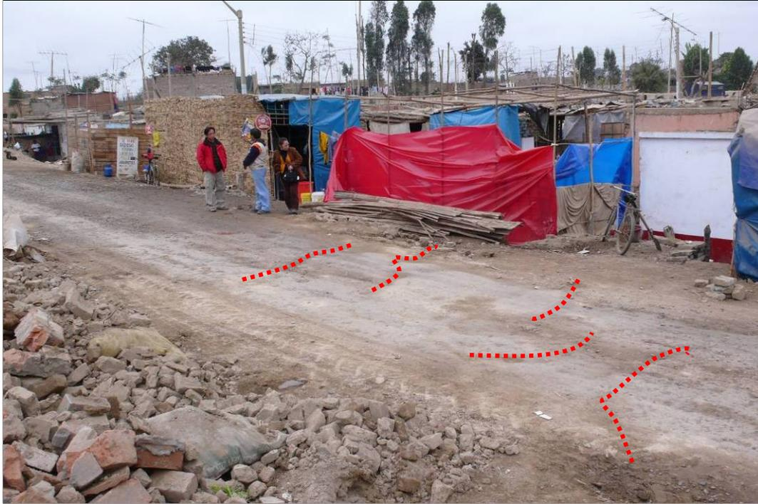
*Fig. 3.10. Large ground cracks in Nuevo Monterrico crossing road at point 61 with destroyed houses in the back ground.*
