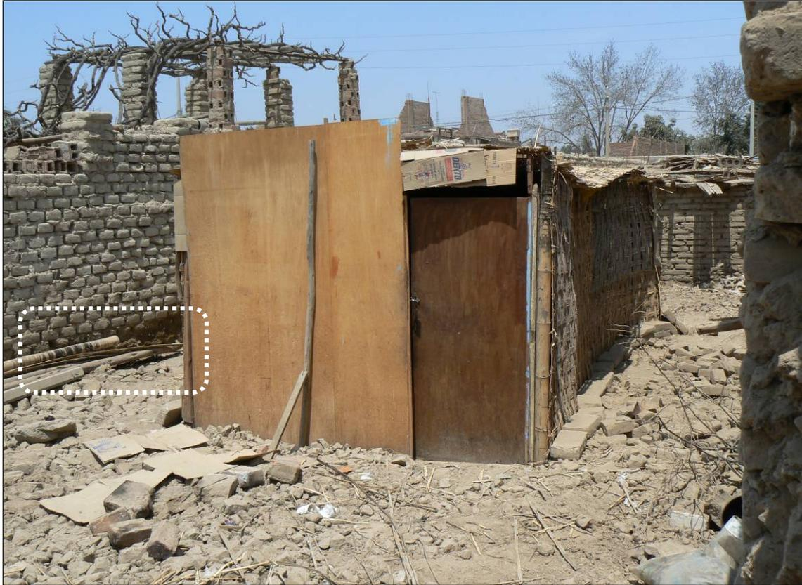
*Fig. 3.16. Temporary self-built house. The original house collapsed in the earthquake. The dashed box shows how the lower part of the wall is darker due to moisture absorption.*
