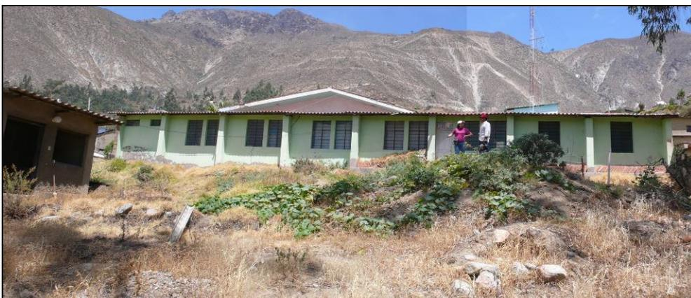
*Fig. 3.13 Health center in Huaytara with cracks in walls due to foundation differential settlement.*
