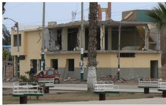
*Fig. 4.26 Collapsed façade wall due to lack of confinement (Sunampe, Chincha)*
