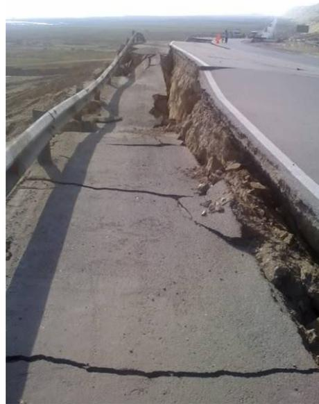
*Fig. 5.8 Lifted shoulder at Playa Jahuay. South Pan-American Highway*   *Fig. 5.9 Road failure due to lateral spreading at the foot of the slope. South Pan-American Highway*
