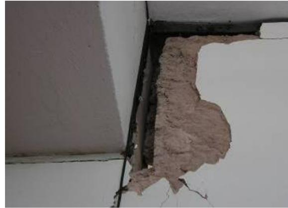
Fig. 4.55 Joint between brick partition and RC structure filled with mortar
