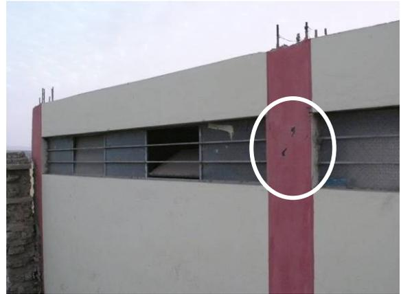
Fig. 4.47 RC-buildings with masonry panels suffered slight shear damage (Beatita de Humay School, Humay)
