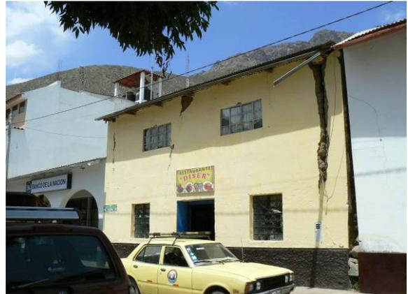
*Fig. 4.18 Adobe house with cracks at wall intersections (Huaytara, Huancavelica)*
