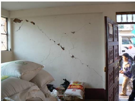
Fig. 4.31 Shear failure of masonry wall due to excessive interstory drift
