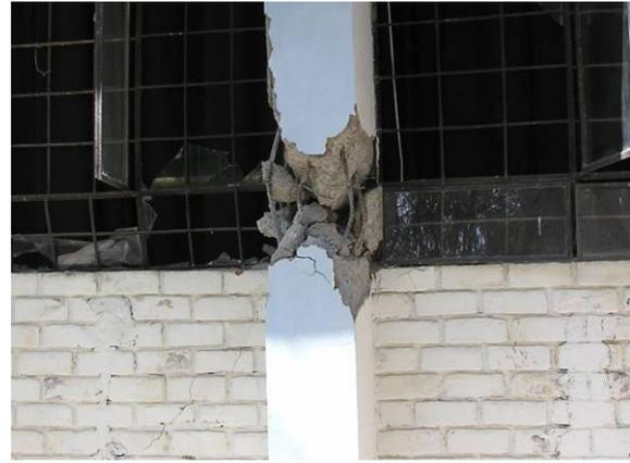
*Fig. 4.59 Insufficient shear reinforcement*
