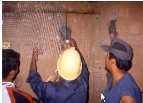
Step 2. Open 5-cm (2-inch) square holes every 50 cm (20 inches) at the intersection of vertical mesh strips. Insert small steel connectors into each hole, moisten the interior and fill them with 1:4 cement:sand mortar.
