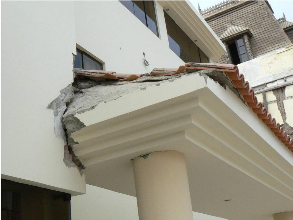
*Fig. 3.23. Close up of hotel damage. Relative ground movement, due to liquefaction, between the columns of the exterior roof structure and the building, caused the cracks.*
