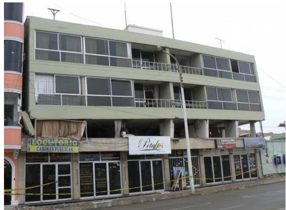
*Fig. 4.35 Soft-story failure due to insufficient stiffness in one direction (Pisco, Ica)*
