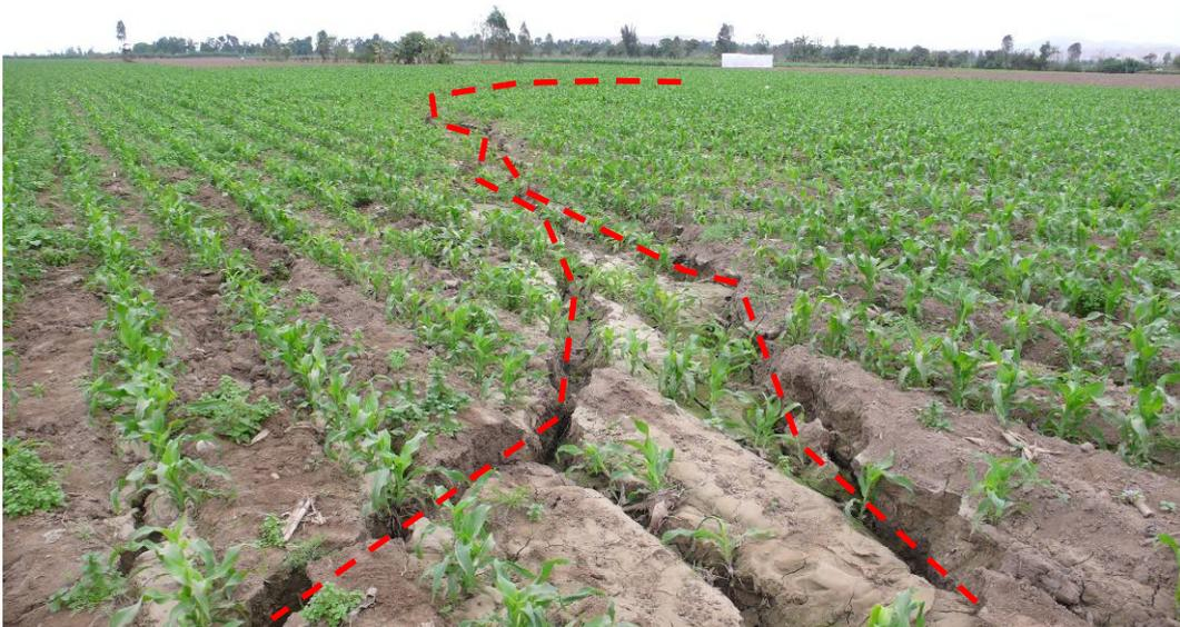
Fig. 3.7. Photo of large ground cracks at GPS points 41-46 in Nuevo Monterrico agriculture field. (Photo taken at red dot in Fig. 3.6.)
