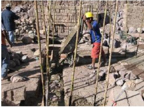
Step 1. Foundation. No reinforce beam W= 55cm H=80cm. Vertical reinforcement is fixed to the beam.
