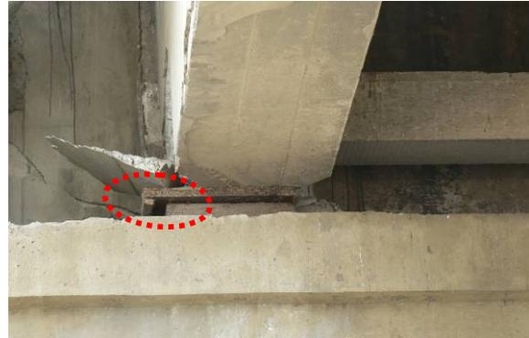
Fig. 5.23 Movable bearing at the southern abutment
