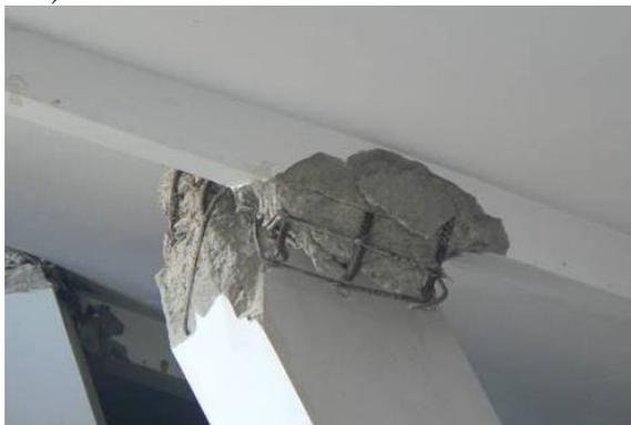
*Fig. 4.34 Beam-column joint detail of building in Fig. 4.32.*
