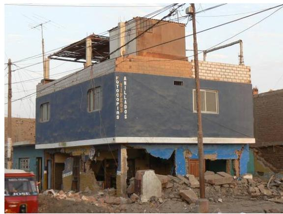
*Fig. 4.8 House with 1<sup>st</sup> story made of adobe and 2<sup>nd</sup> story made of confined masonry. In this case, RC columns were cast in the existing adobe walls to support the 2<sup>nd</sup> story.*
