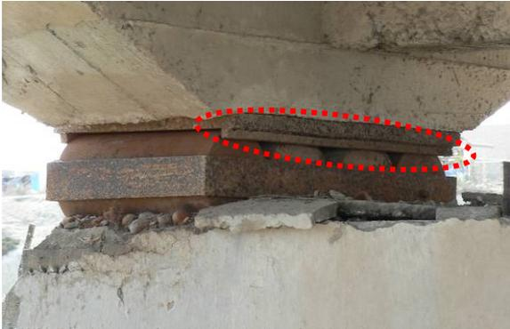
Fig. 5.22 Movable bearings on the pillars
