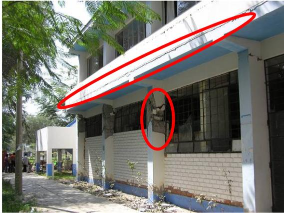
*Fig. 4.58 Chemistry Faculty Building with short column failure and parapet damage*
