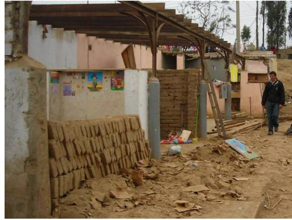
*Fig. 6.12 Adobes from collapsed walls are kept to be used as construction material*
