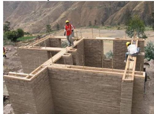
Step 4. Ring beam. Timber beams are fixed the top of adobe wall. (7.5x7.5cm)
