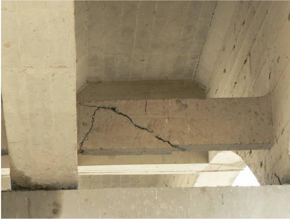
*Fig. 5.29 Damaged transverse beams*
