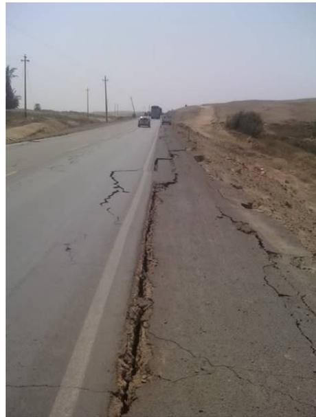
*Fig. 5.5. Shoulder settlement and displacement*
