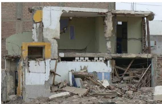
*Fig. 4.25 Load bearing wall made of pandereta bricks and poor steel reinforcement in the confinement (Pisco, Ica)*
