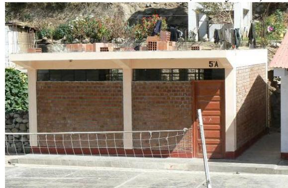
*Fig. 4.45 Confined masonry building did not suffer any damage, (San Juan Bautista school, Huaytara)*
