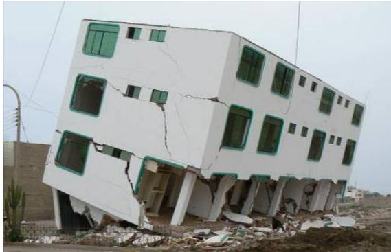
*Fig. 4.32 Apartment building with inadequate stiffness distribution (Pisco, Ica)*
