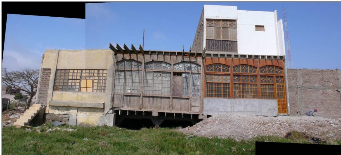
*Fig. 3.20. Old building located close to the ocean in Pisco that performed well even large liquefaction displacement was observed. In the central part a pile foundation is visible.*
