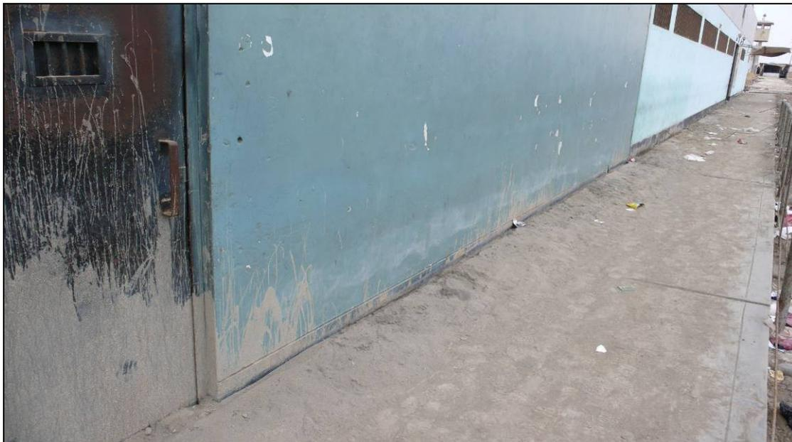
*Fig. 3.29. Liquefaction splashed all the way to the top of Prison building door.*
