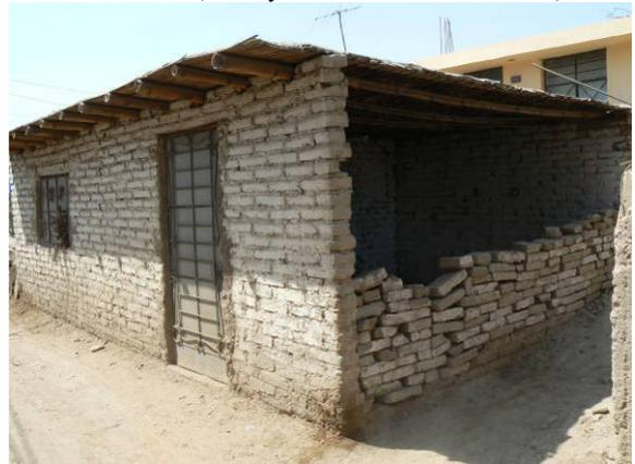
*Fig. 4.20 Wall partial collapse. Walls supporting the roof are standing. This was observed at several locations (Ica).*
