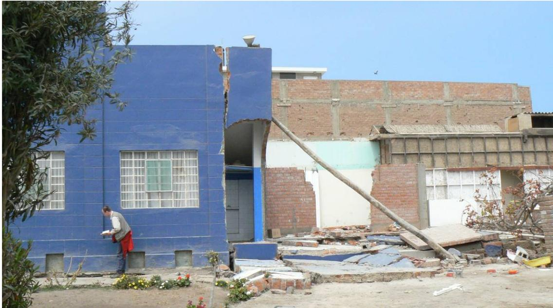
*Fig. 3.19. 10-15 cm soil settlement around blue building on pile (?) foundation. Blue mark in Fig. 3.17*
