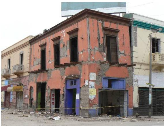
*Fig. 4.7 Old traditional structure with 1<sup>st</sup> story made of adobe and 2<sup>nd</sup> story made of quincha*
