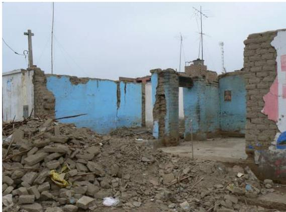
*Fig. 4.21 Collapsed adobe house (Nuevo Monterrico, Canete)*
