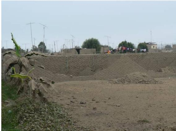
*Fig. 4.23 RC confined adobe wall (in the back), survived the quake, and unconfined adobe wall (front) failed out-of-plane (San Luis, Canete)*
