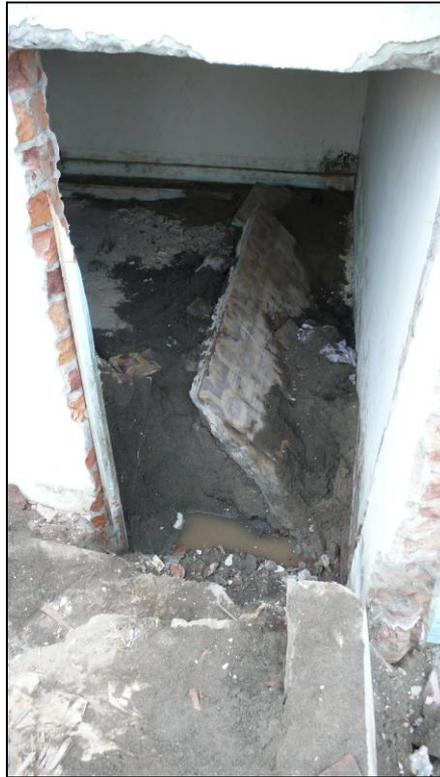
*Fig. 3.28. Foundation pushed up due settlement the building.*
