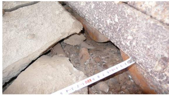
*Fig. 5.26 No bottom steel stoppers were found at the pillar movable bearing.*
