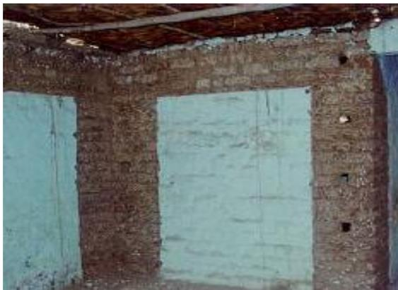
Step 1. Remove the existing gypsum or mud plastering.
