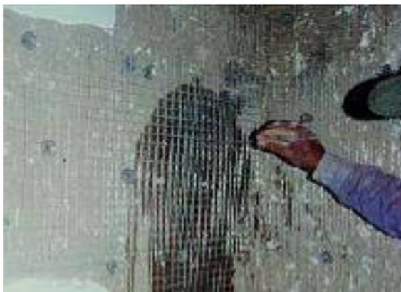
Step 3. Fasten the vertical mesh strips to the adobe wall with nails, and then the horizontal strips. The usual width of mesh strip was 45 cm (18 inches). Bend the ends of the connectors 90° and nail them to the adobe wall.
