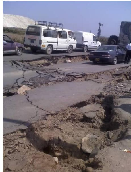
*Fig. 5.3. Liquefaction induced embankment failure*
