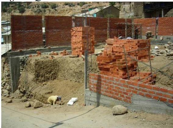
Fig. 4.5 *Confined masonry in process of construction*
