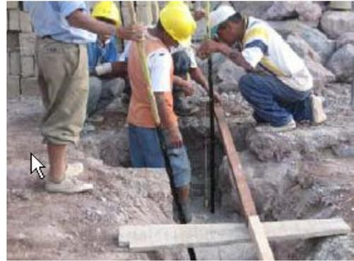
Step 2 Vertical Reinforcement. Cans are placed on center of wall every 80cm, buried 10cm.
