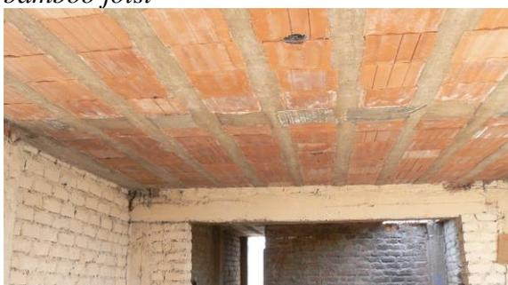
Fig. 4.11 RC concrete joist with clay hollow bricks
