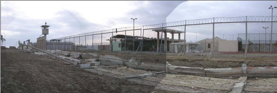
*Fig. 3.30. Collapsed wall at Chinchá prison due to large ground deformation*
