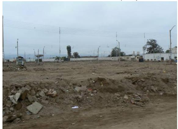
*Fig. 4.22 Totally collapsed adobe houses (Hualcara, Canete) – The hanging electric lines show the location where houses used to be.*
