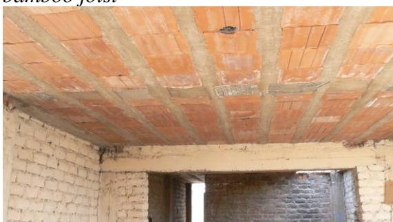
Fig. 4.11 RC concrete joist with clay hollow bricks
