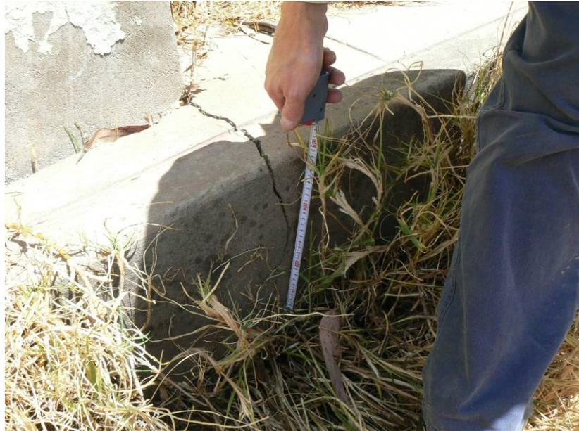
*Fig. 3.14. Huaytara health center foundation slab with 1cm wide crack due to differential settlement.*
