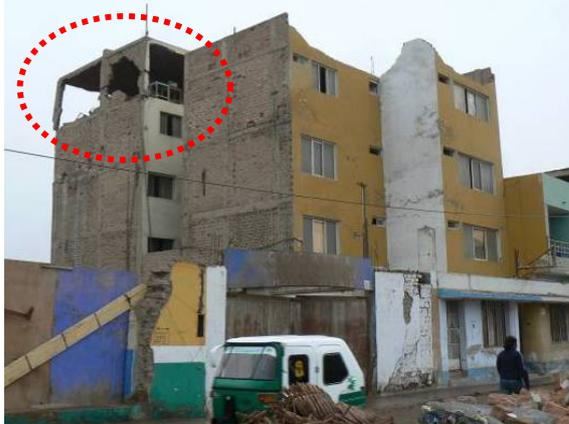
Fig. 4.29 5-story confined masonry building apparently built in several stages (Pisco, Ica)
