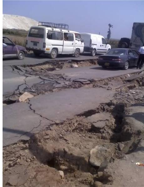
*Fig. 5.3. Liquefaction induced embankment failure*
