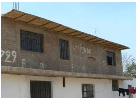
Fig. 4.9 Roof made of straw mat and bamboo joist
