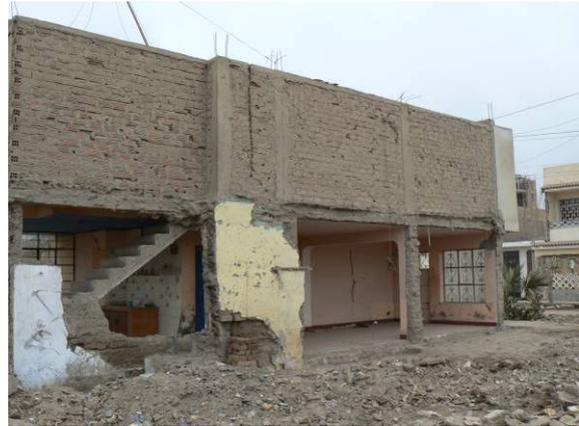
*Fig. 4.24 The house shown "borrowed" the wall of the neighboring adobe house, which collapsed. Only the RC columns built to support the 2<sup>nd</sup> floor survived. (Pisco, Ica)*
