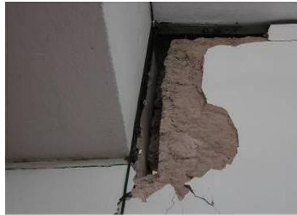
Fig. 4.55 Joint between brick partition and RC structure filled with mortar
