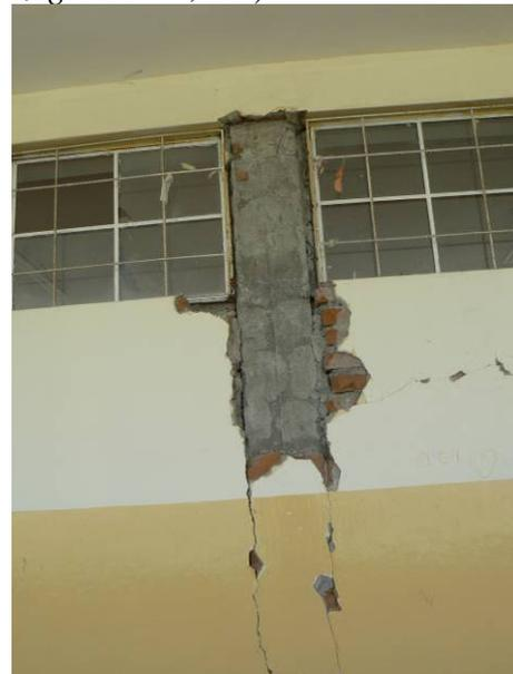
Fig. 4.51 Insufficient clearance between masonry panels and RC structure (San Luis Gonzaga School, Ica)
