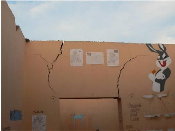
*Fig. 4.27 Lack of confining beam (Tambo de Mora, Chincha)*
