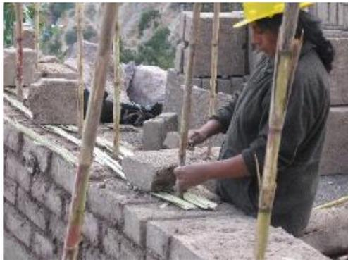
Step 3. Horizontal reinforcement. Crushed canes are placed every four layers and connected to vertical canes with nylon strings.
