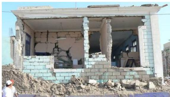
Fig. 4.40 Concrete block wall collapsed out-of-plane
