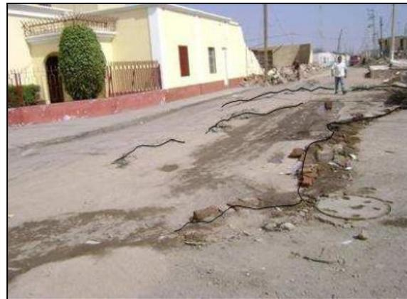
*Fig. 3.41. Sub parallel cracks with lateral spread along the streets in the southwest of Pisco (Rodriguez et al [16])*
