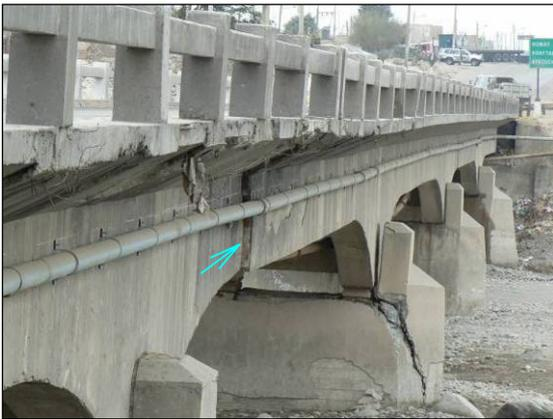
*Fig. 5.25 Bridge slab displacement (picture taken towards the north). Arrow indicates the gap corresponding to the southern 8 cm gap shown in Fig. 5.24*
