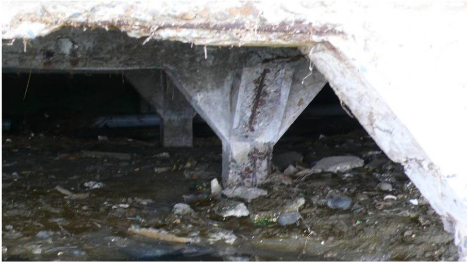
*Fig. 3.21. Close up of pile foundation showing corroded reinforcement bars. The age of building foundation is unknown, but many of the buildings in these area were up to 100 years old.*
