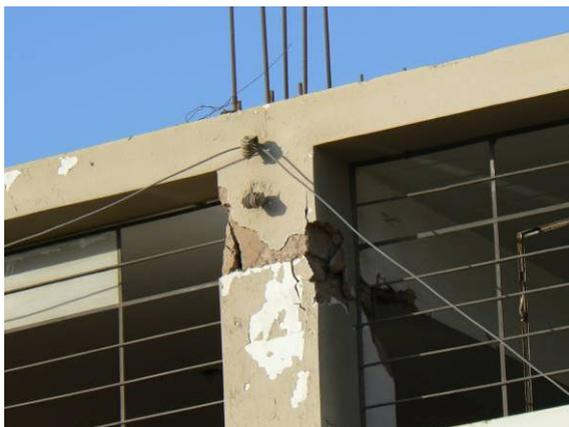
*Fig. 4.36 Shear failure of beam-column joint (Parcona, Ica)*
