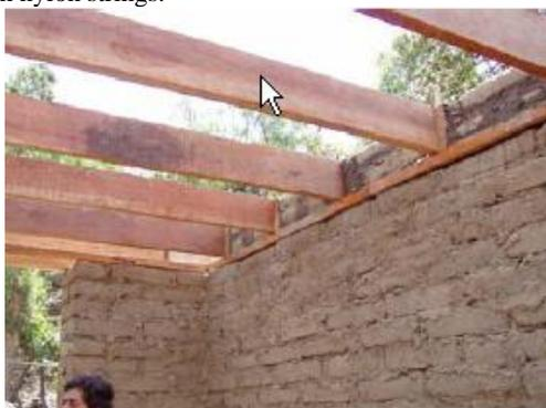
Step 5. Roof. Timber beams are placed every 60 cm (5x20cm)
