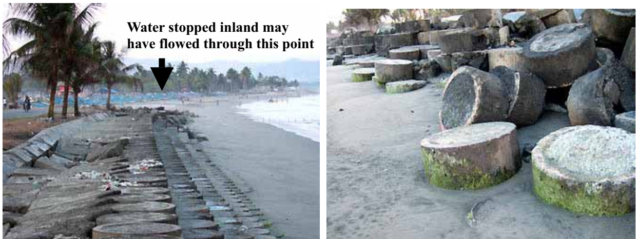
Figure 6. Cylindrical retaining blocks piled up along the beach.
