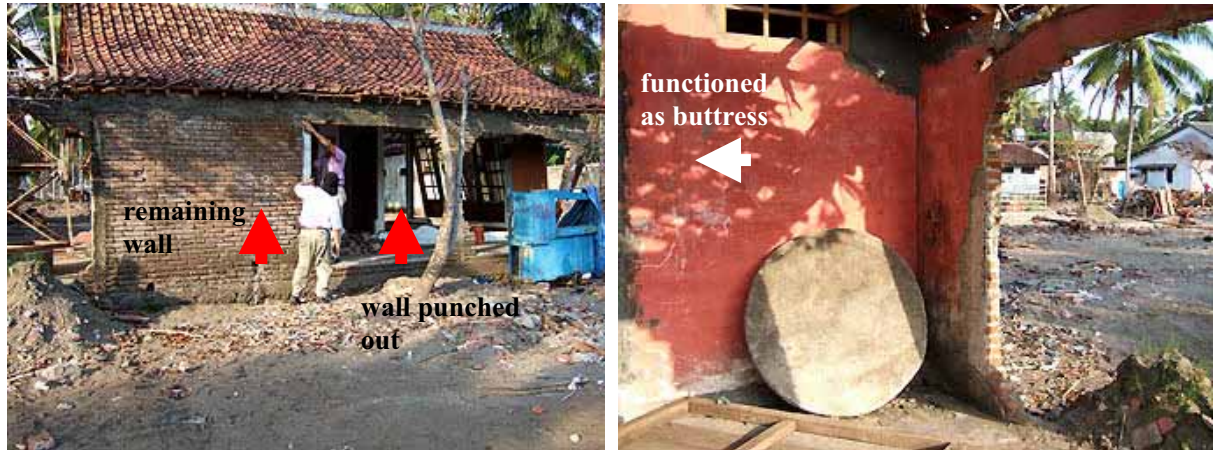
Figure 2. Tsunami at Pangandalan punched out brick walls
