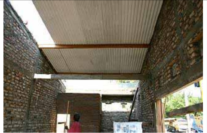
Beams along the top ends of walls are seen.
