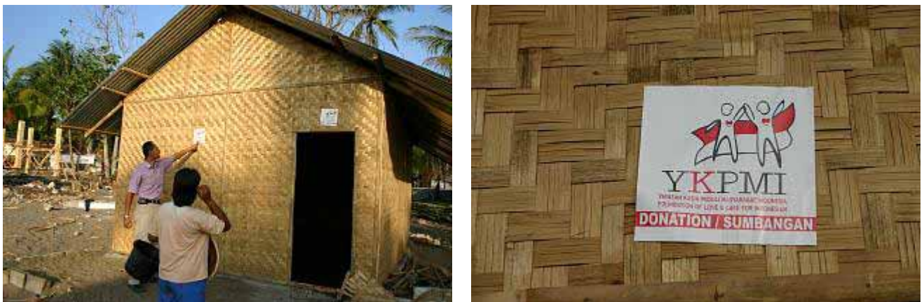
Figure 4. Bamboo-woven panels for survivors' houses
