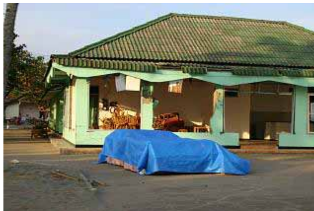
Figure 3. It may be shop house, front face seems to be windows, these are destroyed in a early stage of Tsunami, water pressure would be released.
