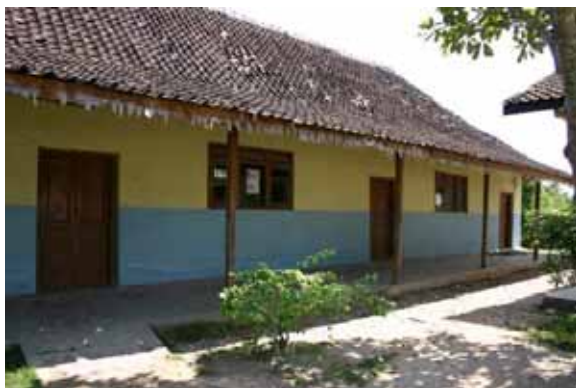
Building #2: Stone masonry structure
