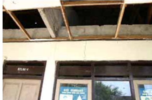
Building #1 : RC column and beam
