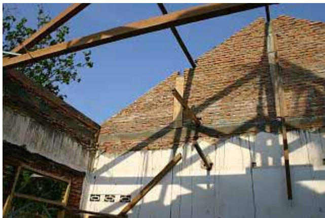
2006.09.16 SD2 Parangtritis Under repair
