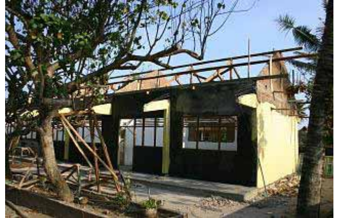
2006.09.16 Repairing. Top ends of walls are connected with RC beams
