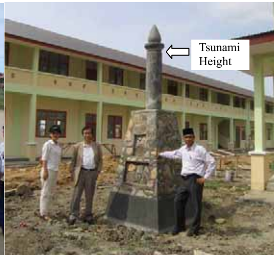
Figure 13. A Tsunami Pole at a School
