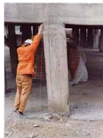
Photo 4 Contribution of nonstructural elements to soft first story (1992 Erzincan EQ)
