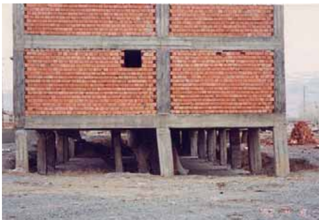
Photo 4 Contribution of nonstructural elements to soft first story (1992 Erzincan EQ)
