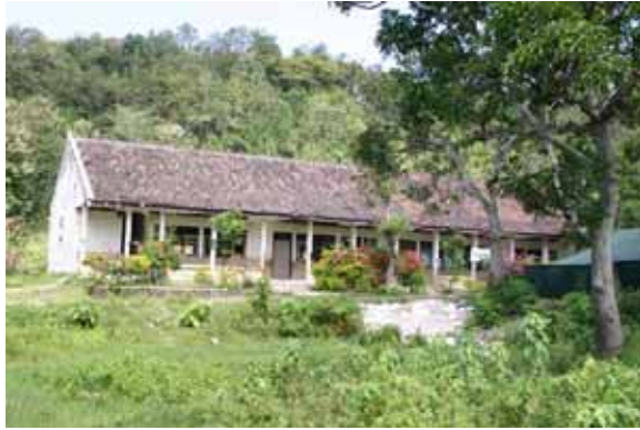
Building #1 : URM with RC columns
