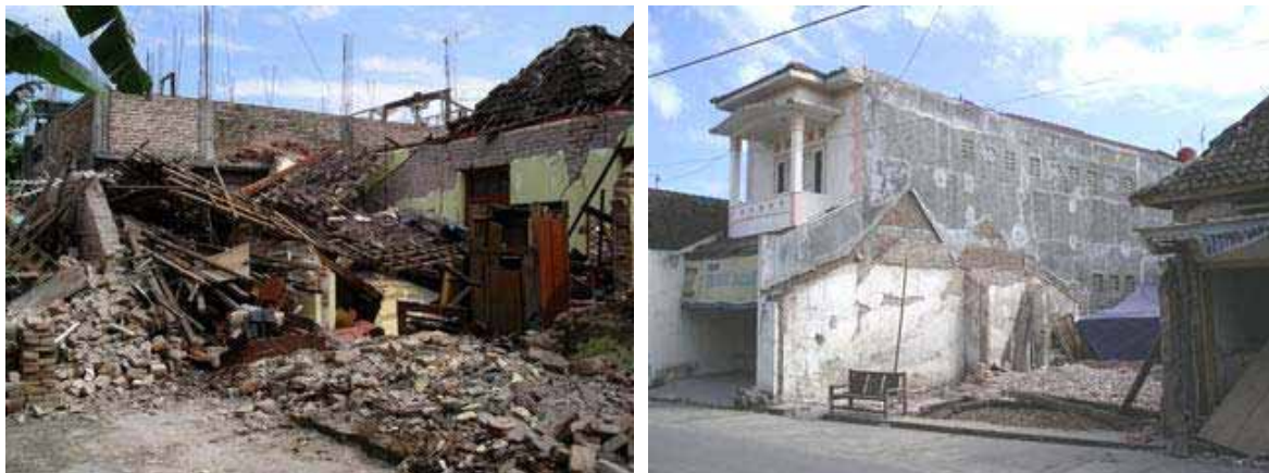
Photo 2 Devastated URM house
