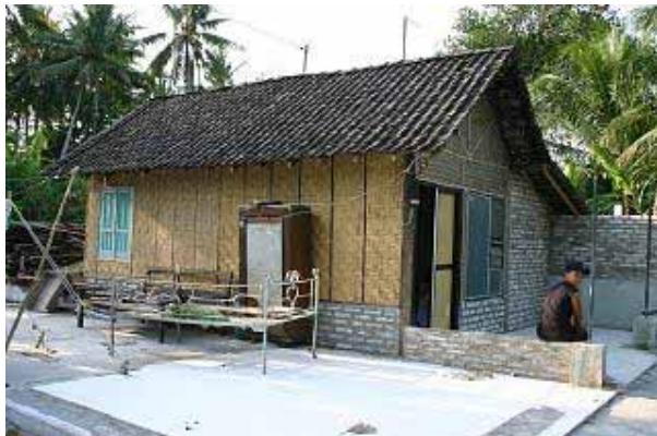
Bamboo house at Bantul
