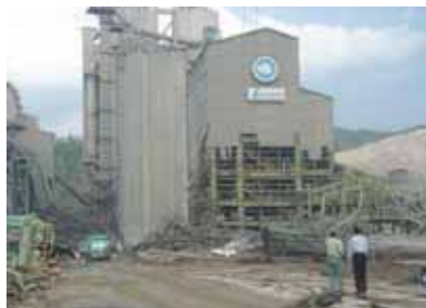
(a) Cement Factory
