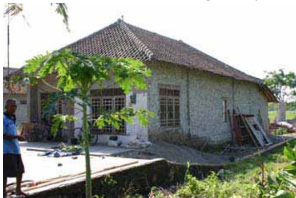
Photo 7 Stone masonry house
