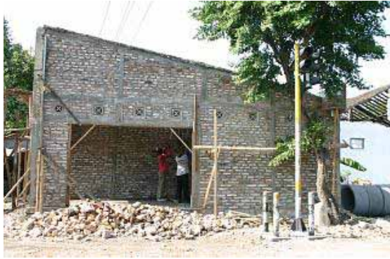
Shop house? At the corner of cross section of Bantul to Imogiri. RC frame confines brick wall.
