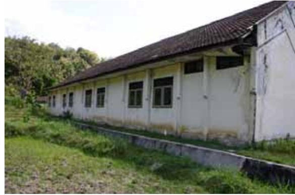
South side of building #1
