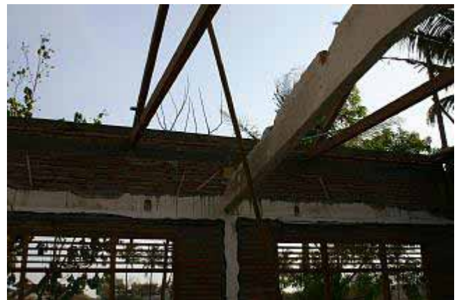
2006.09.16 SD2 Parangtritis Under repair
