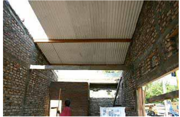
Connection beam is observed
