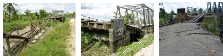
Figure 4: Damage of Lafau Bridge
