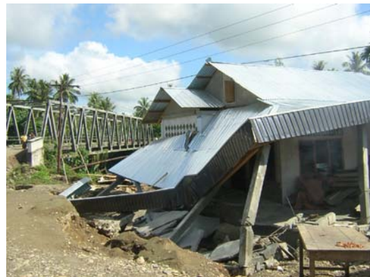
Photo 2 Liquefaction induced damage to buildings in Gunun Sitoli 2)
