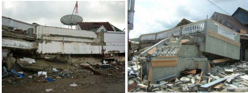
Figure 7: Pan cake failure of buildings
