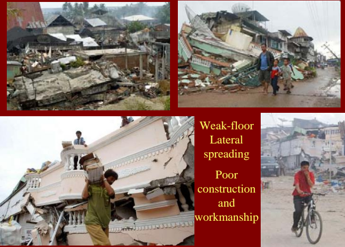
RC Building – Total Collapse – Weak Floor Phenomenon
