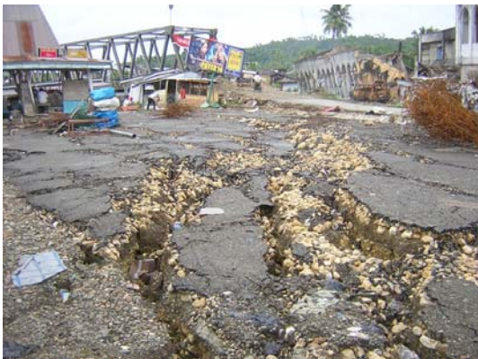
Photo 3 Lateral spreading due to liquefaction 2)
