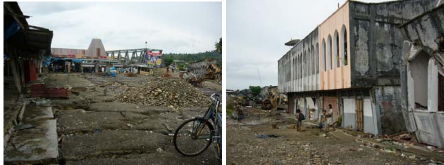
Figure 6. Effect of liquefaction and lateral spreading on RC building and truss bridge
