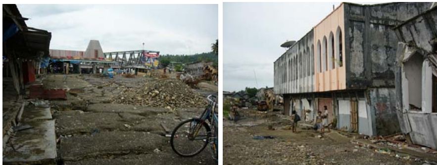
Figure 8: Effect of liquefaction and lateral spreading on RC building and truss bridge
