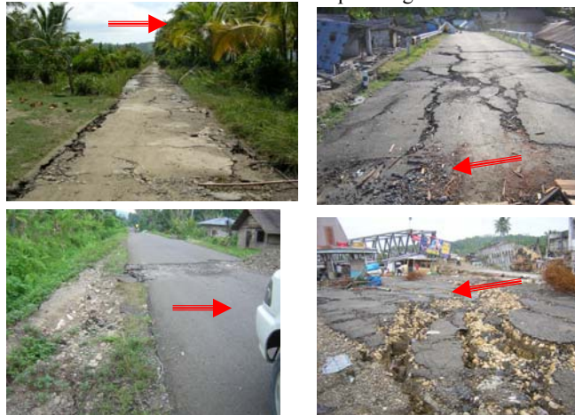
Settlement & Lateral Spreading
