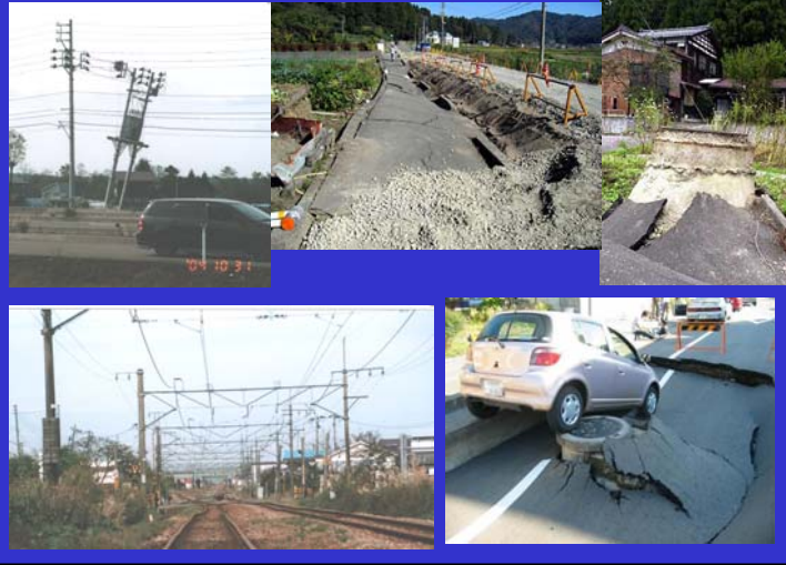
Lateral spreading, uplifting, sinking due to liquefaction
