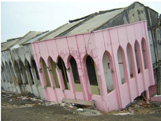
Photo 1 Liquefaction induced damage to buildings in Gunun Sitoli 2)
