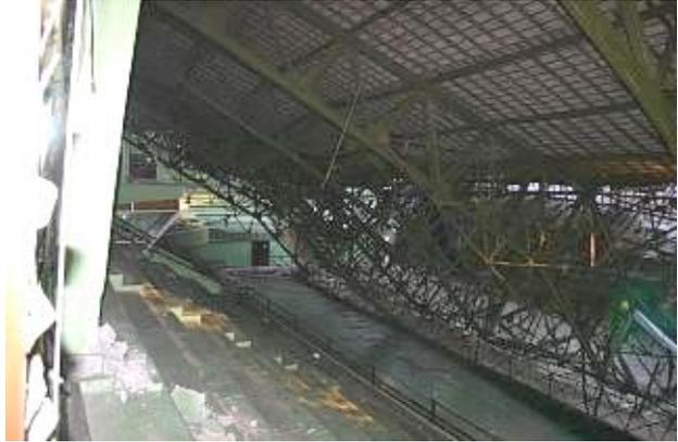
Amongrogo Sport Center / Collapsed roof system associated with column failure underneath
