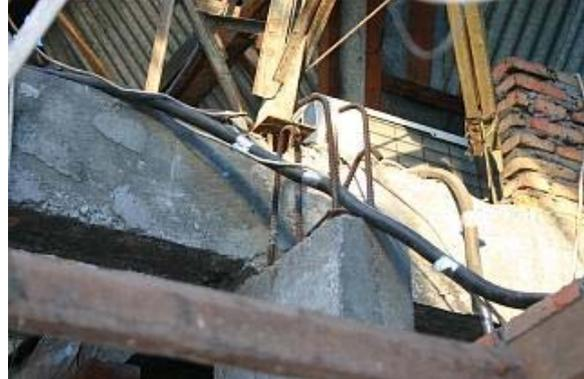
Damage to roof system above top story (some column rebar were not anchored to beams)
