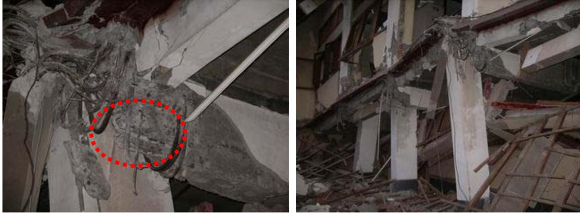
University of Economic Science (STIE) / Beam bottom rebars inadequately anchored to joints
