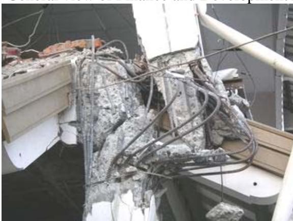
Beam-column joint failure
