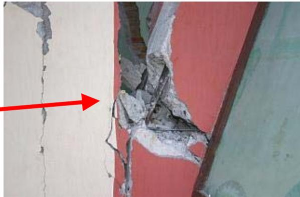
Heavy damage to RC columns and exposed rebars
