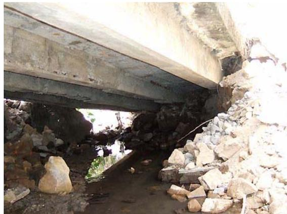
(c) Four simple beams support the deck.
