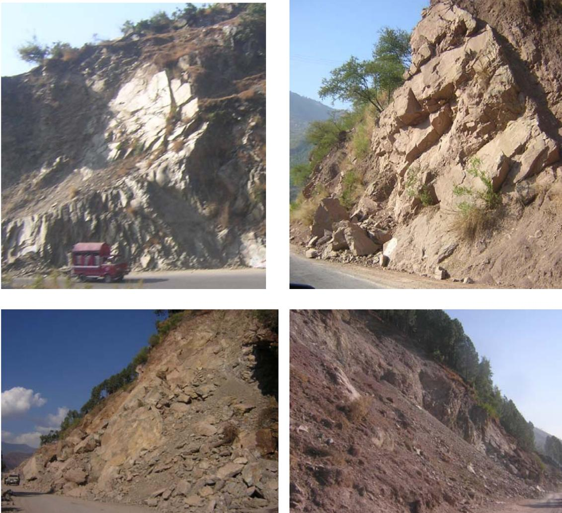
Figure 10.7 Some examples for planar sliding failure of rock slopes
