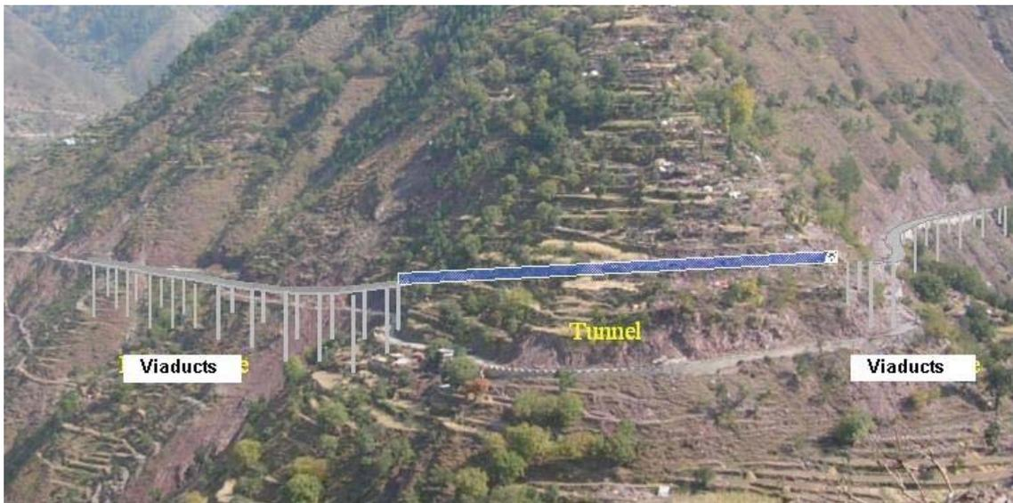
Figure 11.10 An example of combined viaduct-tunnel re-routing for Balakot area
