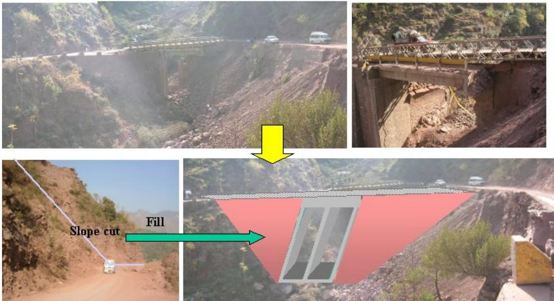
Figure 11.5 Recommendation for the construction of a box-culvert for the damaged bridge
