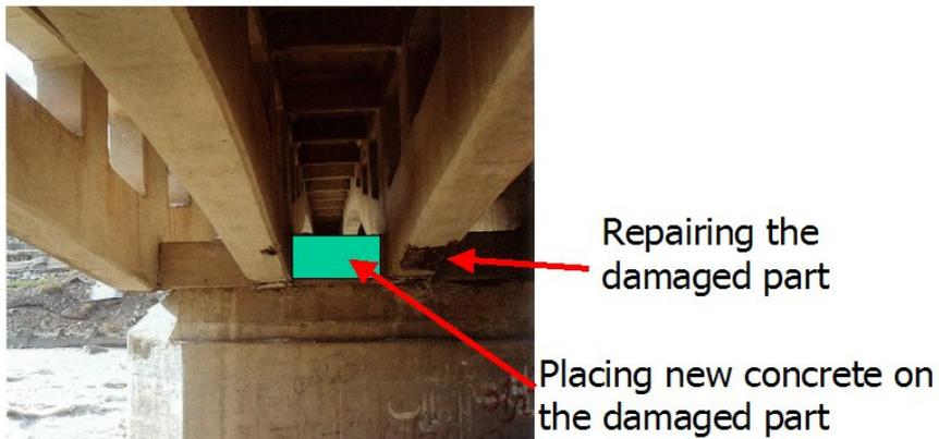
Figure 11.1 Recommendations of possible options for restoration of Balakot bridge
