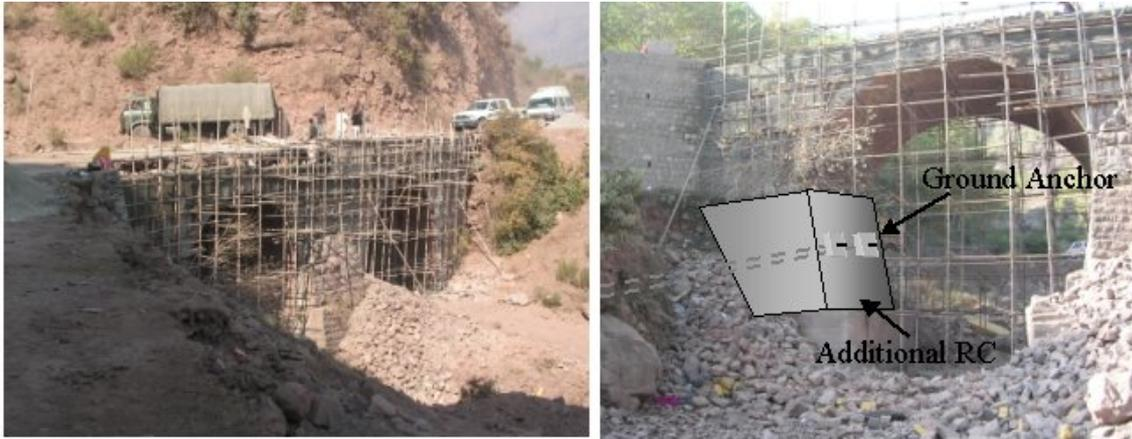
Figure 11.4 Recommendation for the restoration of the damaged arch bridge
