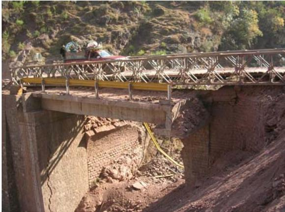
(a) RC bridge with masonry abutments
