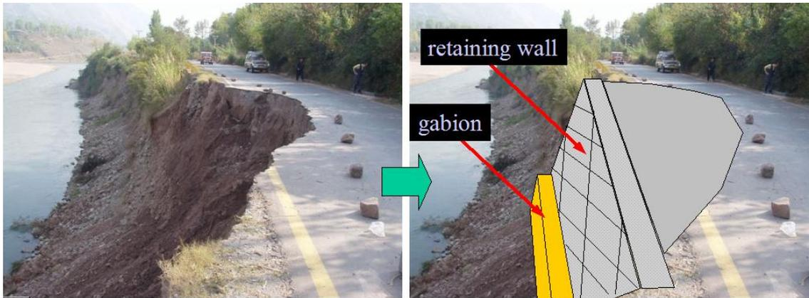
Figure 11.6 A recommended protection procedure for the collapsed section of the embankment.
