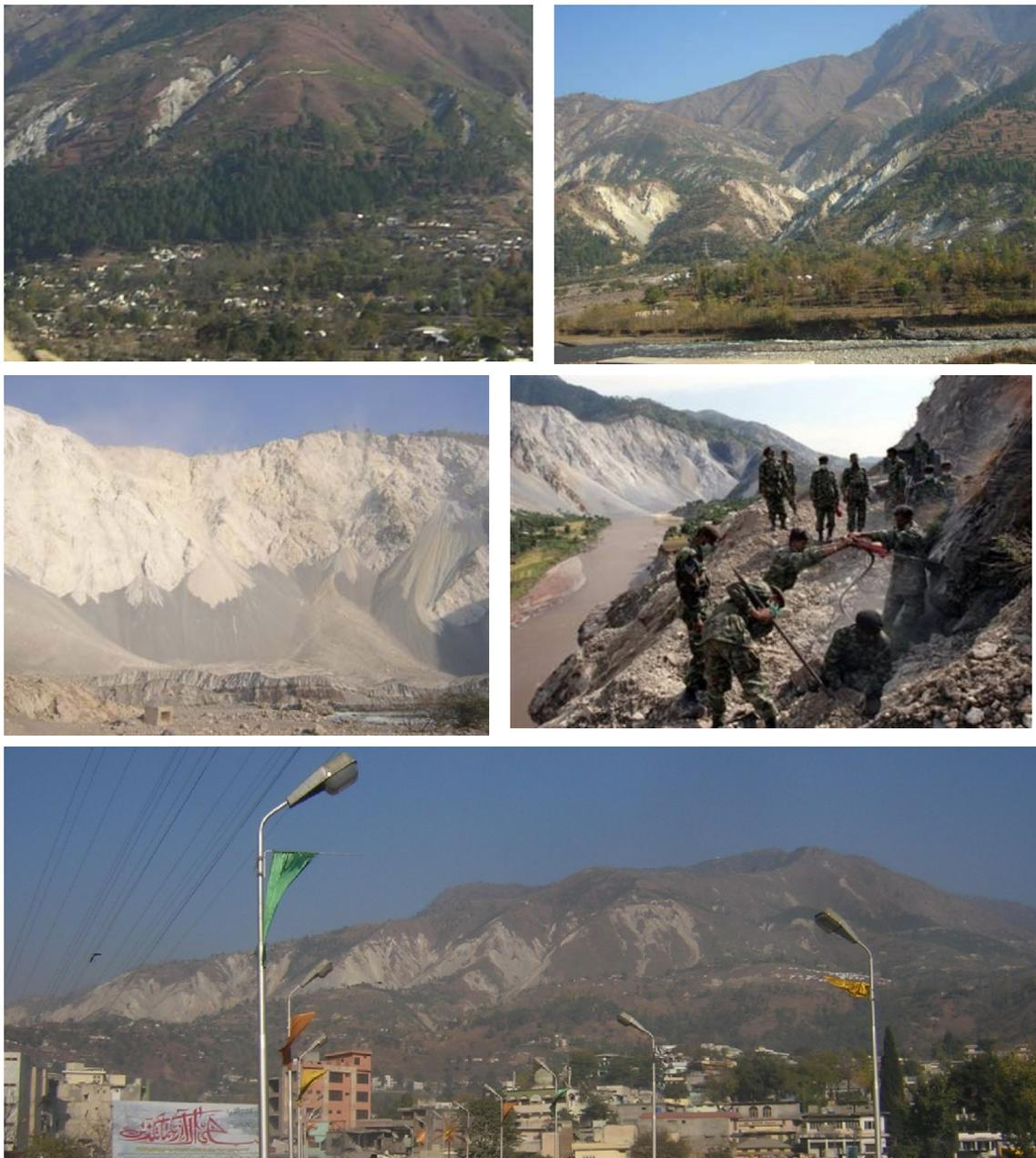
Figure 7.4 Slope failures observed in the regions of Balakot and Muzaffarabad
