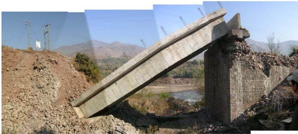
(c) Damaged RC bridge with masonry abutments
