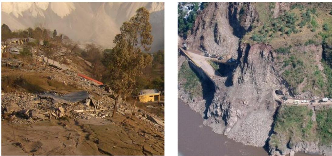
Figure 11.15 Some examples of slope failures in ground containing cobbles
