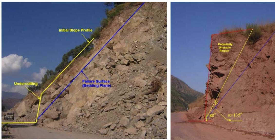
(a) Sliding slope failure due to undercutting (b) Stable slope against flexural toppling
