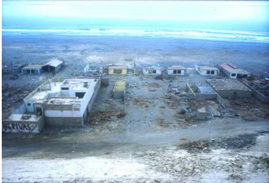
Figure 6.19 Damage of houses in Los Cerrillos (Location B in Figure 6.16 )
