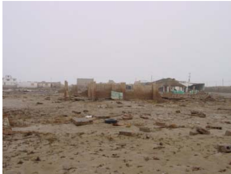
Figure 6.7 Completely destroyed houses at La Punta
