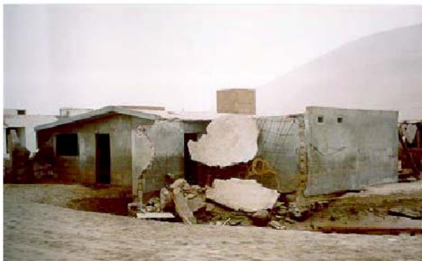
Figure 6.17 Destroyed dwellings by tsunami
