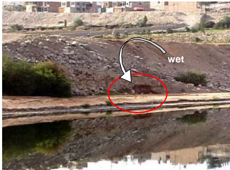
Figure 4.3. Embankment between the upper and lower ponds
