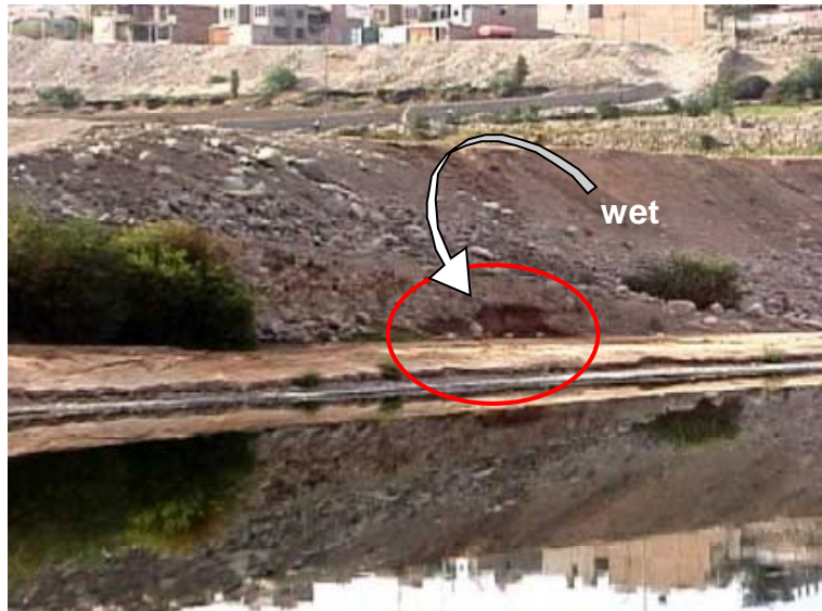
Figure 17. Embankment between the upper and lower ponds
