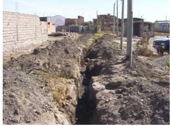
(b) Re-excavated drainage channel that was clogged with spread soil
