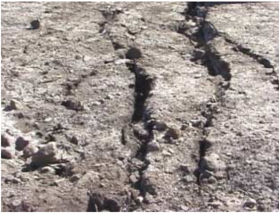
(c) Cracking in ground surface located at a horizontal distance of about 25 m from drainage channel
