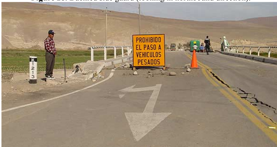
Figure 29. Settlement of bridge approach and cracking of road. Only one lane is open for traffic (looking in southbound direction).
