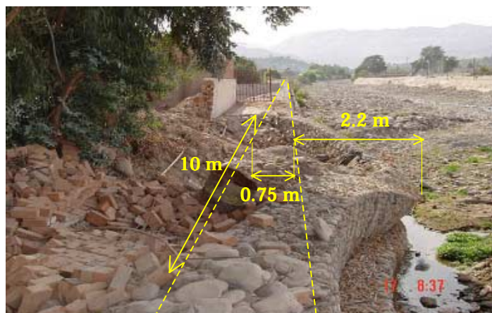
Figure 14. Deformed Gabion wall
