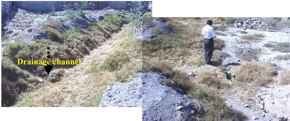
(a) Lateral spreading toward drainage channel
