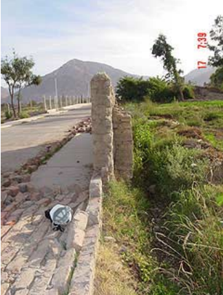
Figure 11: Standing adobe wall and fallen masonry wall.
