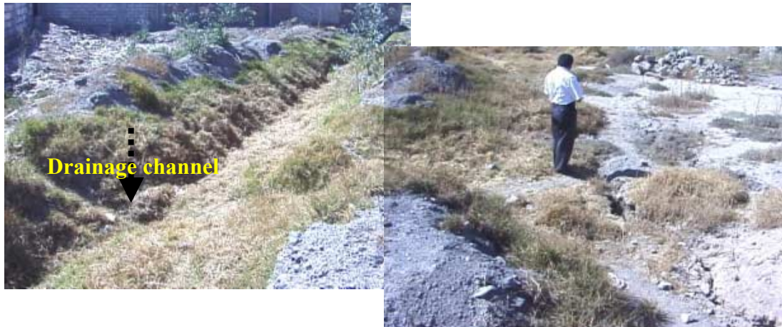
(a) Lateral spreading toward drainage channel
