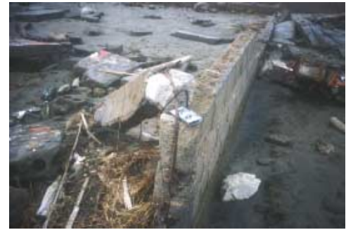
↑ (a) reinforcing bars bent by tsunami
