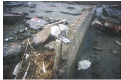
↑ (a) reinforcing bars bent by tsunami
