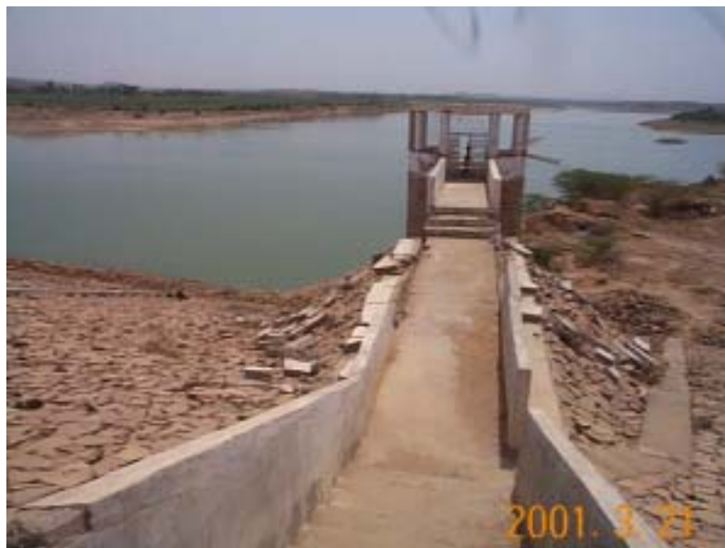
Figure 6.11 Water intake tower of Rudramata dam
