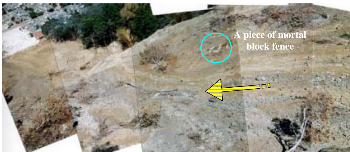
Fig. 1.5 Lower part of the hollow: A piece of mortar block fence (within the circle) is caught on the small amount of the soil mass stopped at the lower edge of the hollow.
