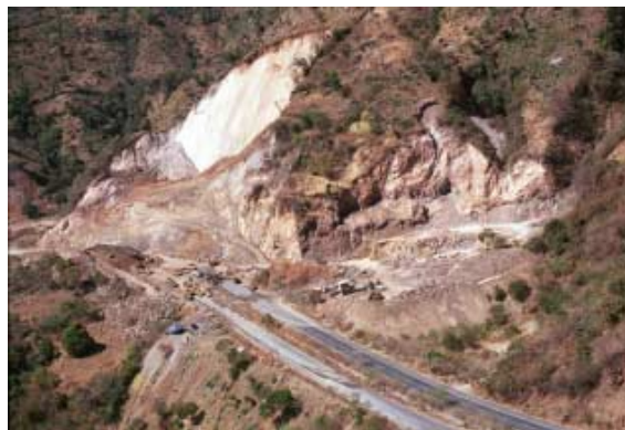
Figure 2.10 Blocked PanAmerican Highway, San Vicente
