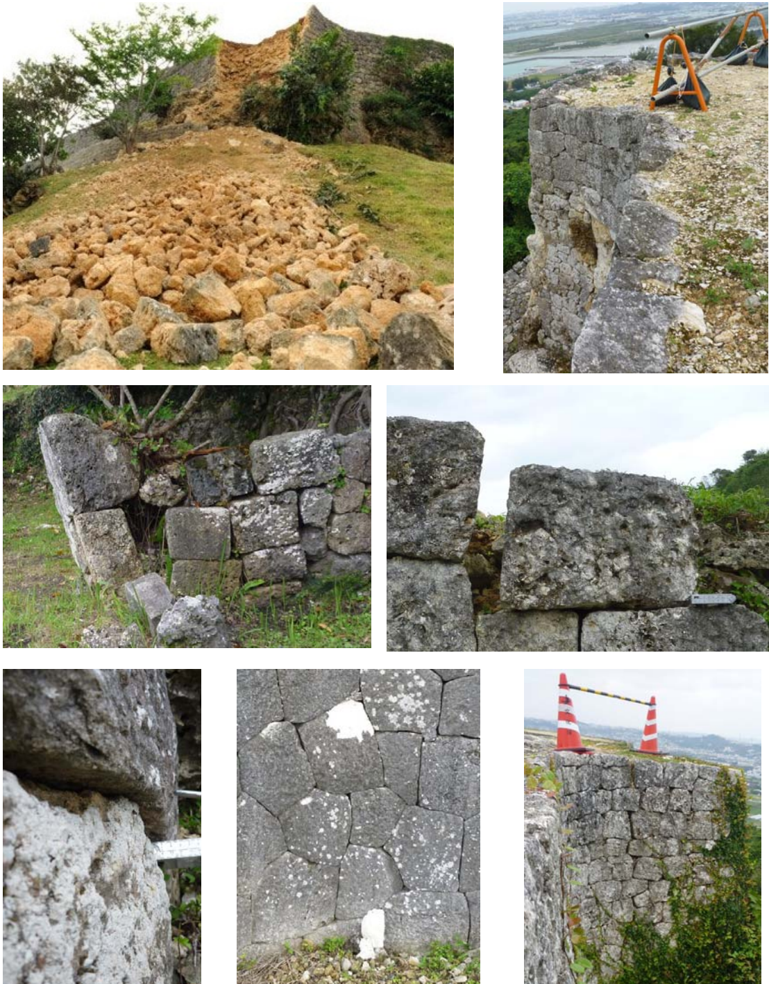
Figure 19: Collapse of the castle wall and dislocation or rotation of blocks and walls
