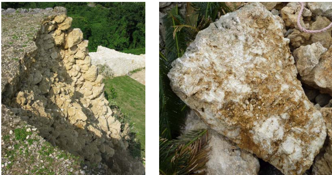
Figure 20: Close-up views of the collapsed wall and typical rock block
