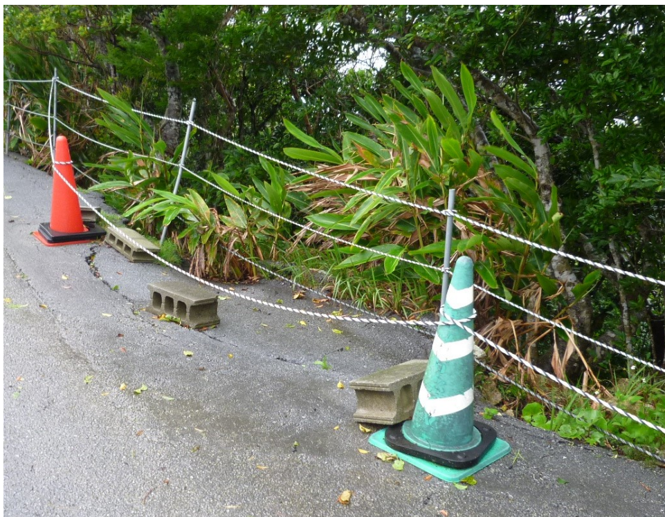
Figure 23: Partial failure of road embankment near Nakagusuku
