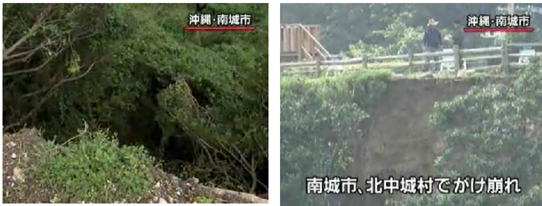
Figure 22: Slope failure in Nanjo City (from mass media)
