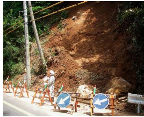
(b) Slope failure on Route 17
