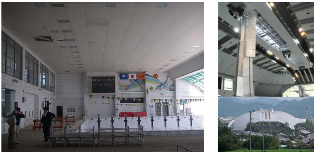
Figure 26: Fall of panels from the roof of swimming pools in Shizuoka
