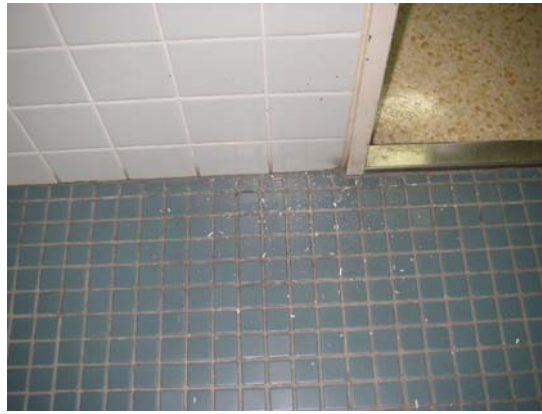
(c) Cracking in the unretrofitted floor of a retrofitted building
