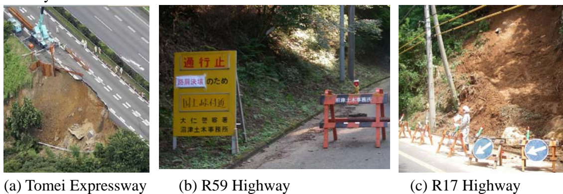
Figure 45: Damage to expressways and roadways
