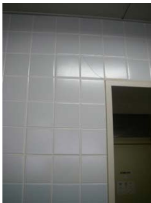
(c) Cracking in the unretrofitted floor of a retrofitted building
