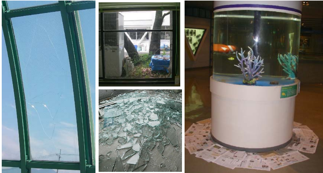
Figure 27: Examples of fractured or broken glasses of windows and aquarium
