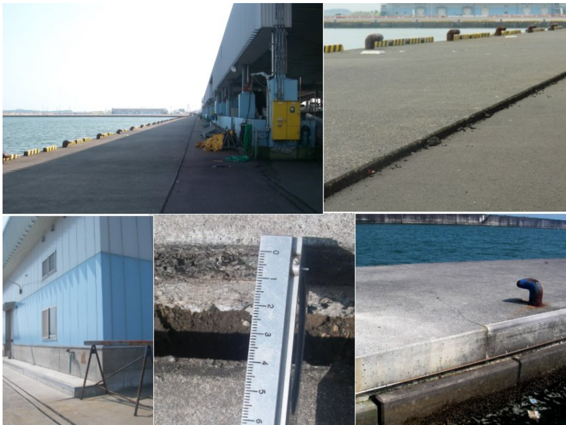
Figure 48: Damage at Yaizu new fishing port
