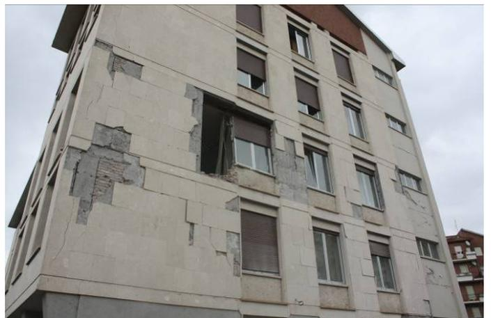
**Photo 13** Damage of joints and masonry walls
