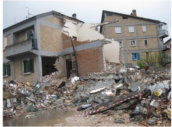
**Photo 22** Collapse of a two-story RC building
