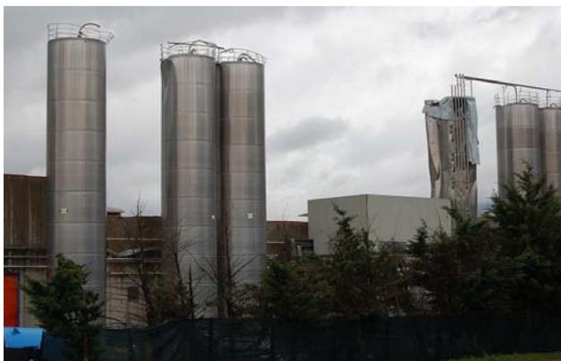
Photo 35 Buckled silos at VIBAC
