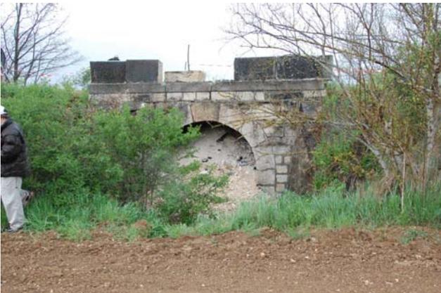
**Photo 31** Emergency repair of a stone masonry arch culvert (SR261)
