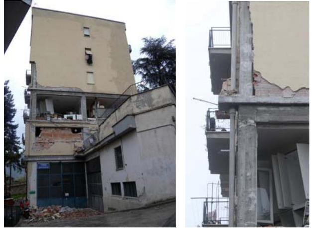
**Photo 16** Fall of masonry walls in a six-story building
