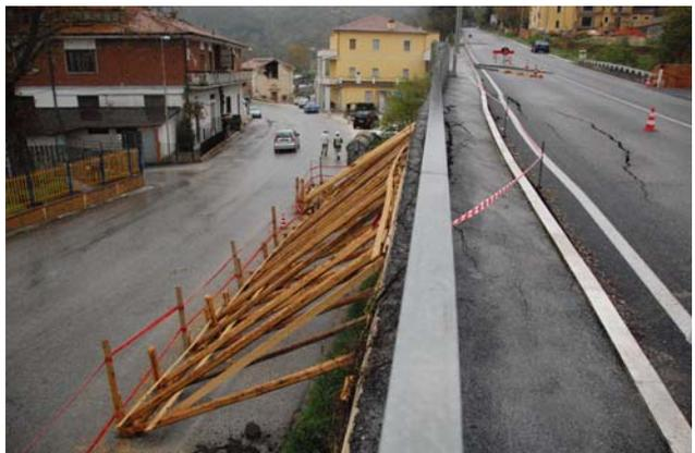
**Photo 34** Subsidence of a road embankment at the
