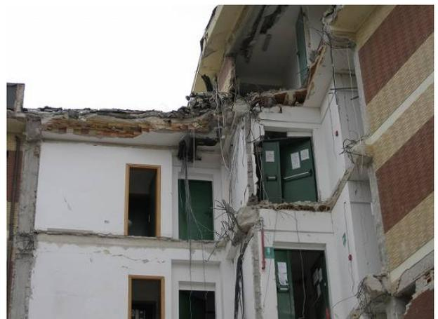
**Photo 9** Collapsed dormitory and two extended buildings
