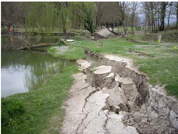
**Photo 2** Separated blocks due to lateral spreading
