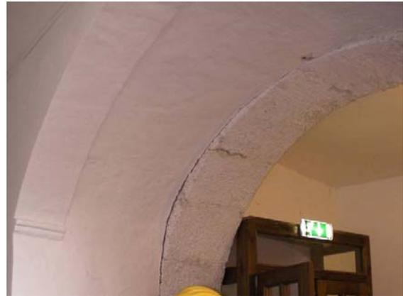
**Photo 24** Cracks and residual drift of an arch
