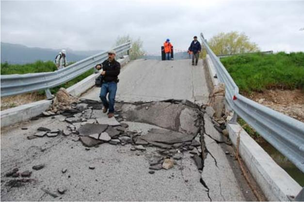
**Photo 29** Pile-bent piers which punching Village
