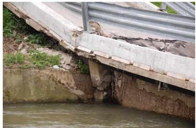
**Photo 28** Damage of pile-bent pier
