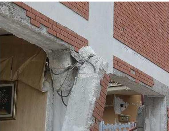
**Photo 19** Shear failure of a column at the top
