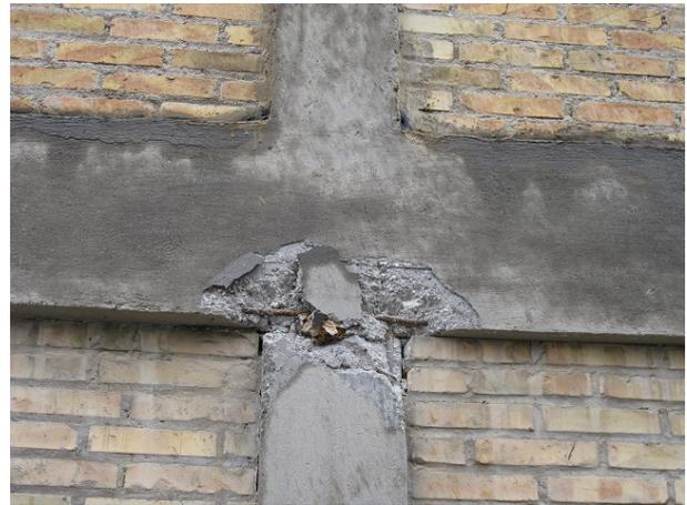
**Photo 18** Corrosion of longitudinal bars in a beam
