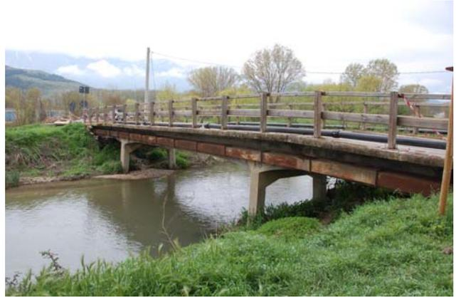
**Photo 30** A 20 m long bridge near Onna the deck sheared the deck slab
