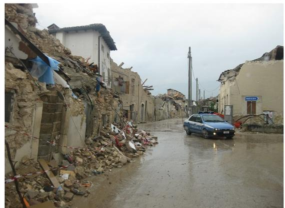
**Photo 26** Collapse of unreinforced masonry buildings in Onna village
