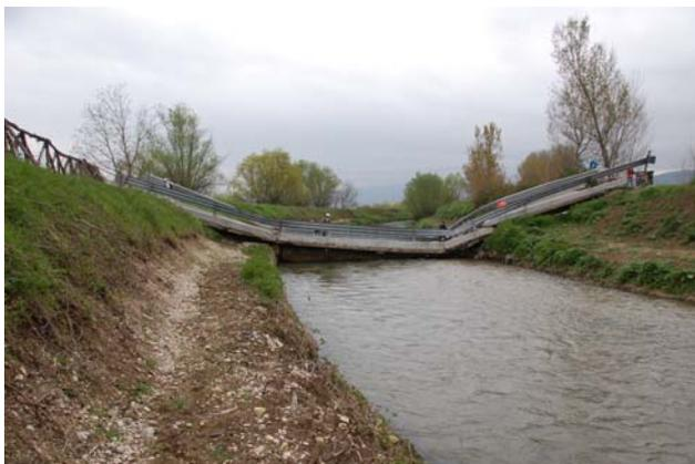
**Photo 27** Collapse of a three span continuous bridge near Fossa Station
