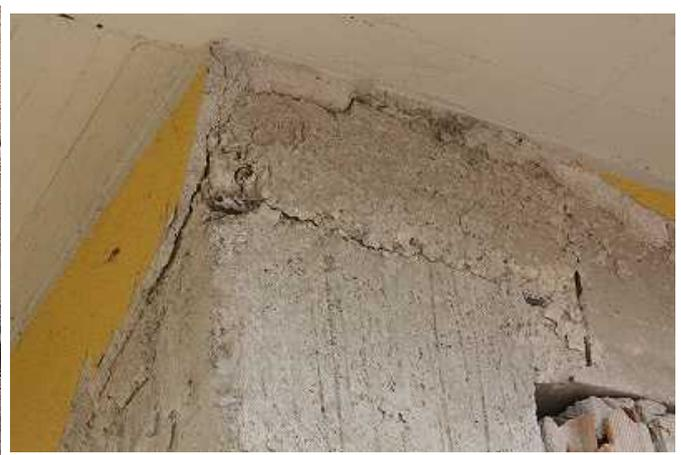
**Photo 20** Beam-column joint with construction joint at the top of the column
