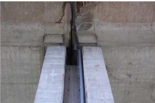
**Photo 33** Residual drift of two bridges in the intersection of Route SS17 and Route SR615
