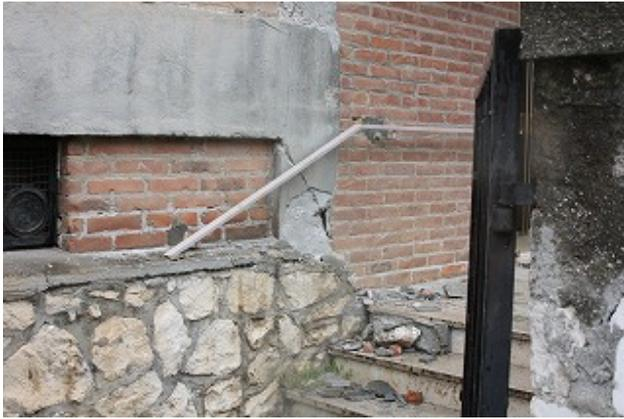
**Photo 21** Shear cracks of a short column in the first story
