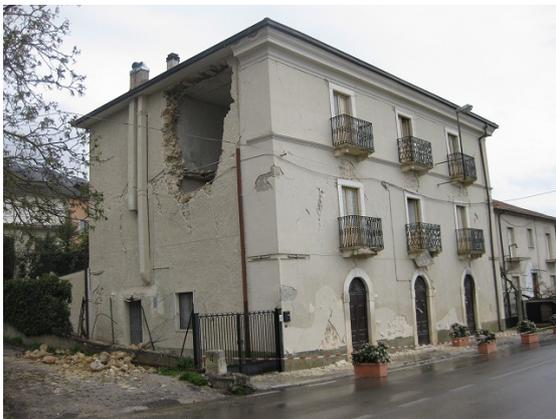
**Photo 25** Fall of wall bricks and finishing mortar of an unreinforced masonry building
