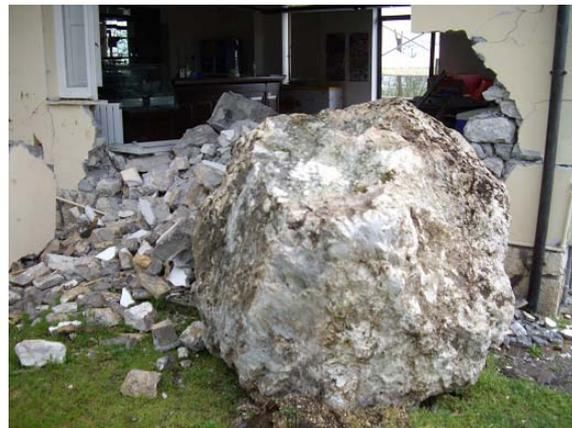
**Photo 4** A 12 ton fallen rock with 1.9m long, 1.6m wide and 1.5m tall
