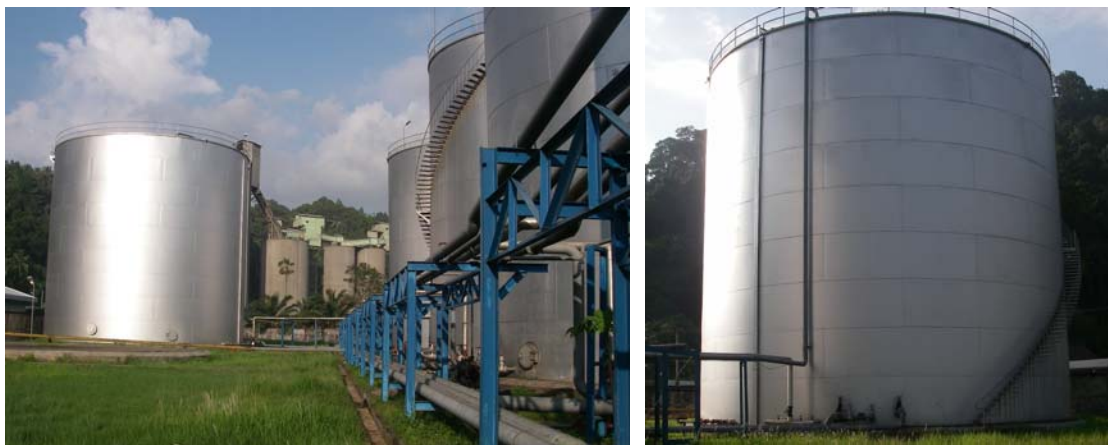
Fig.5.13 Tank yards in Teluk Bayur Port of Padang Ciity and Painan City
