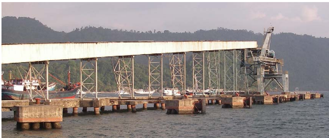
Fig.5.14 Slightly damaged Conveyor of loading facility at Teluk Bayur Port
