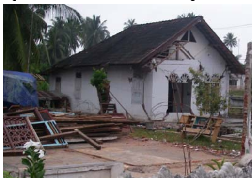
Fig.5.2 Collapsed or heavily damaged brick masonry houses
