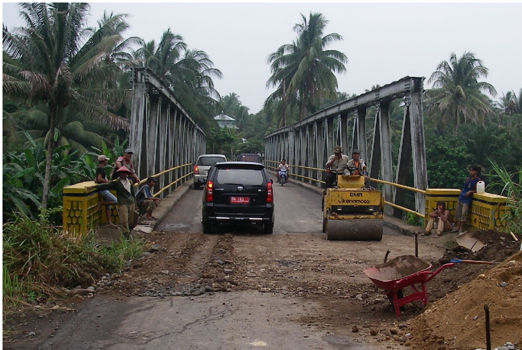
Fig.5.11 Damage to approach embankments of bridges
