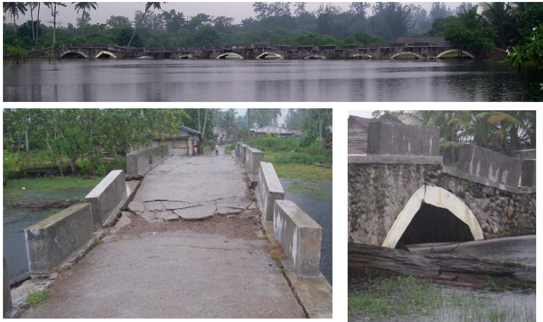
Fig.5.9 Damage to the arch bridge at Pasir Ganting due to ground liquefaction
