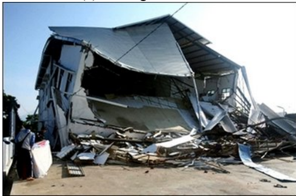
(c) Collapsed show room in Argamakmur
