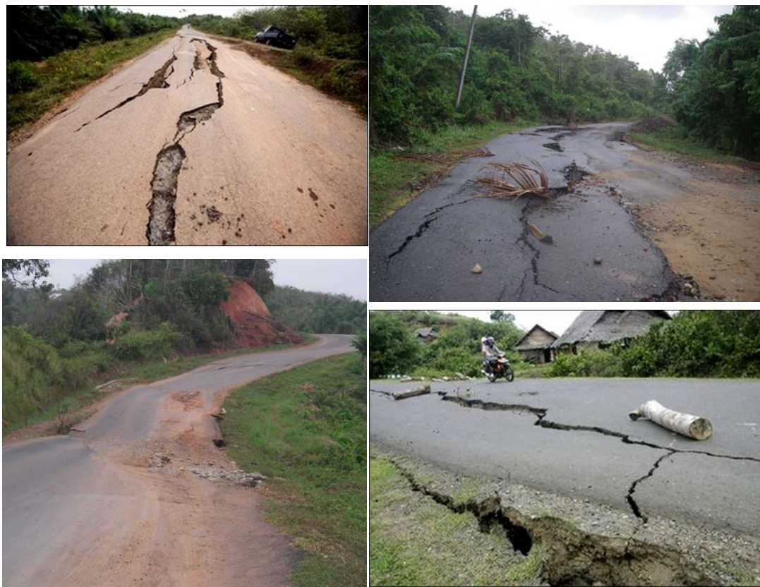
Fig.5.8 Some examples of failures of embankments of roadways
