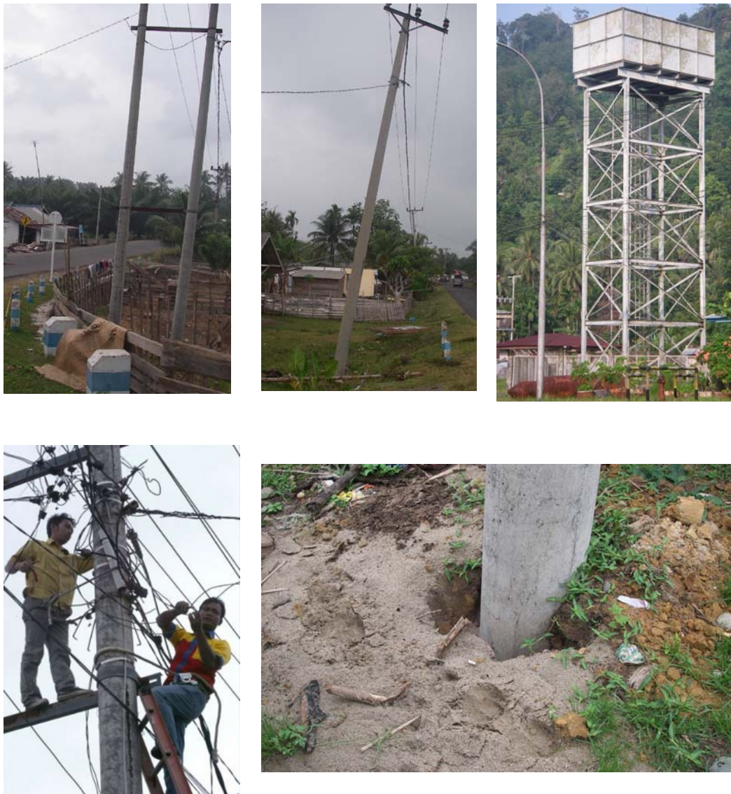
Fig.5.12 Views of some damage to utility poles and a non-damaged elevated water tank
