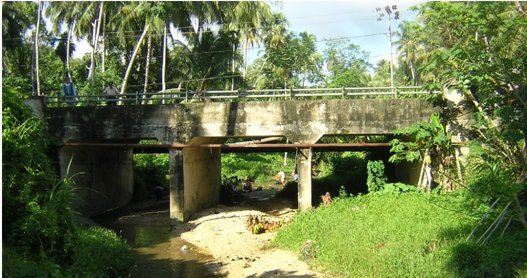
Figure 10.6 Non-damaged RC box culvert
