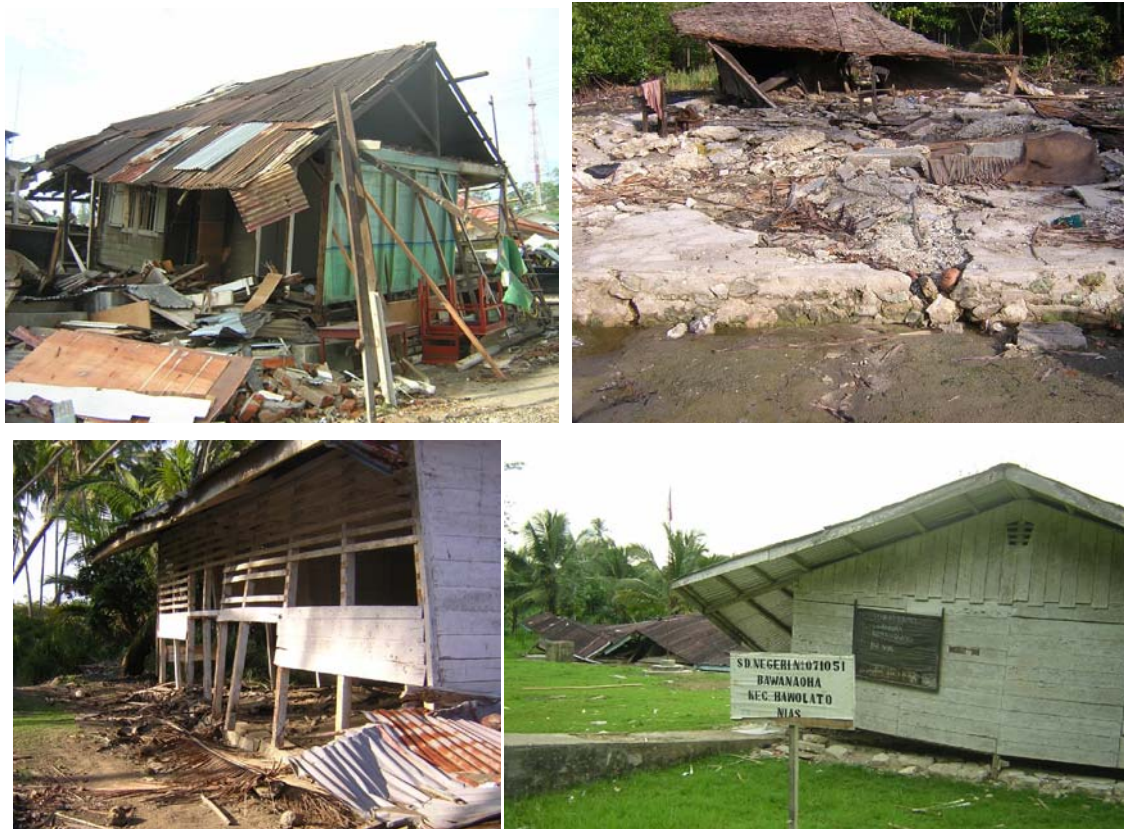
Figure 9.11 Damage to wooden houses and schools
