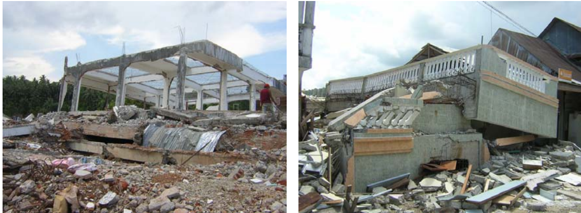
Figure 9.10 Heavy damage or collapse of RC buildings in Telukdalam
