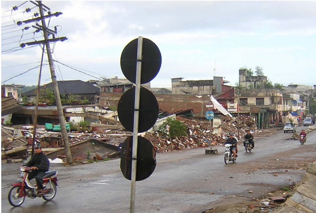
Figure 9.8 Collapsed buildings at a corner of street in Gunung Sitoli
