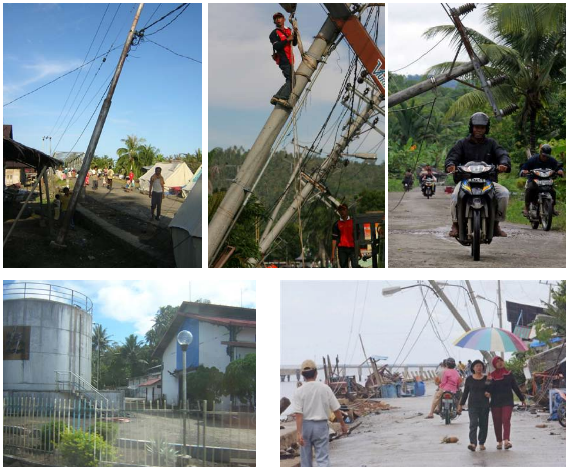
Figure 14.1 Effects of the earthquake on electricity system
