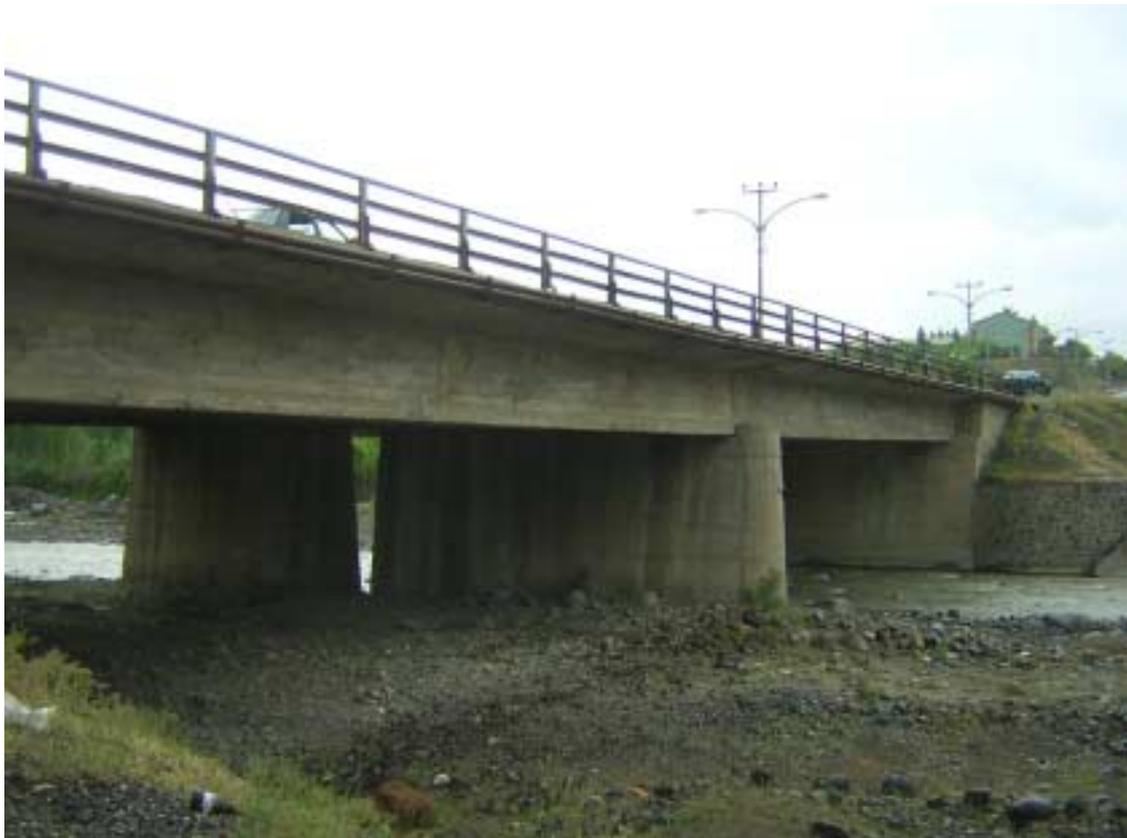
Figure 10.5: Slightly-damaged RC three-span highway bridge on Çapakçur brook
