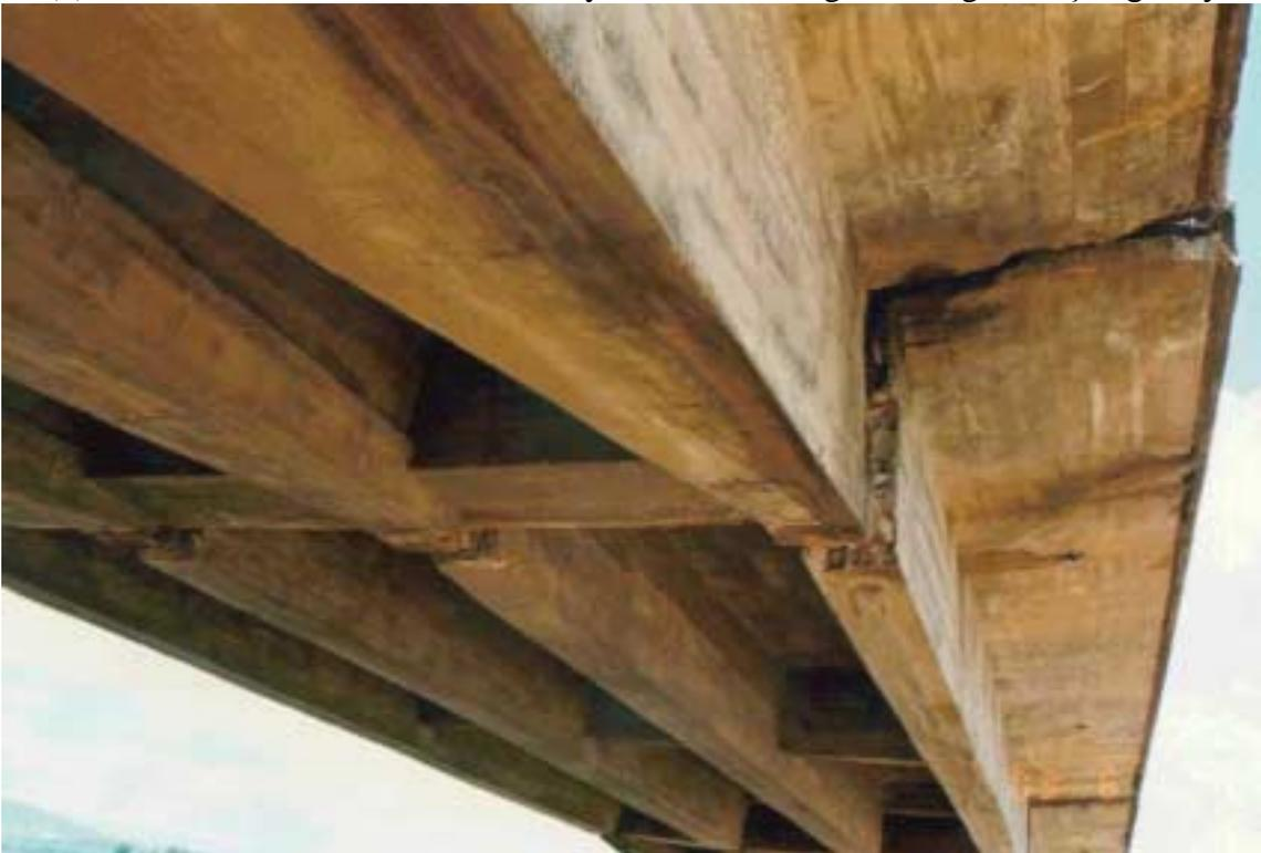
(c) Girder off-set of Gerber-type section of the bridge
