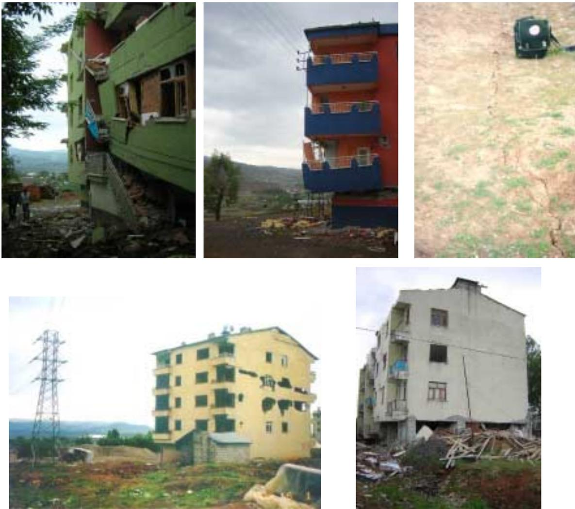
Figure 8.5: Collapsed or heavily damaged RC buildings nearby slope crest in Saray District
