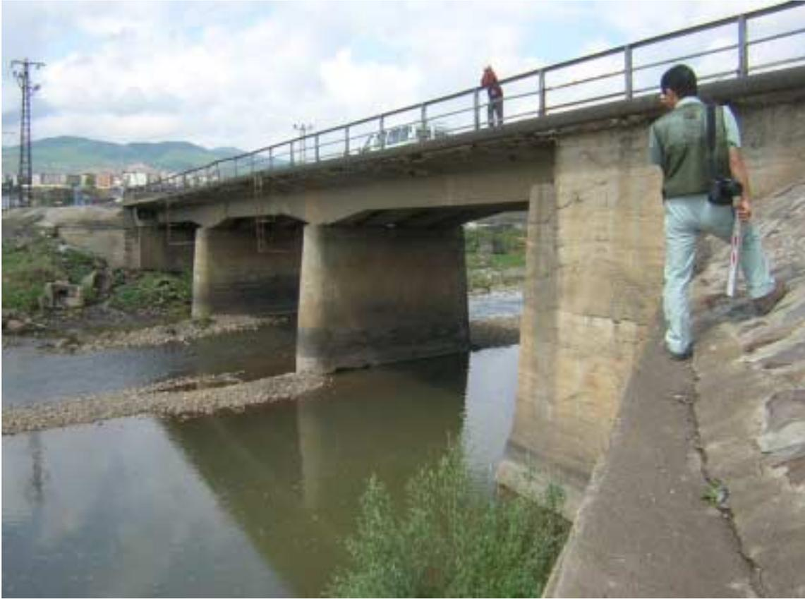
Figure 10.4: Non-damaged RC three-span highway bridge on Gayıt brook
