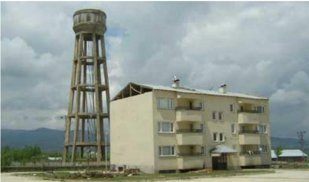
Figure 13.7: The non-damaged water tower in Çeltiksuyu village where two school buildings with 3-4 floors were all collapsed
