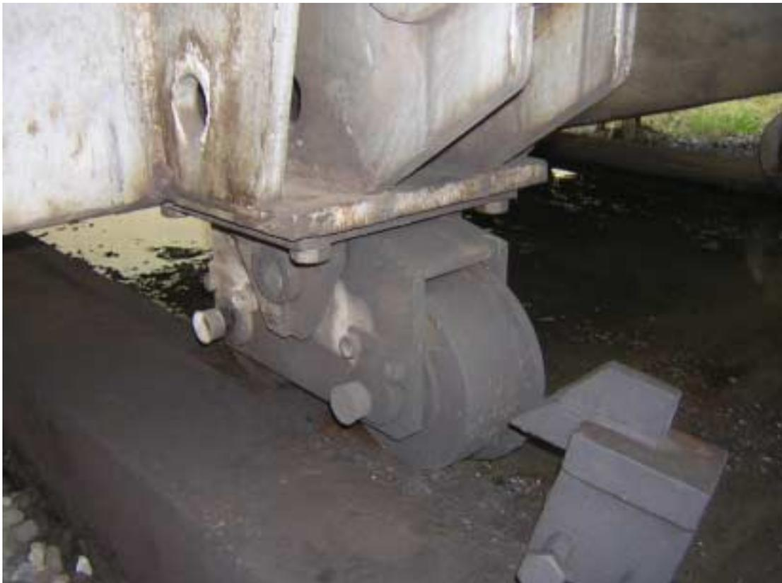
Figure 9.4 Slightly displaced transformer
