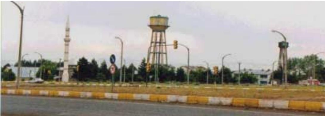
Figure 13.6 Non-damaged water towers in Bingöl City nearby the strong-motion station
