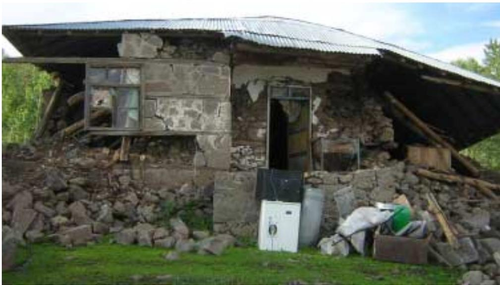
(b) The collapse of a stone masonry house (ground is very soft)
