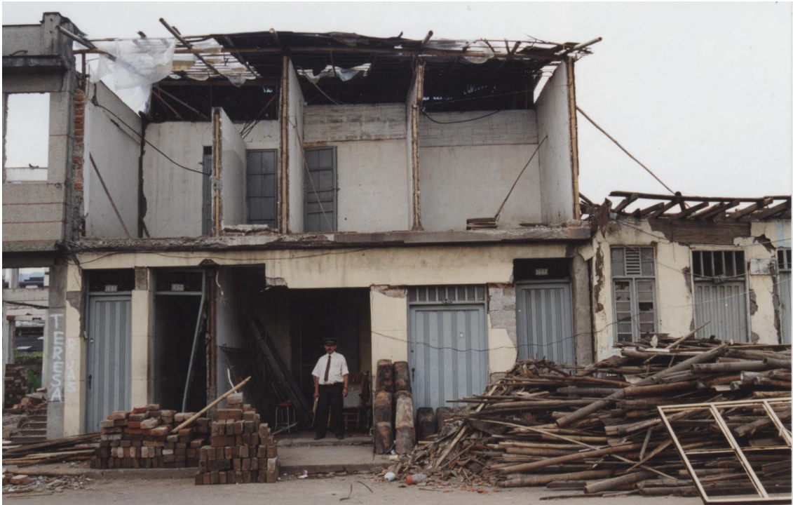
Photo 5 Damage to unreinforced masonry wall (Armenia)
