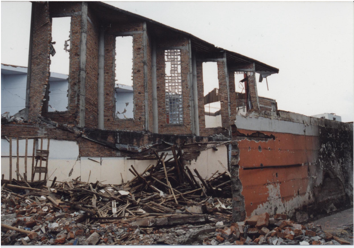
Photo 7 Collapse of two story houses (Armenia)
