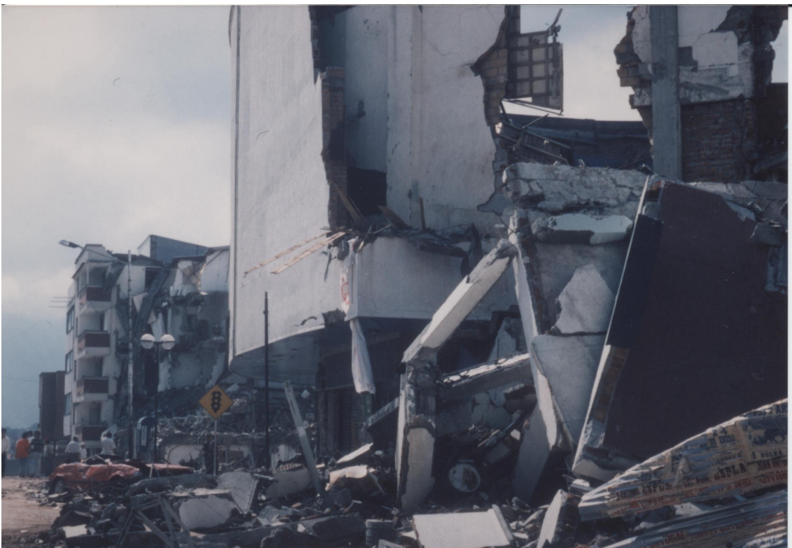
Photo 15 Damage to first story of building
