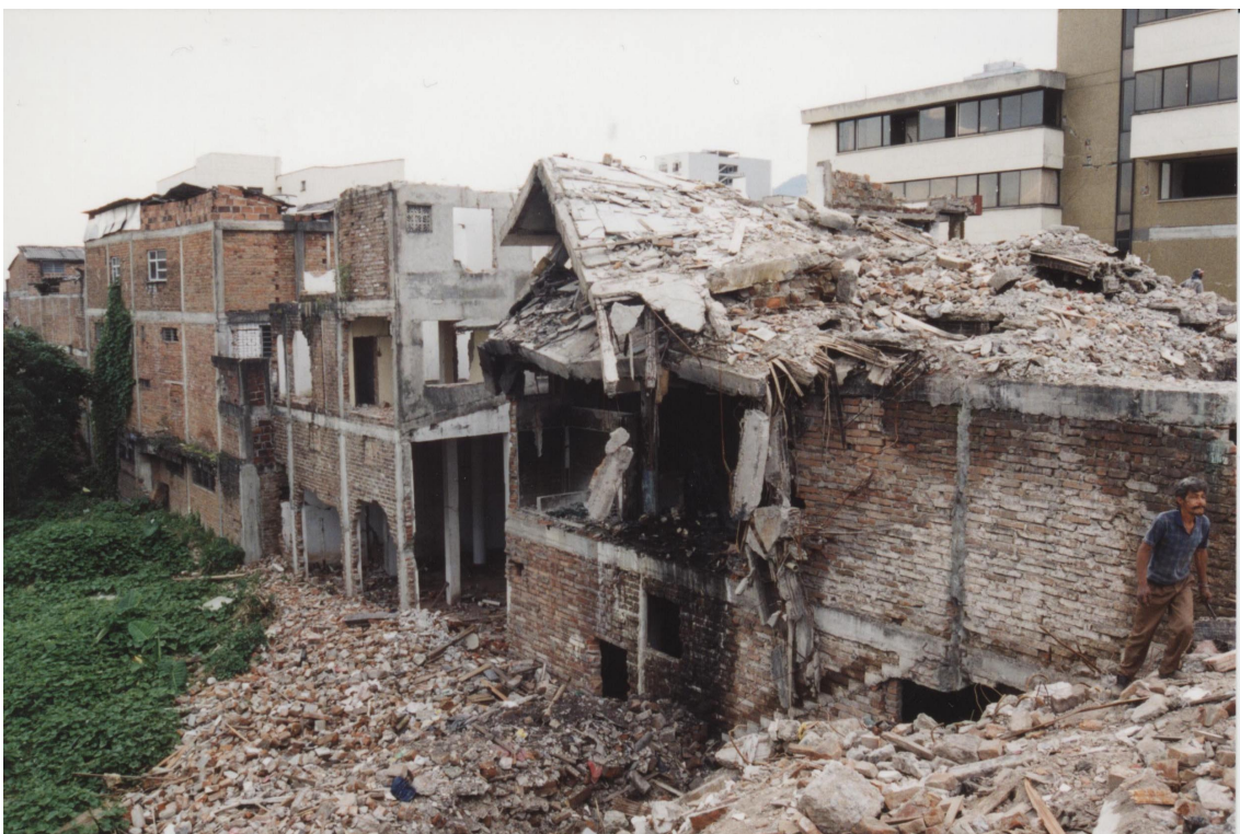
Photo 8 Collapse of masonry wall structures (Armenia)
