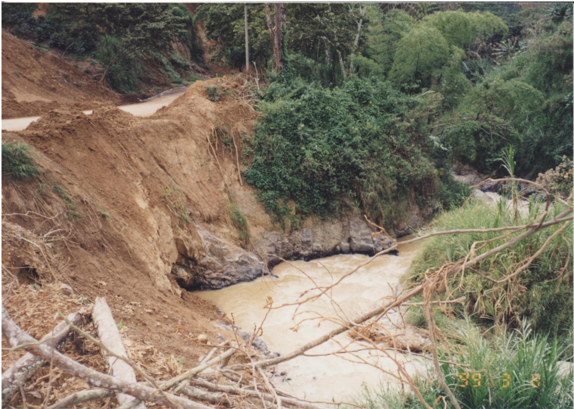
Photo 17 Slope failure along the road between Calarca and Barcelona
