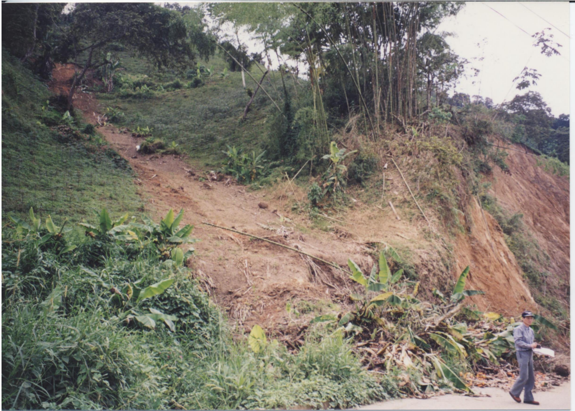
Photo 18 Slope failure along the road between Calarca and Barcelona
