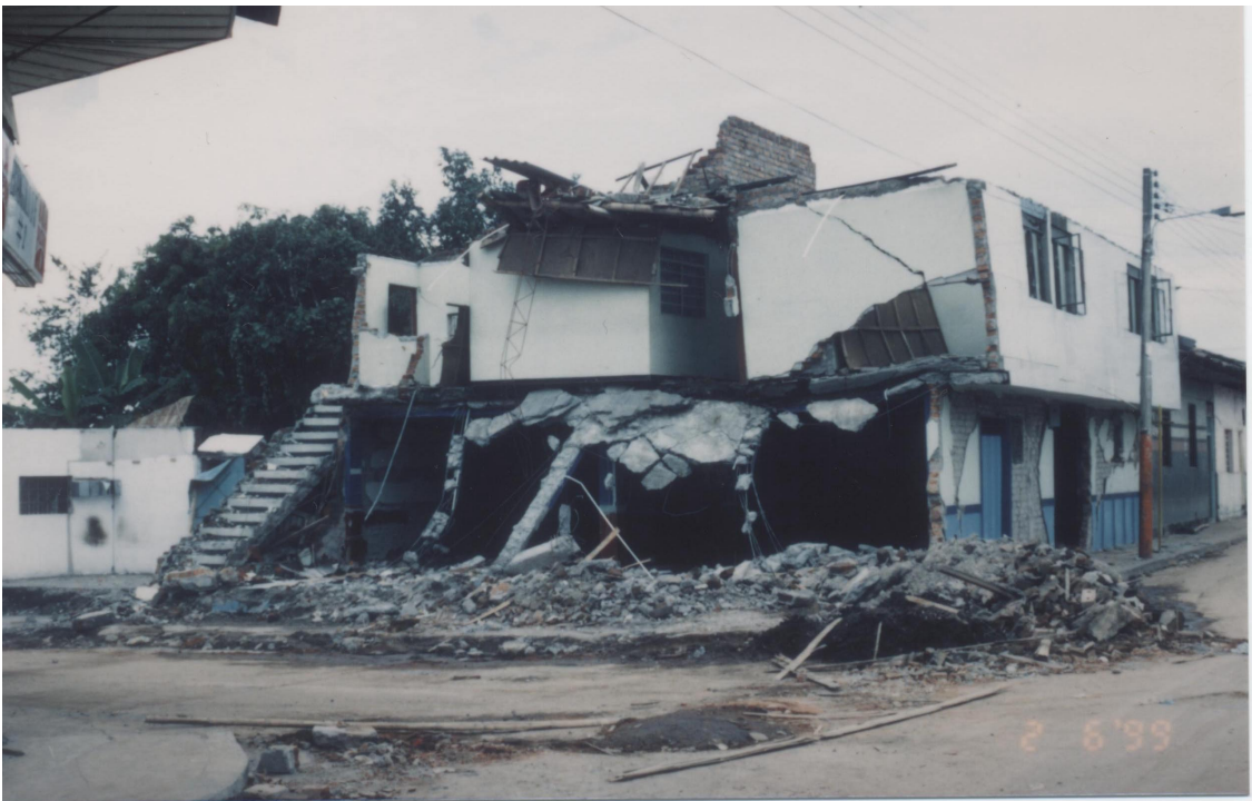
Photo 2 Collapse of two story houses (Courtesy: by E.Rodriguez Grandos) (Armenia)
