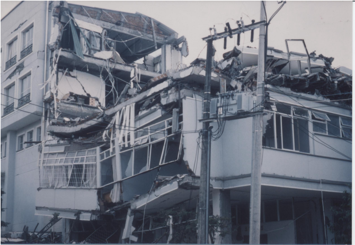
Photo 14 Damage to irregular building (Armenia)
