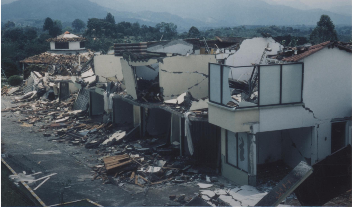
Photo 1 Collapse of two story houses (Courtesy: by E.Rodriguez Grandos) (Armenia)
