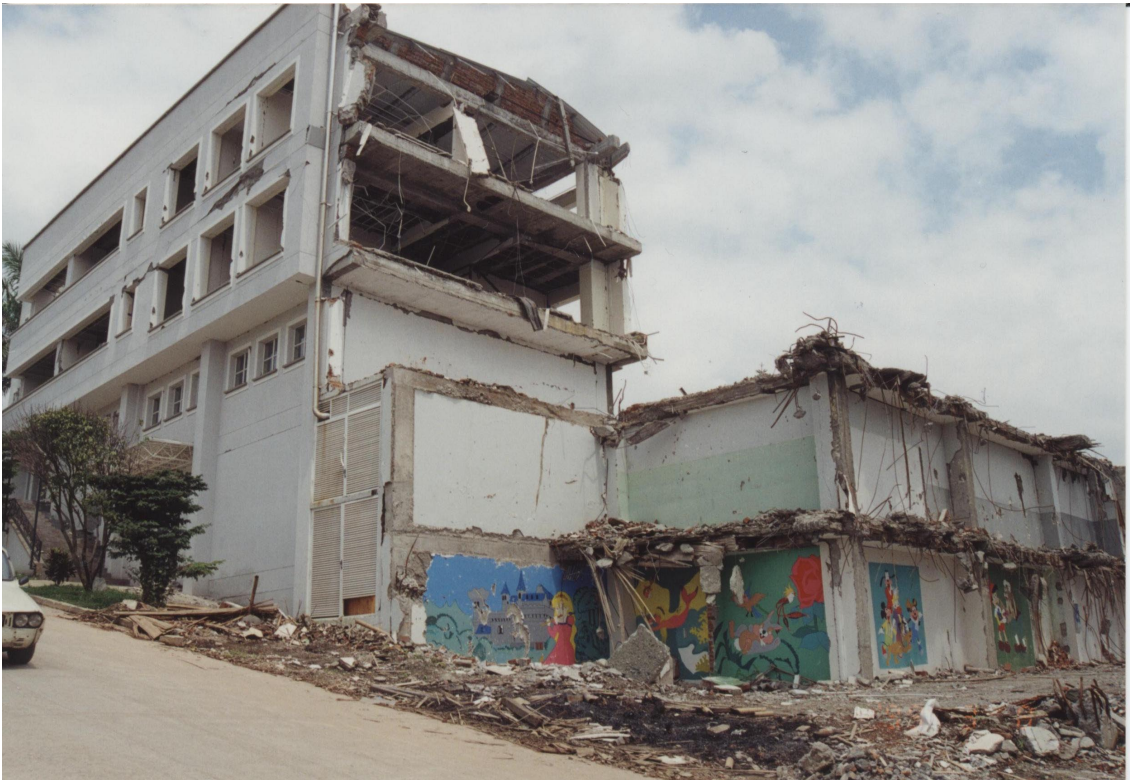
Photo 13 Damage to building on hillside (Armenia)
