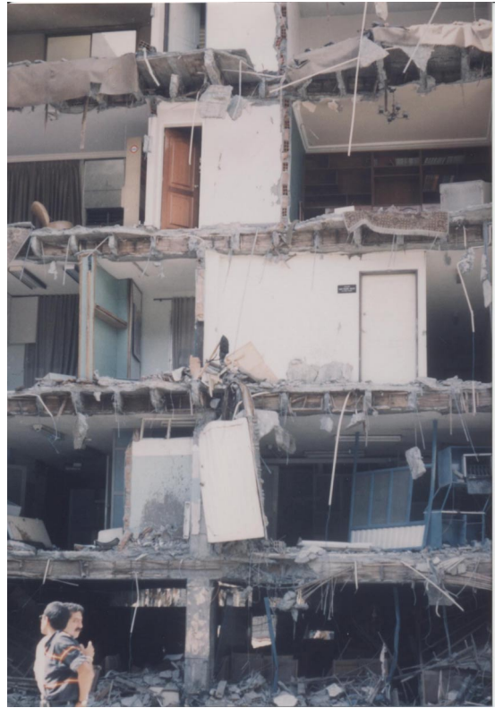
Photo 12 Fall of masonry walls (Armenia)
