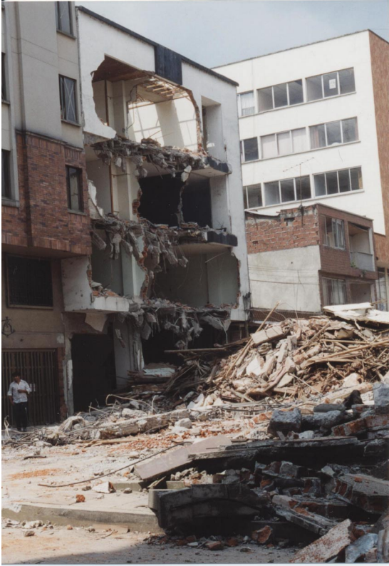
Photo 11 Fall of masonry walls (Armenia)
