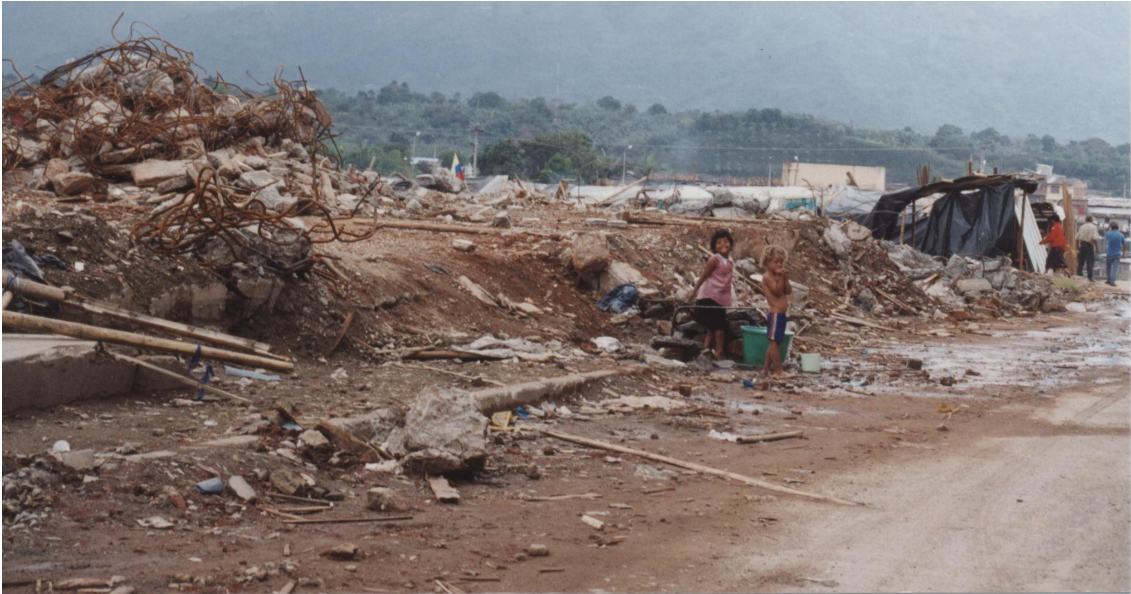
Photo 9 Severe damaged area in Armenia City
