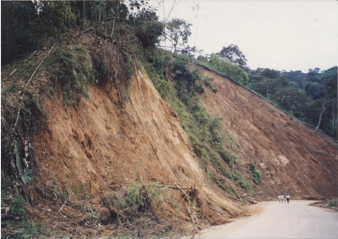
Photo 16 Slope failure along the road between Calarca and Barcelona
