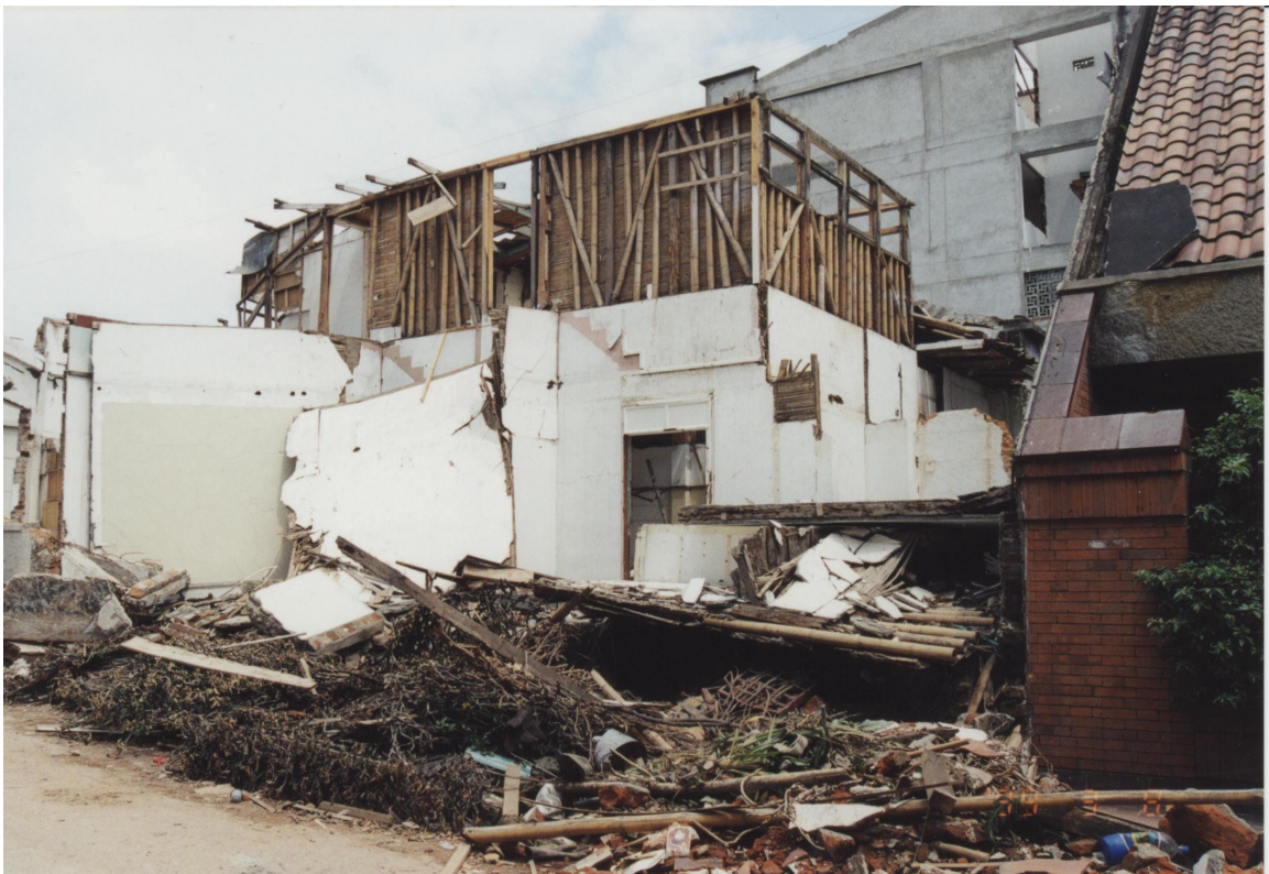
Photo 4 Collapse of two story houses with bamboo frame plastered wall (Armenia)
