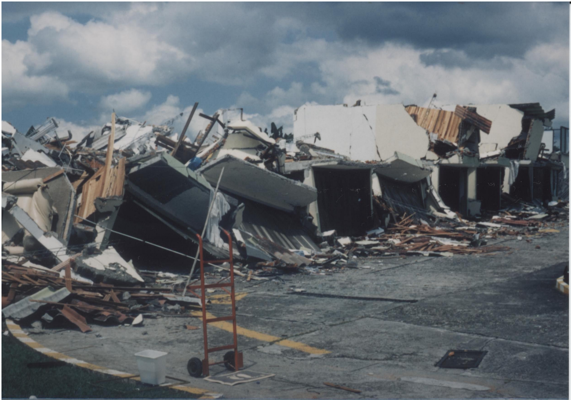
Photo 3 Collapse of two story houses (Courtesy: by E.Rodriguez Grandos) (Armenia)
