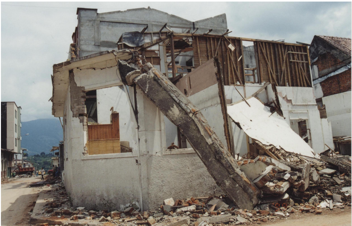
Photo 6 Collapse of two story houses (Armenia)
