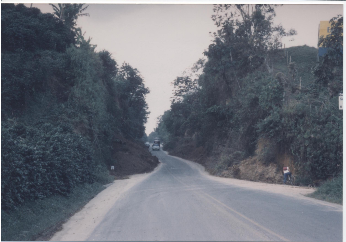
Photo 19 Slope failure at Armenia City
