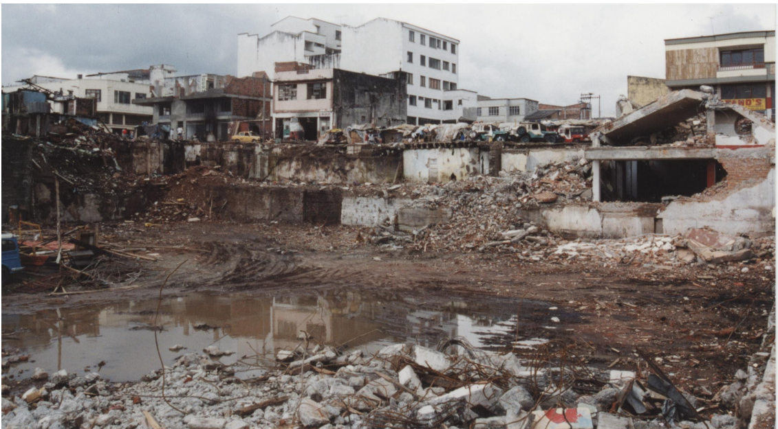
Photo 10 Severe damaged area in Armenia City
