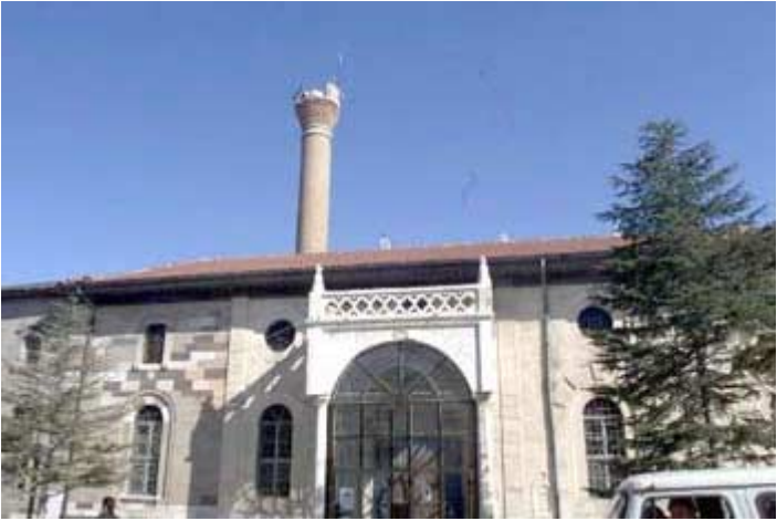
Figure 24 Damage to mosques and collapses of their minarets (pictures by Milliyet)
