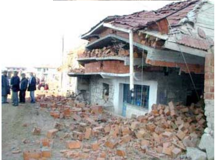
Figure 22 Damage and collapses of wooden and masonry structures (pictures by Milliyet)
