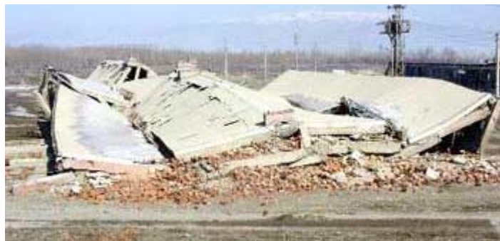
Figure 23 Damage and collapses of reinforced concrete structures (pictures by Milliyet)
