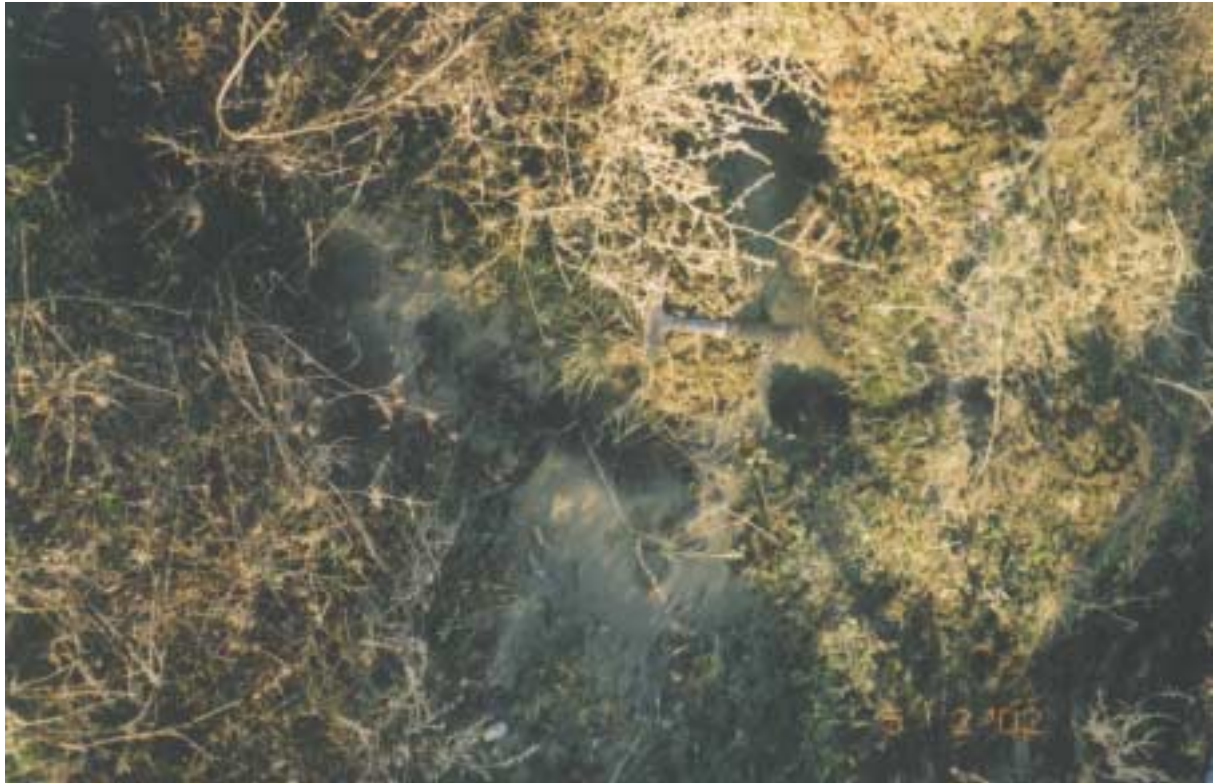
Figure 26 Ground liquefaction (picture by H. Kumsar of Pamukkale University)
