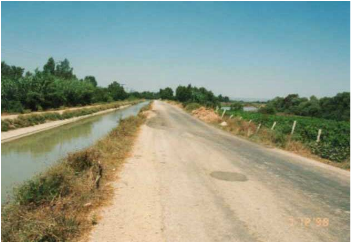
Figure 9.9: Embankment failure near Abdioglu village
