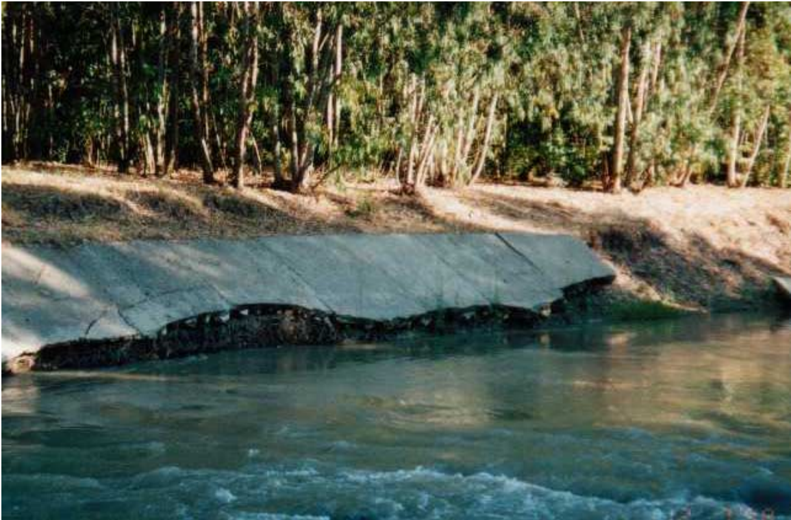
Figure 9.5: Failure at the southern bank of a stream near Sirkeli village (SE of Ceyhan town)
