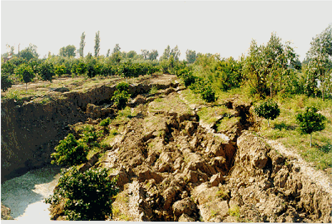
Figure 9.3: Soil slope failure along Ceyhan River near Abdioglu village
